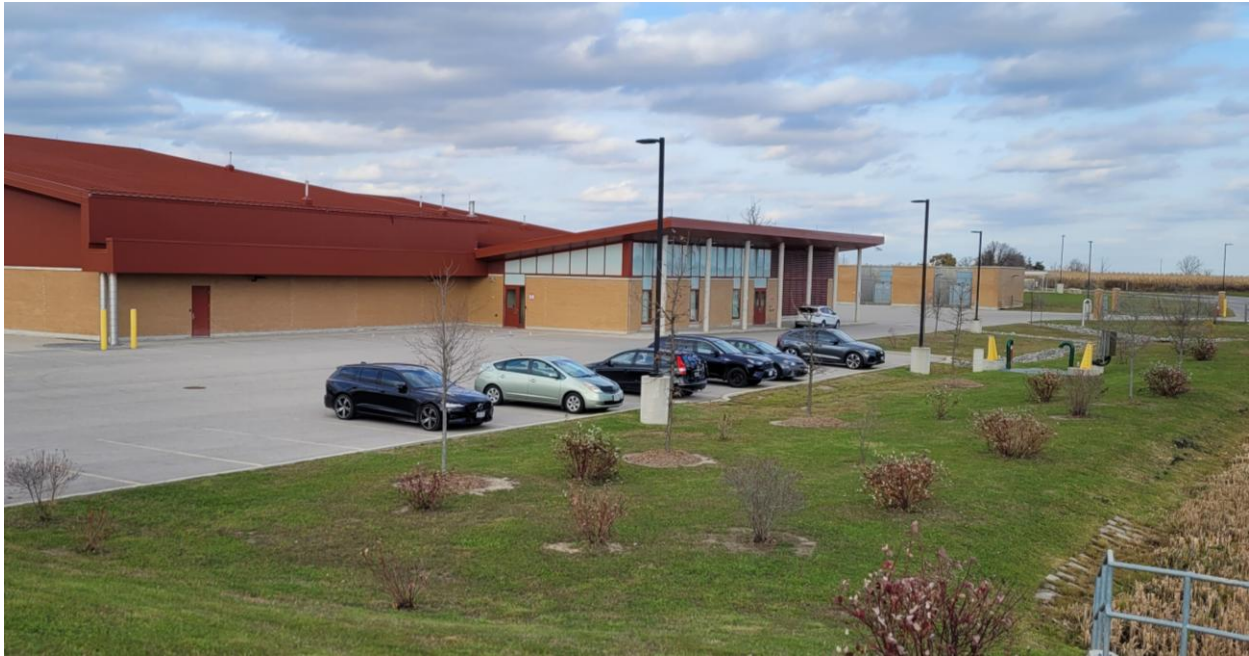
Figure 4-9: Alloa Reservoir and Pumping Station Facility
