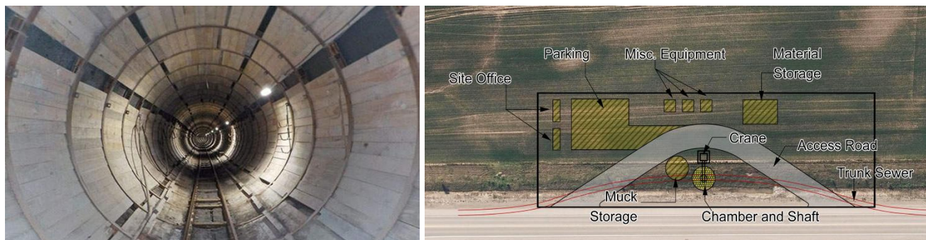
Figure 6-7: Inside a Tunnel Shaft (left) and Typical Shaft Compound Layout (right)
