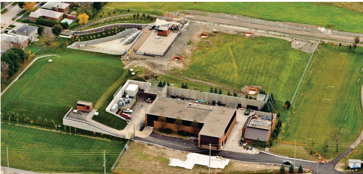
Figure 7. Herridge Reservoir and Pumping Station
