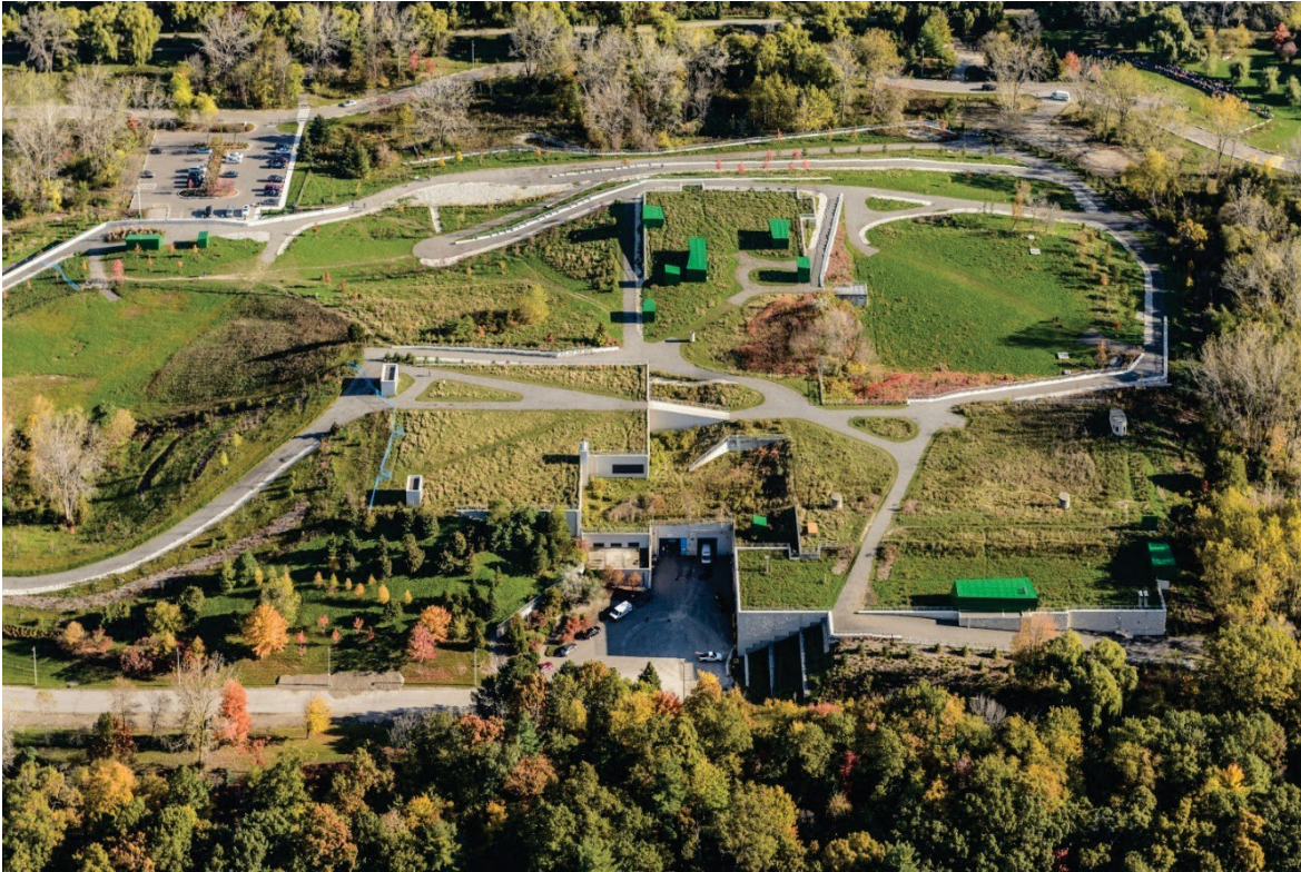
Figure 6. Lorne Park Water Treatment Plant
