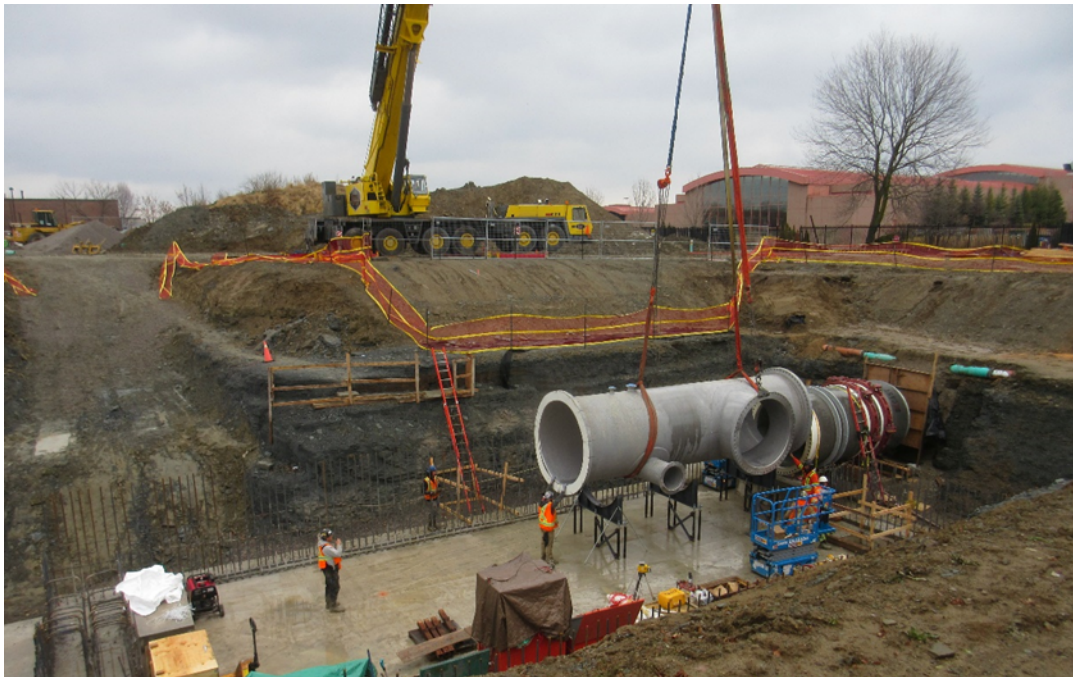
Figure 2. Arthur P. Kennedy WTP yard piping upgrade project
