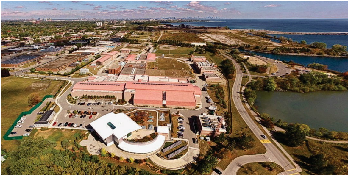
Figure 5. Arthur P. Kennedy Water Treatment Plant
