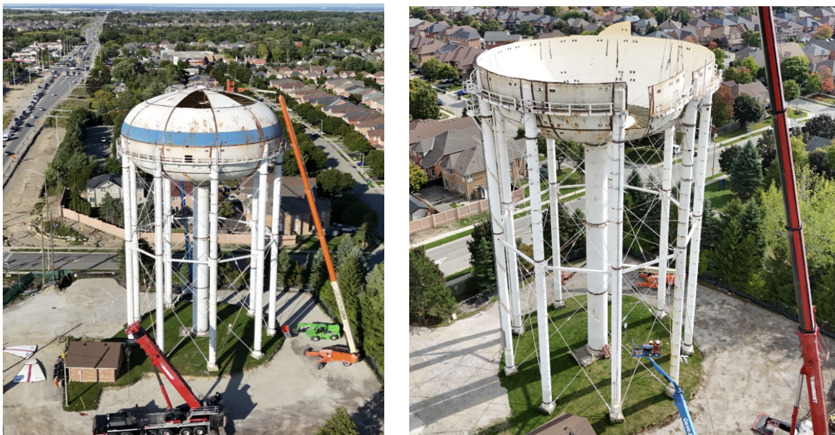
Figure 4. Snelgrove Elevated Tank Removal Project
