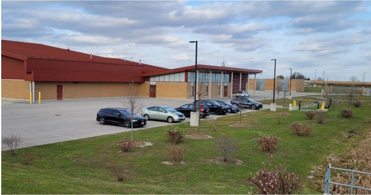
Figure 4-9: Alloa Reservoir and Pumping Station Facility
