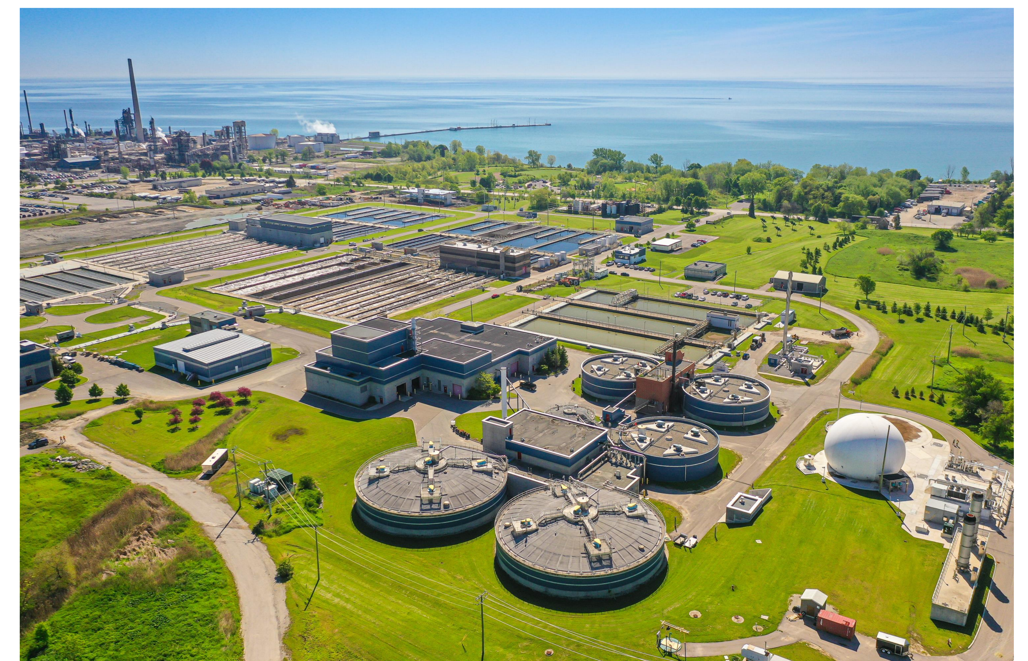
Clarkson Wastewater Treatment Facility, Peel Region
