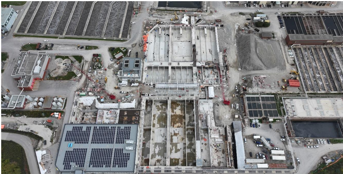
Figure 6. Aerial view of G.E. Booth WRRF under construction
