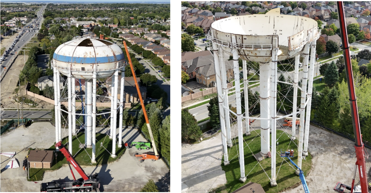
Figure 4. Snelgrove Elevated Tank Removal Project
