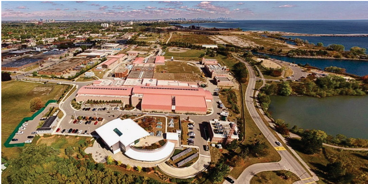
Figure 5. Arthur P. Kennedy Water Treatment Plant
