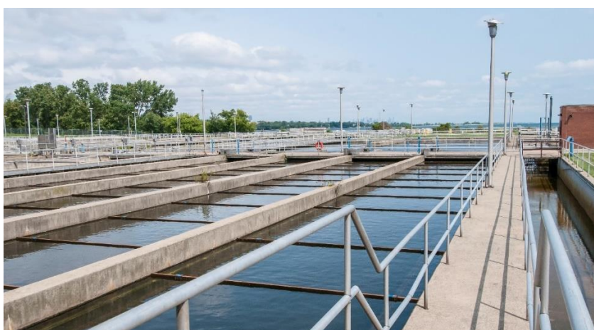
Figure 10. Row of outdoor wastewater secondary clarifier tanks at a Peel Region water resource recovery facility
