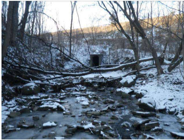
View facing upstream at the Bovaird Drive culvert outlet. It is evident that the culvert is undersized in relation to the existing watercourse. Scour along bed and banks of channel have resulted.
