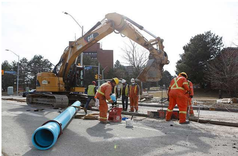
Region of Peel Watermain Construction
