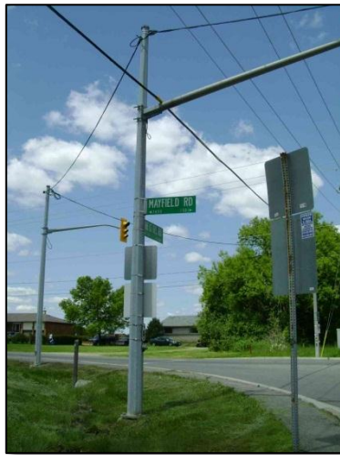
Mayfield Road Intersection
