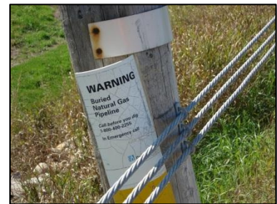
Underground Gas Line Marker at Mayfield Road
