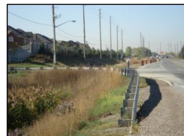
Existing Hydro One Brampton overhead hydro line.
