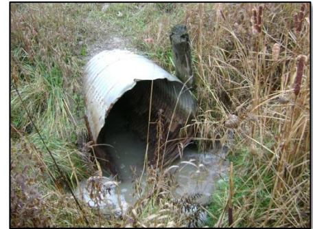
Mayfield Road CSP Culvert
