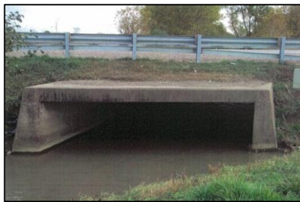
Mayfield Road Open Bottom Concrete Culvert
