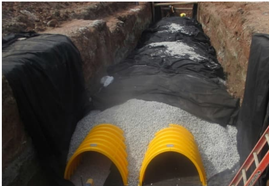
Figure 6.8 – SWM Alternative 7 Superpipe Storage
