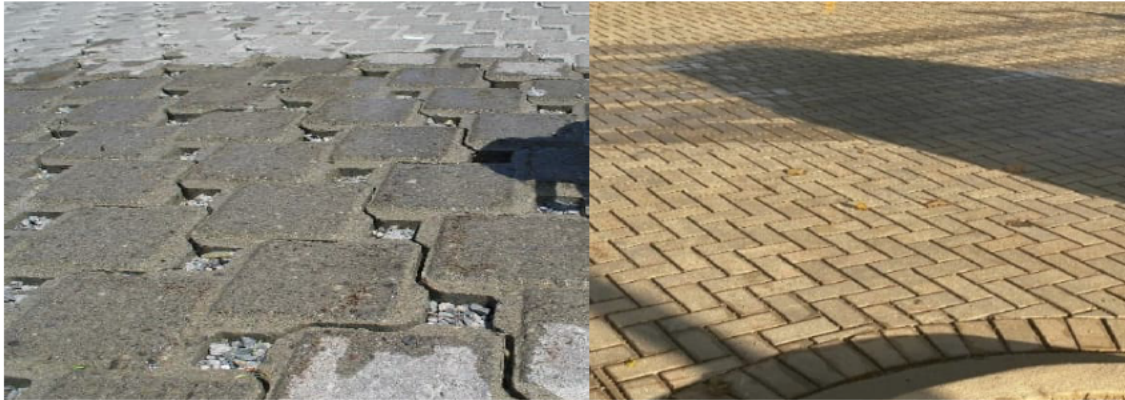
Figure 6.6 – SWM Alternative 5 Permeable Pavement
