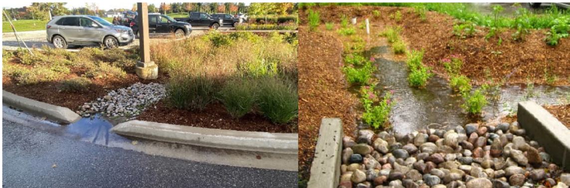
Figure 6.5 – SWM Alternative 4 Bioretention Facilities
