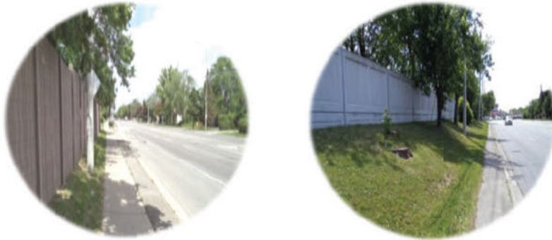
Existing Noise Walls
