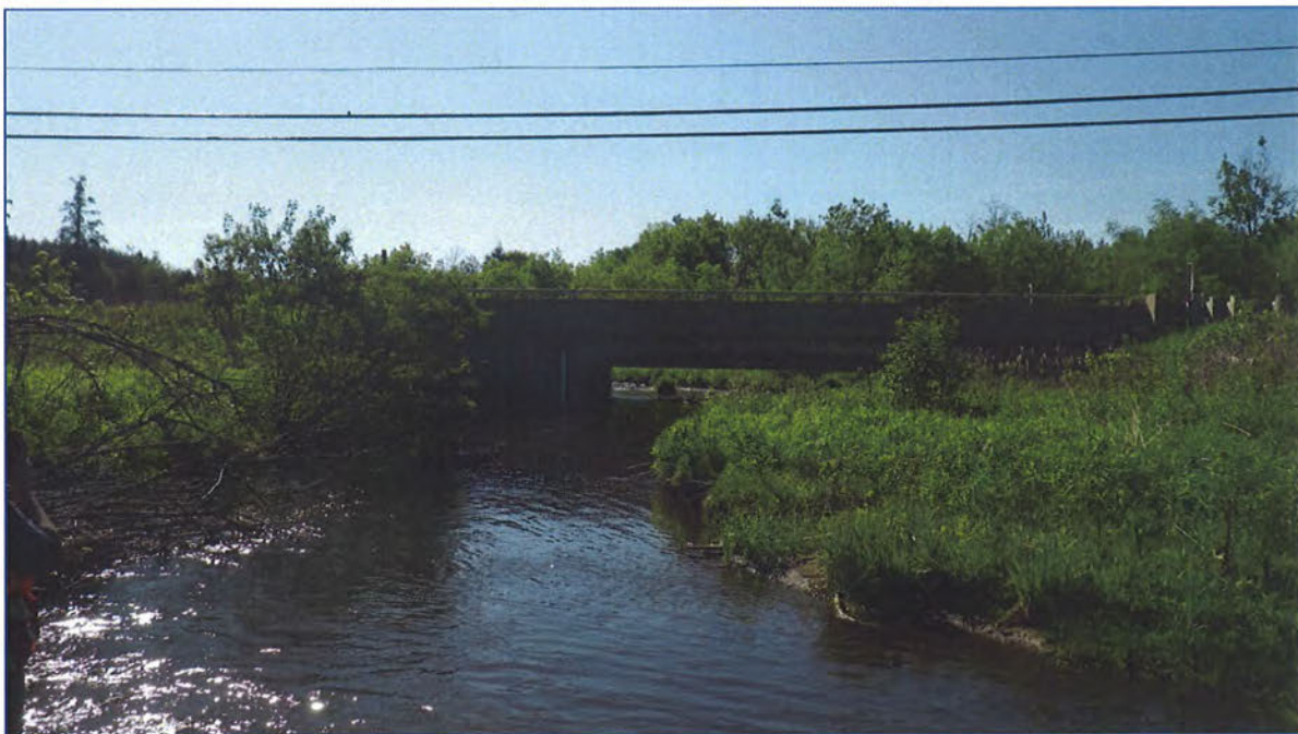
Photo 6: Shaws Creek - View downstream of bridge at Highway 136; note the leaning /failed shrubs along left bank due to erosion and the misalignment of the channel with the bridge opening.
