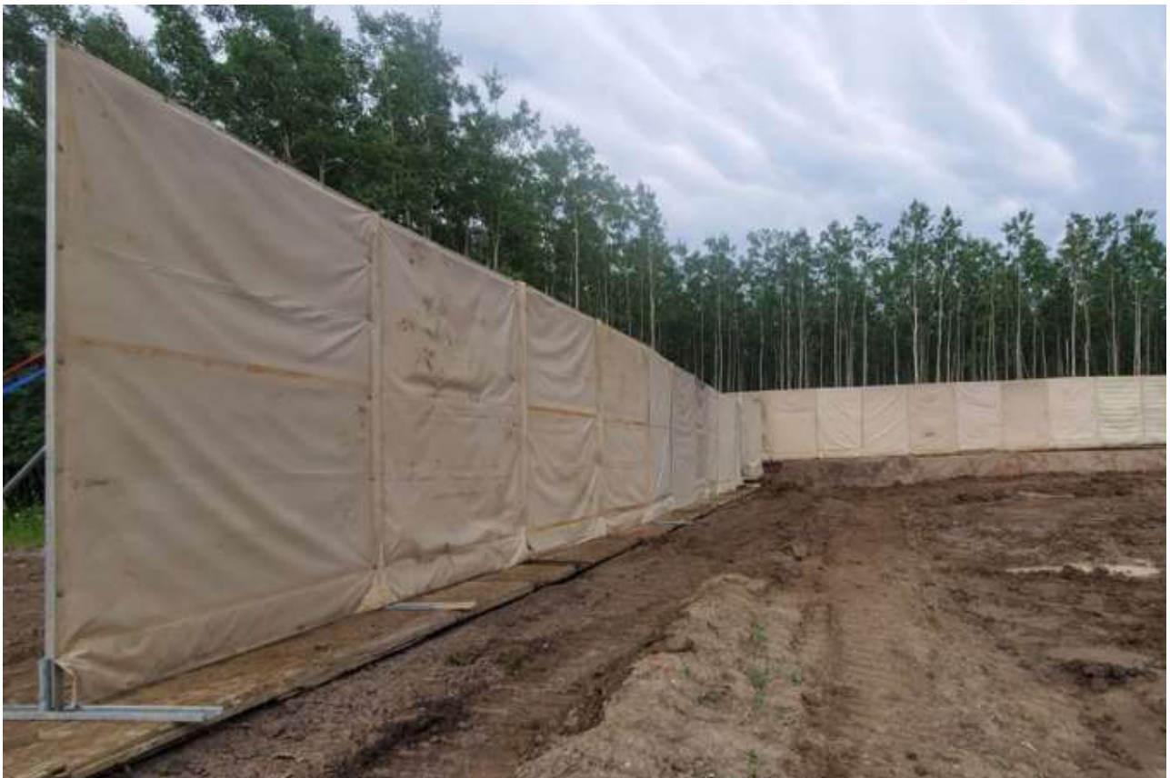
Figure 2: Example of a Temporary Noise Curtain
