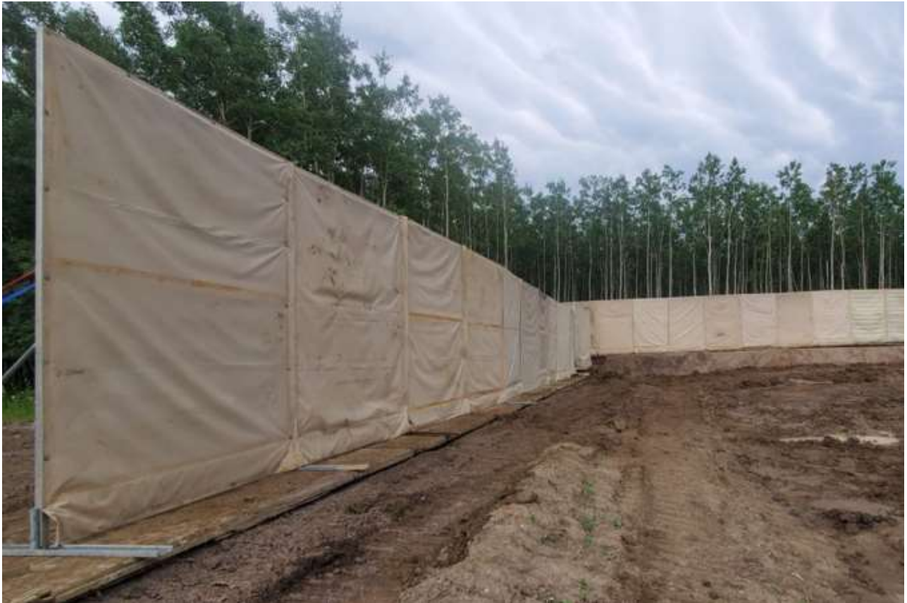
Figure 2: Example of a Temporary Noise Curtain
