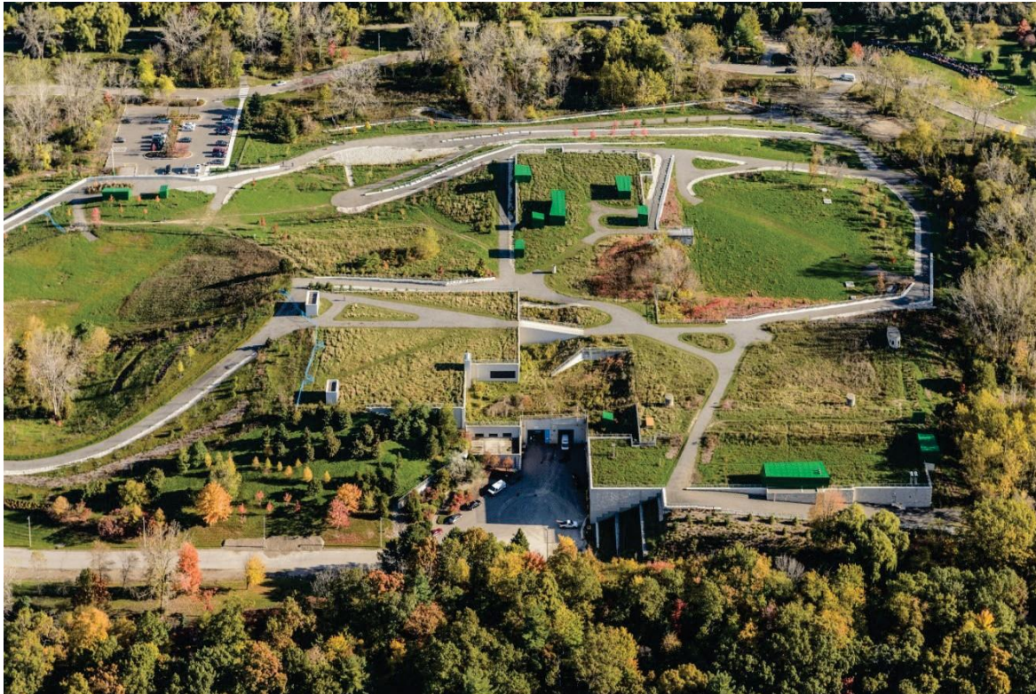
Figure 6. Lorne Park Water Treatment Plant
