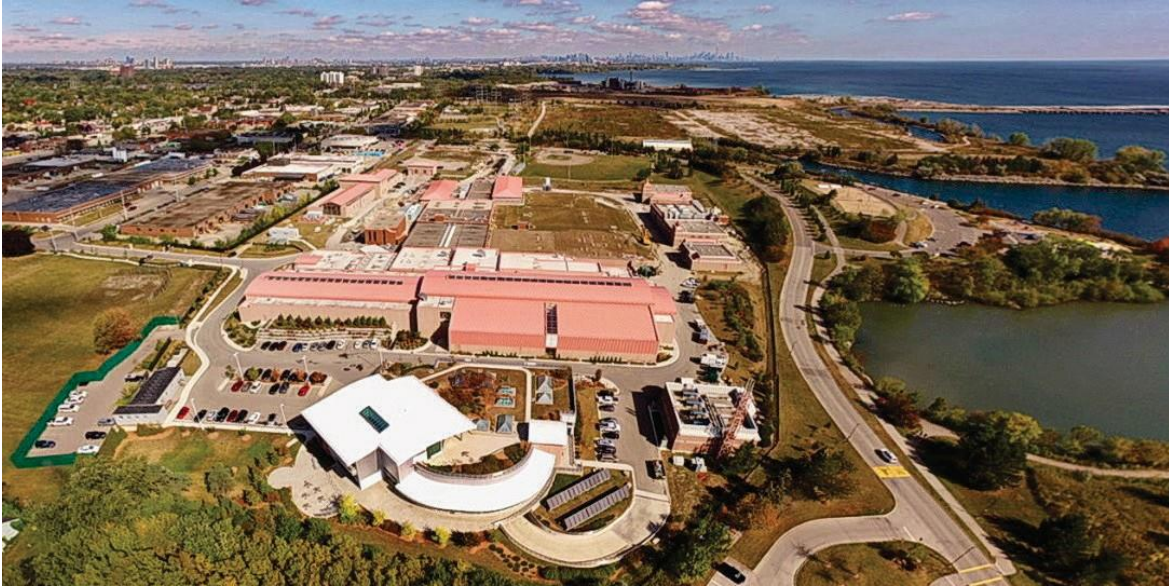
Figure 5. Arthur P. Kennedy Water Treatment Plant
