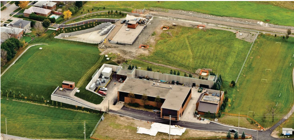
Figure 8. Herridge Reservoir and Pumping Station
