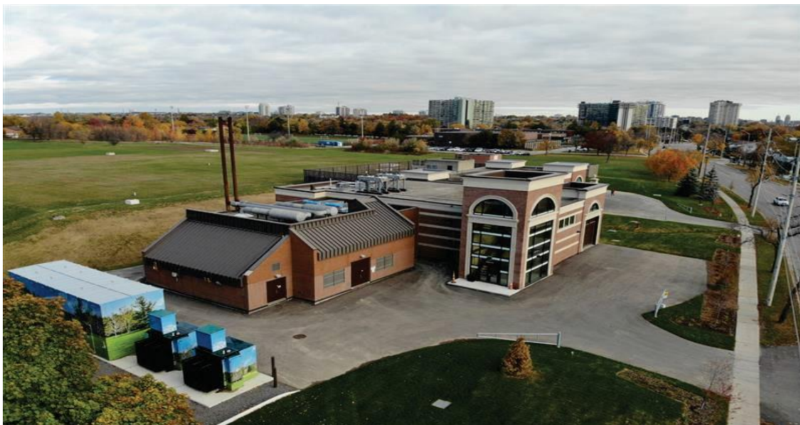
Figure 4. Silverthorn Pumping Station electrical building upgrade
