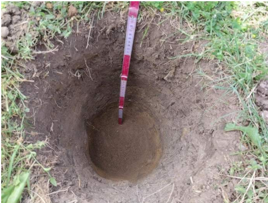
Image 6: Example of disturbed soil profile with various layers of fill overlying subsoil
