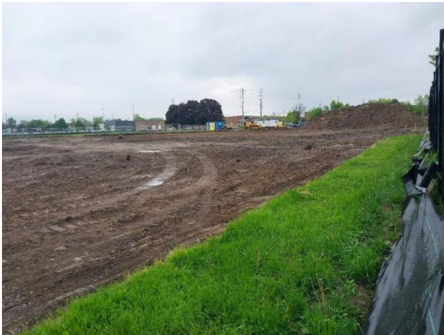
Image 8: Construction of Yard Piping Upgrades project underway; further work required
