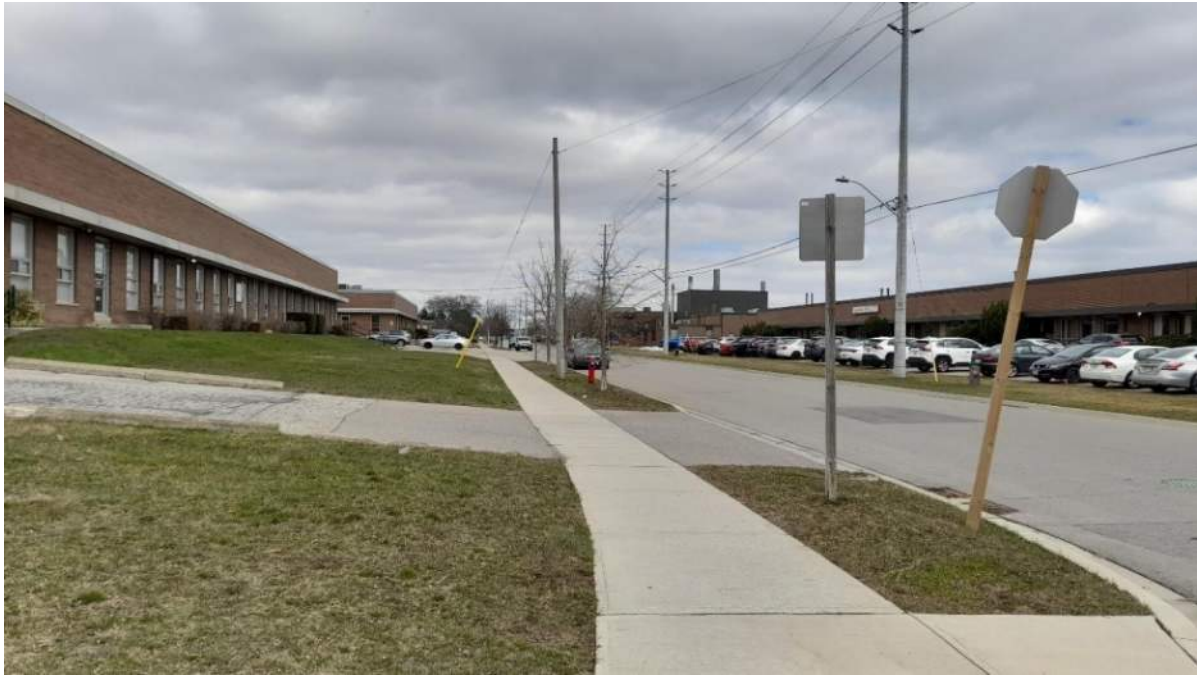
Plate 6: Industrial and commercial properties along Rangeview Road, looking east from East Avenue (A.S.I., 2024).
