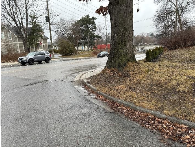
Motor Vehicle Facilities: Sightlines facing north are partially obstructed by large tree and grade change at the underpass, requiring drivers to encroach the pedestrian right-of-way for a clear sightline. Photo Location: On westbound approach, looking north
