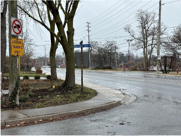
Motor Vehicle Facilities: Sightlines facing south are partially obstructed by trees and signage, requiring drivers to encroach the pedestrian right-of-way for a clear sightline. Photo Location: On westbound approach, looking south
