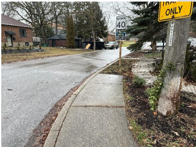
Southeast sidewalk abruptly ends
