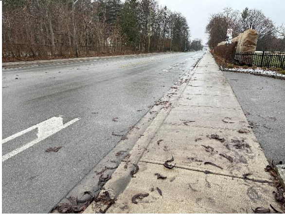
Bicycle lane markings are discontinued through the intersection Photo Location: Dixie Road at Toronto Golf Club Access, south side of the intersection, looking north
