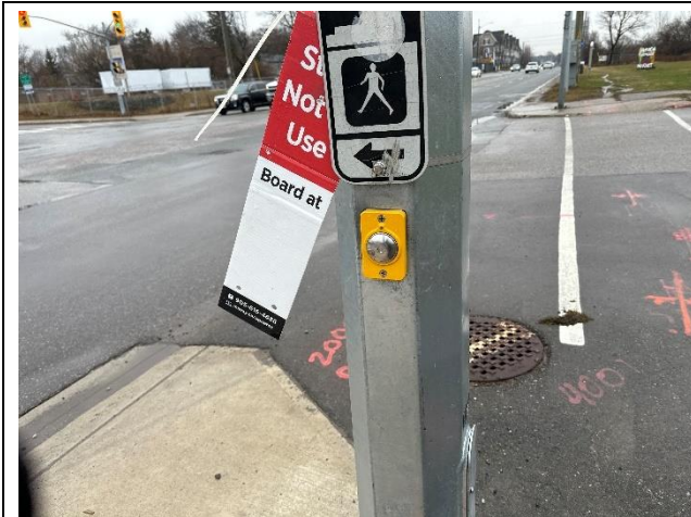
Exhibit 21: An Example Location with Missing Accessible Pedestrian Signals
