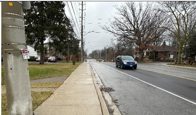
Bicycle lane buffer is missing for southbound traffic approaching the intersection Photo Location: Dixie Road at St. James Avenue, northwest corner, looking north
