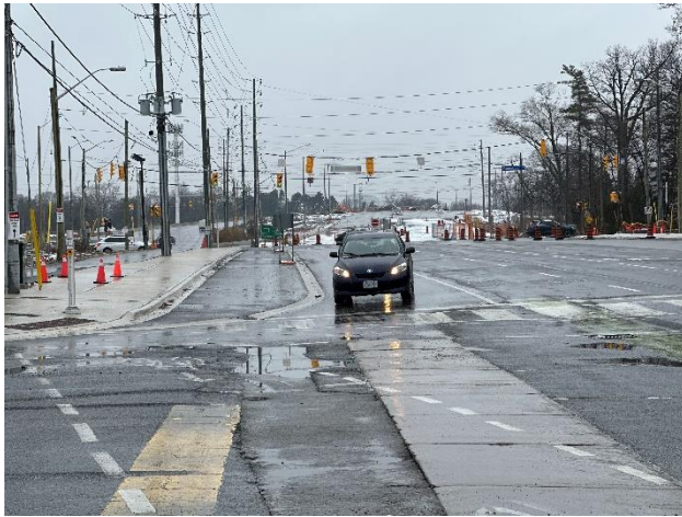
Aggressive turning behaviour (southbound right turning vehicles)
