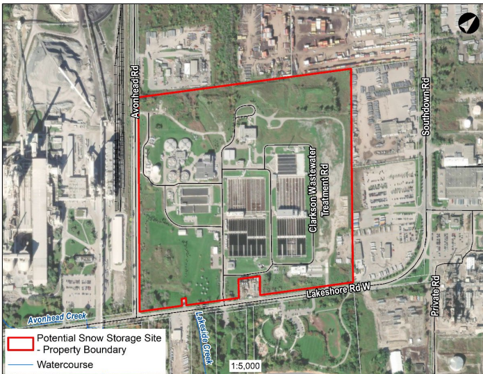
Clarkson Wastewater Treatment Plant
