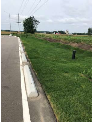
Figure 2. Charleston Sideroad Snow Storage Facility Bioswale
