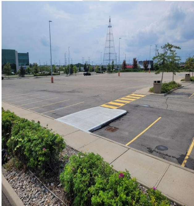
Photo 7. Existing parking lot disturbance, view west.
