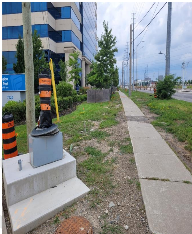
Photo 4. East edge of property, note the disturbance associated with the buried utilities, view north.
