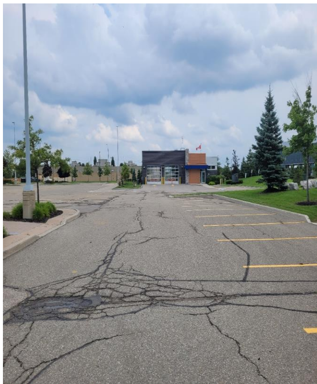
Photo 3. Existing building. Note the light standards and buried utilities (electrical box to the right of the building), view south.
