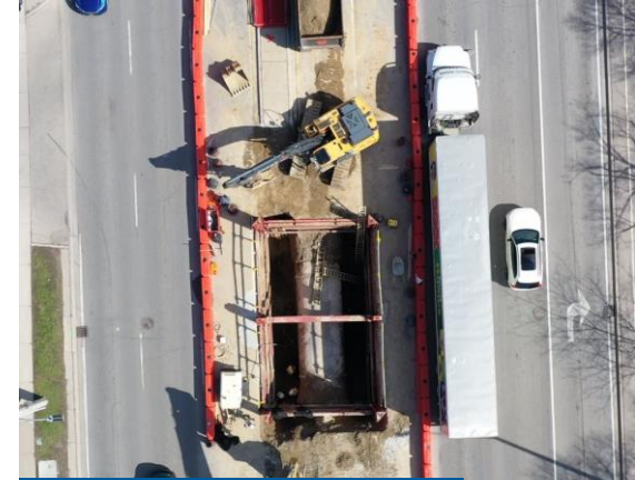
Shaft compound in middle of road.
