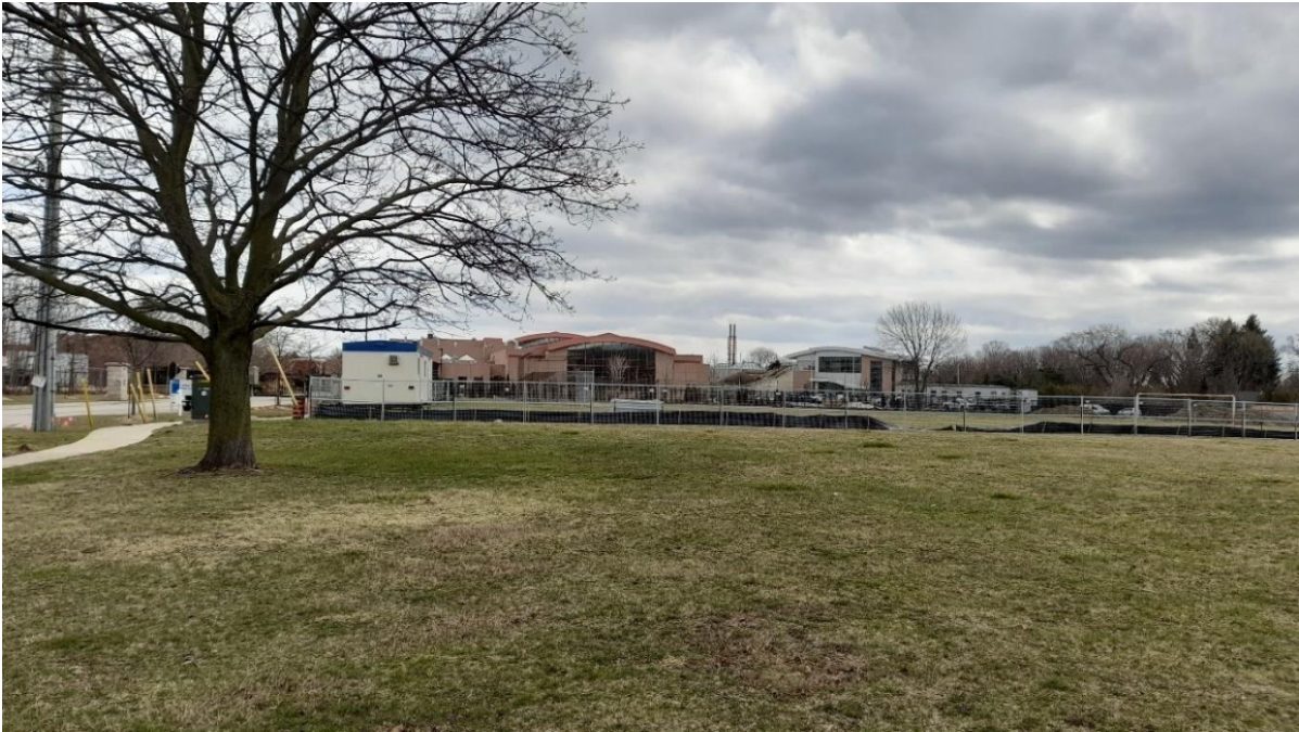
Plate 3: Looking south from within the park to the W.T.P. (A.S.I., 2024).
