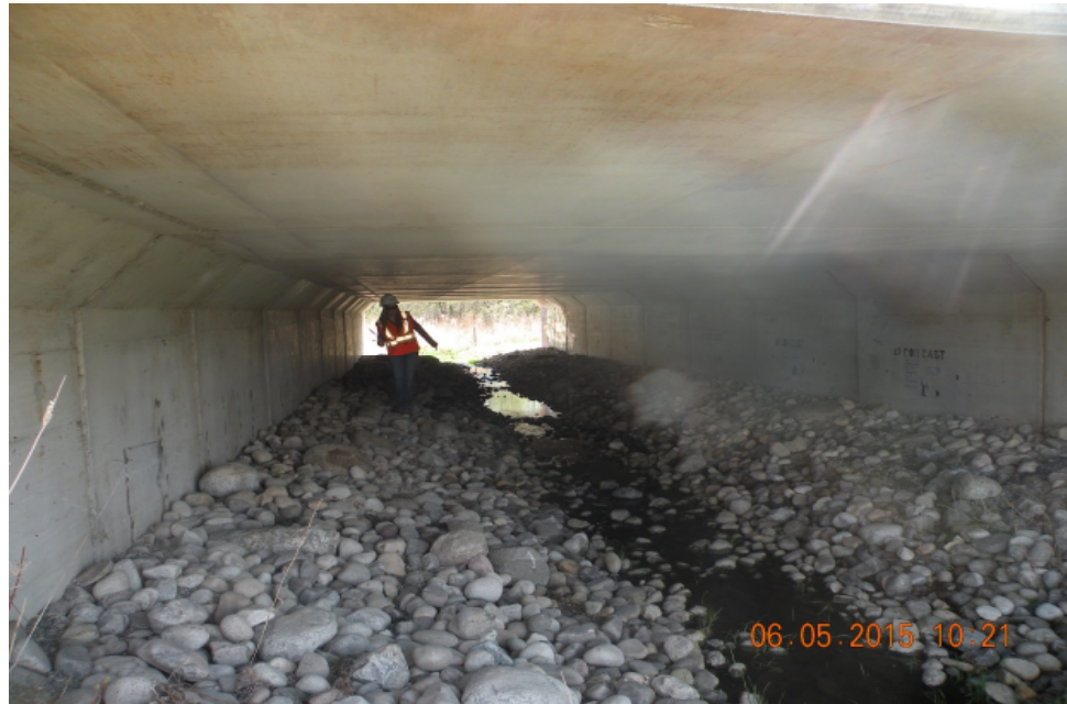
Looking East Through the Structure
