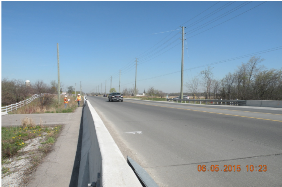
Looking North at Bridge
