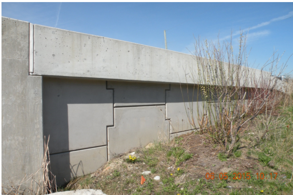
North East Abutment
