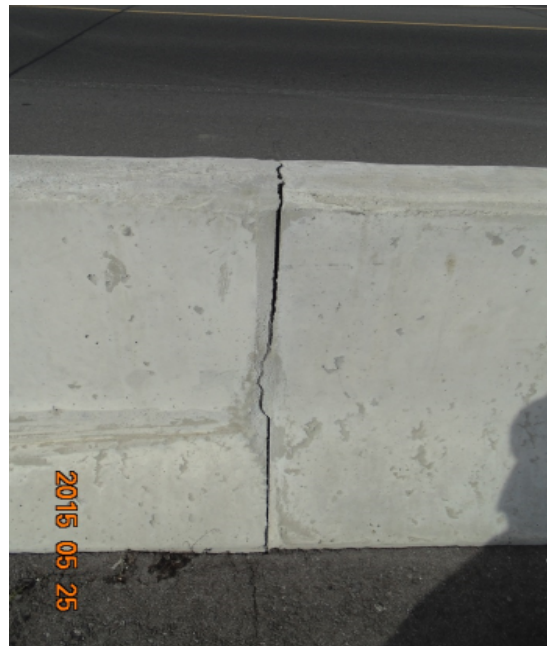
Typical Joint on Barrier Wall
