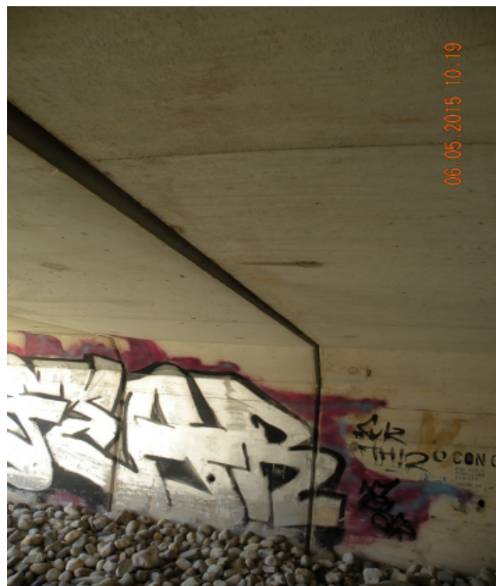
Typical Joint and South Abutment Wall
