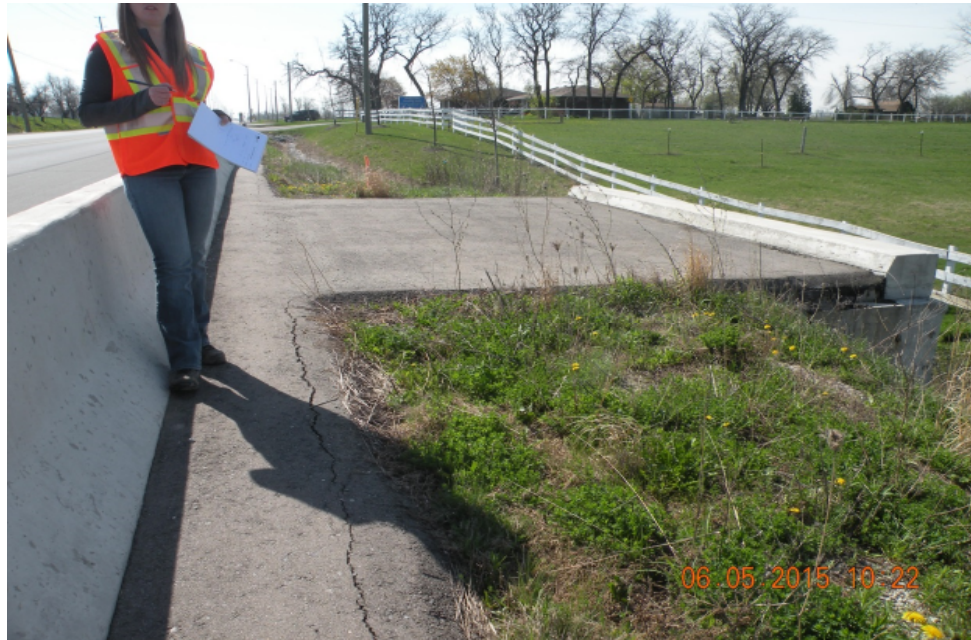
Extension on West Side
