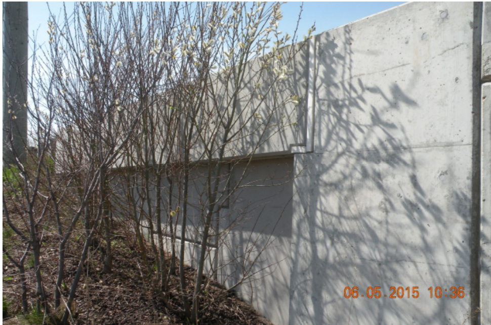
Typical Wingwall / Retaining Wall
