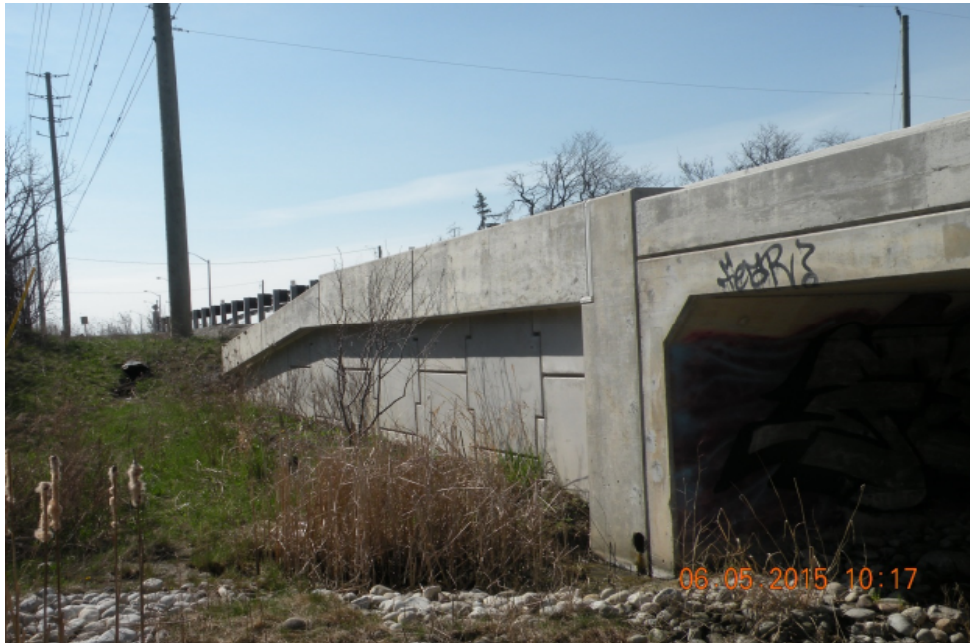
South East Abutment
