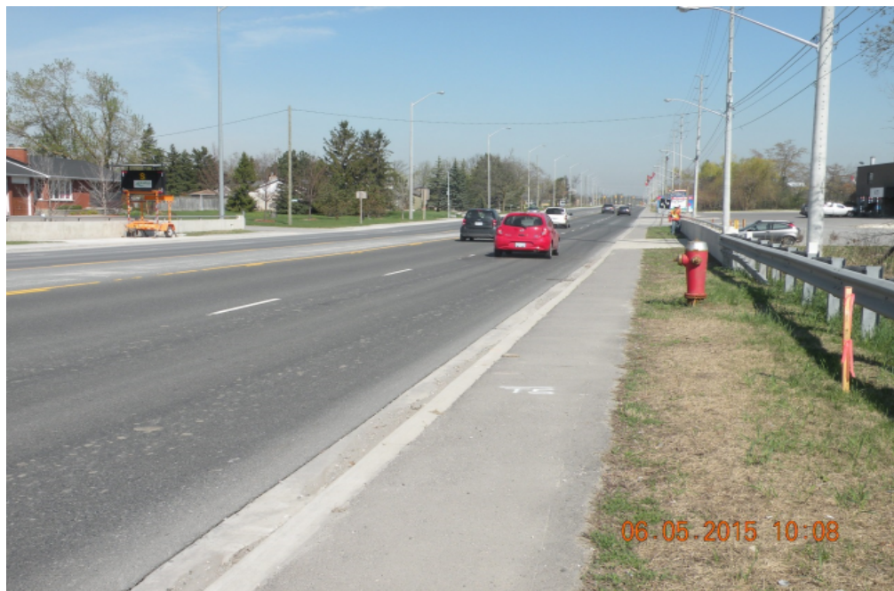
Looking North at Bridge
