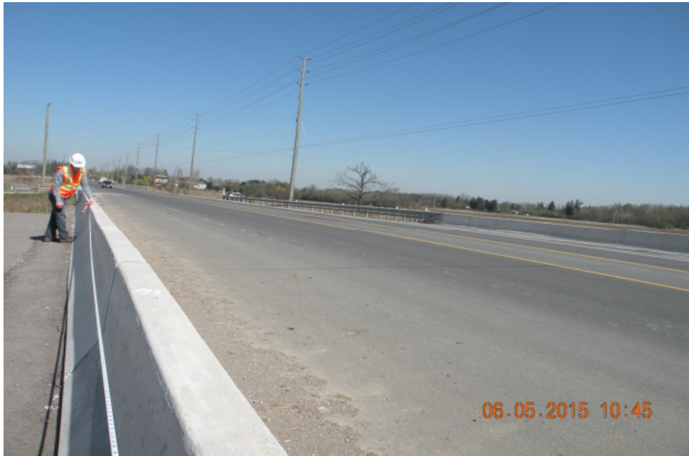
Looking North at Bridge
