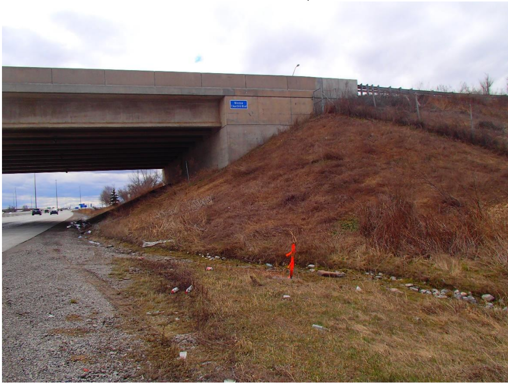
PHOTO 5: North abutment, east side
