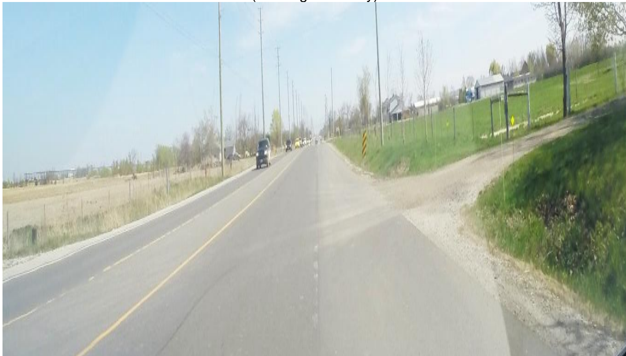
Typical Photograph #6 Winston Churchill Boulevard Southbound at Station 2+900 (Looking Southerly)
