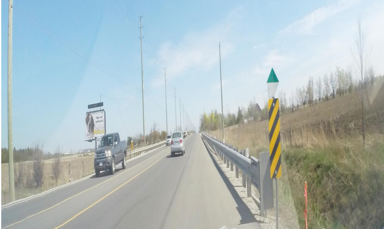
Typical Photograph #5 Winston Churchill Boulevard Southbound at Station 3+800 (Looking Southerly)
