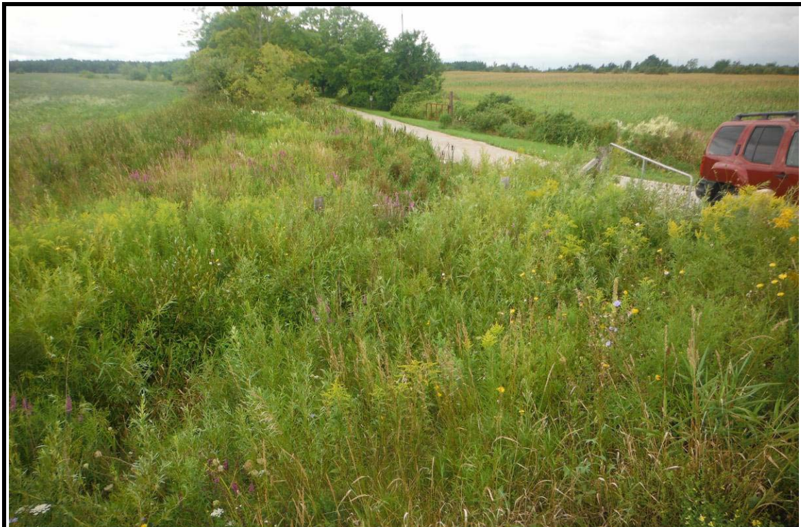
PHOTOGRAPH NO.: 6 - Culvert 3 FROM: Road LOOKING: Upstream at channel COMMENT:
