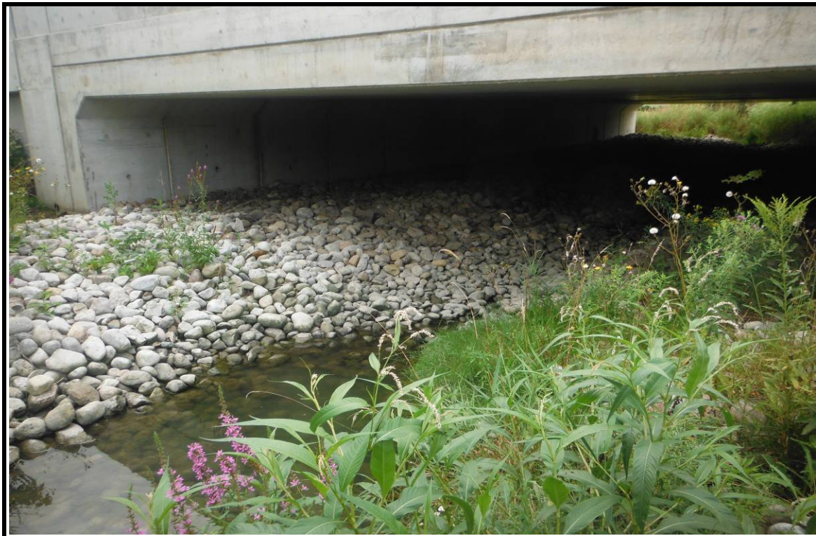
PHOTOGRAPH NO.: 15 - Culvert 10 FROM: Upstream of bridge LOOKING: Through culvert COMMENT:
