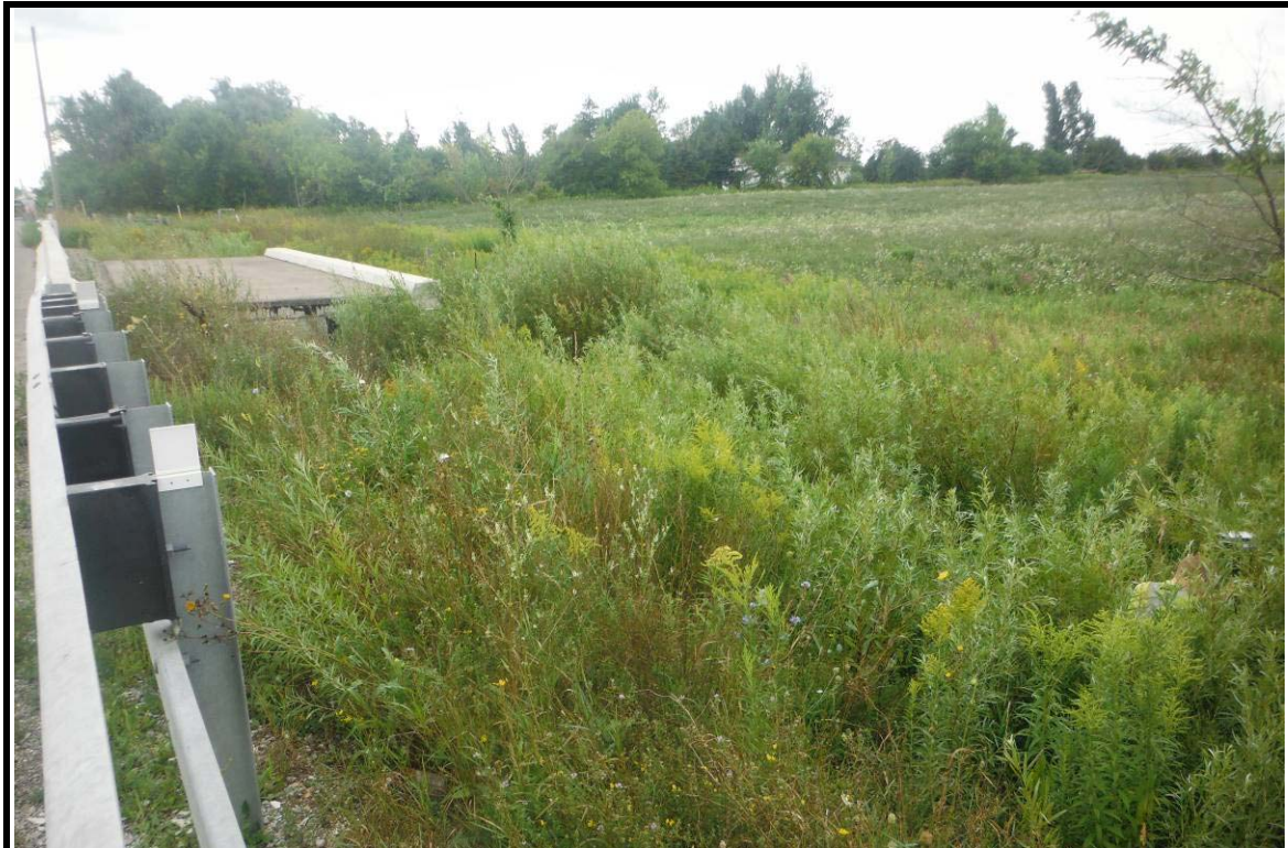
PHOTOGRAPH NO.: 5 - Culvert 3 FROM: From road LOOKING: At culvert 3 COMMENT:
