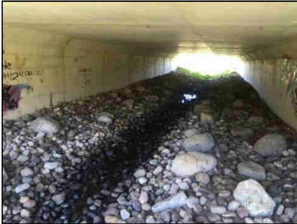
Photo 7. Levi Creek South – Looking West through Culvert *Dry
