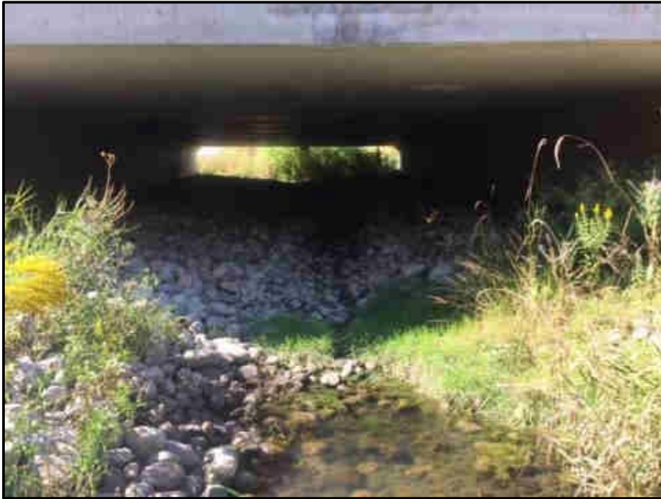
Photo 1. Mullet Creek – Looking West through the Culvert from Downstream * Instream Culvert Dry
