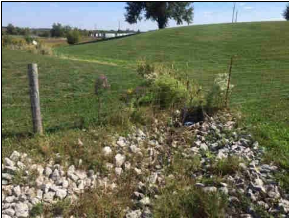
Photo 4. Drainage Feature # 1 – East of Winston Churchill Blvd. – Dry Swale
