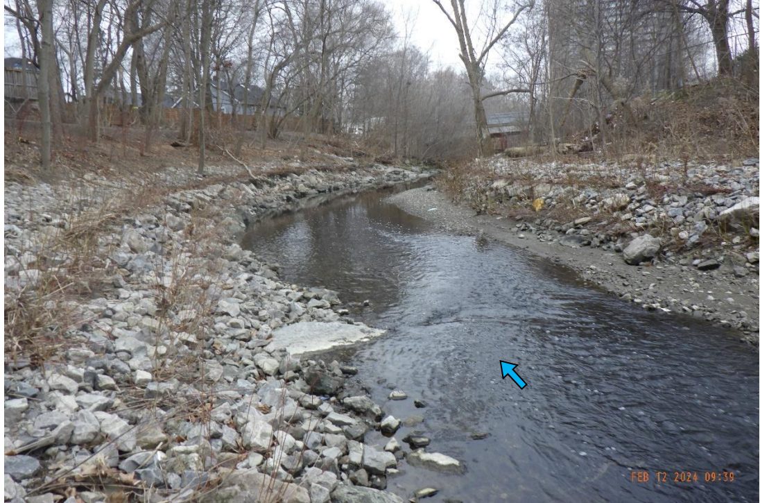
Upstream of Kirwin Drive and the subject sewer crossing location, Cooksville Creek was armoured with riprap and armourstone grade controls. The arrow denotes flow direction.
