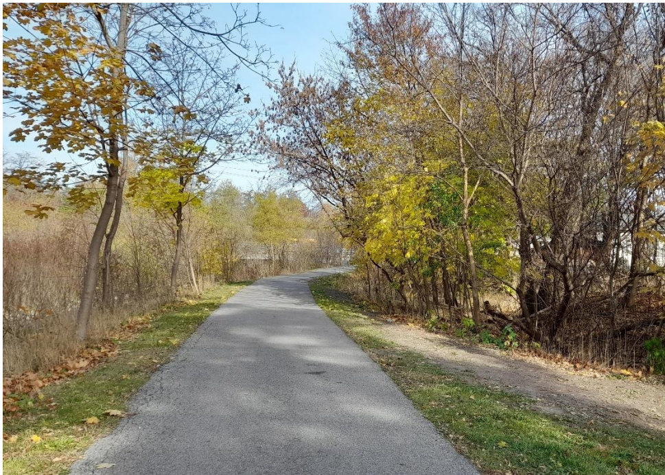
Image 10: Preferred Route: Land south of disturbed Cookville Creek trail requires Stage 2 Survey.
