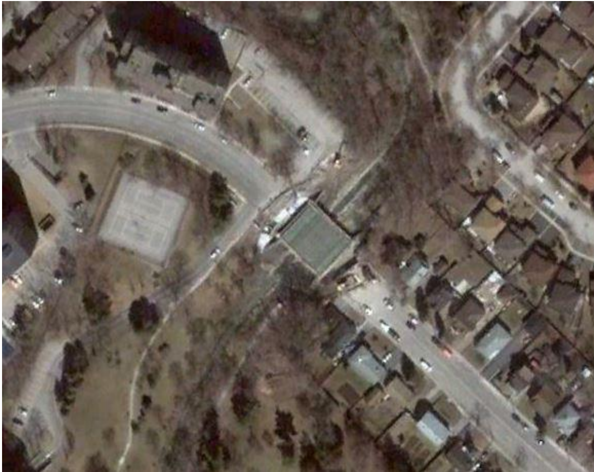
Image 19: Reconstruction of Kirwin Avenue Bridge over Cooksville Creek in 2007 (Google Earth Pro, 2023).
