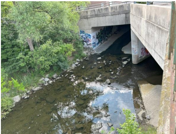
Photo 9: Cooksville Creek, upstream of Jaguar Valley Dr, double concrete culverts.
