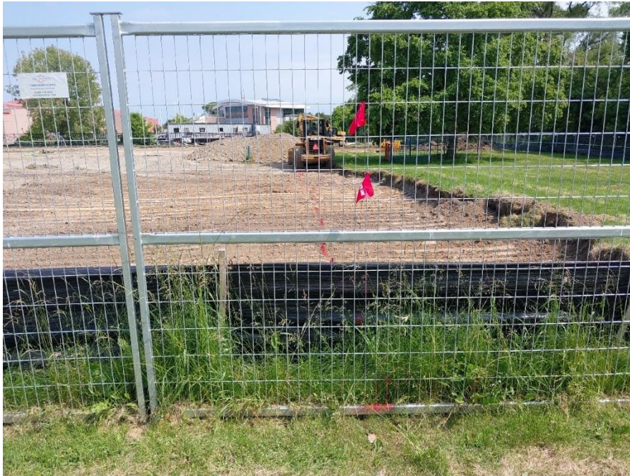
Image 7: Construction of Yard Piping Upgrades project underway; further work required
