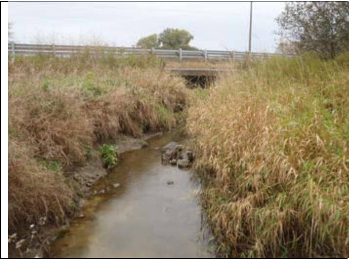
Photo 13: Crossing 14 downstream – looking upstream
