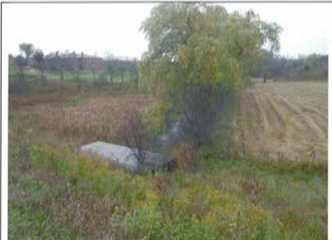
Photo 3: Crossing 6 upstream - looking upstream from Mayfield Road
