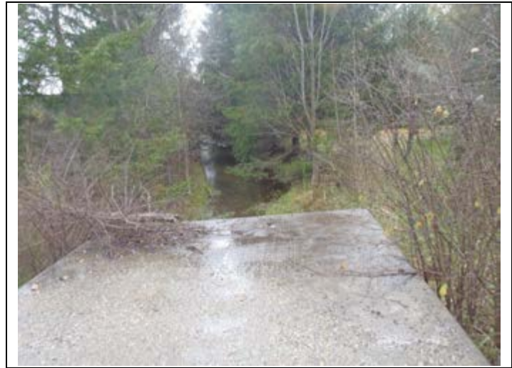
Photo 2: Crossing 5 upstream – looking upstream from Mayfield Road
