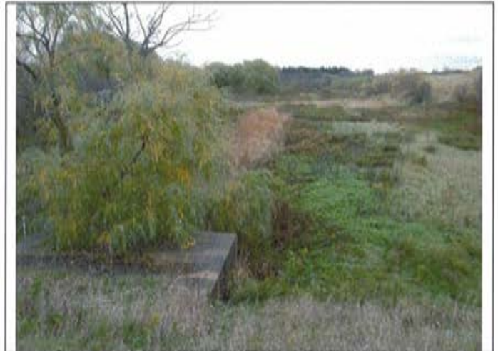
Photo 4: Crossing 6 downstream - looking upstream
