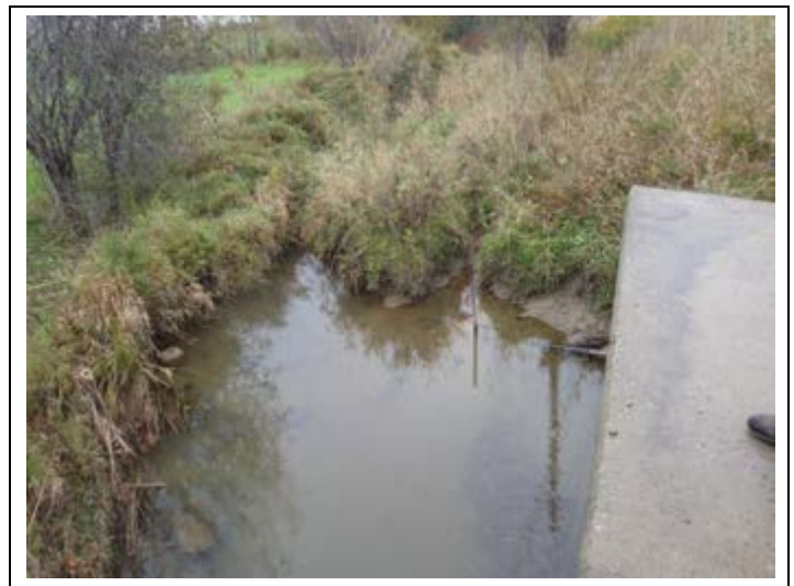
Photo 10: Crossing 14 upstream – looking upstream from Mayfield Road
