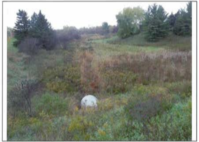
Photo 2: Crossing 7 upstream - looking upstream from Mayfield Road
