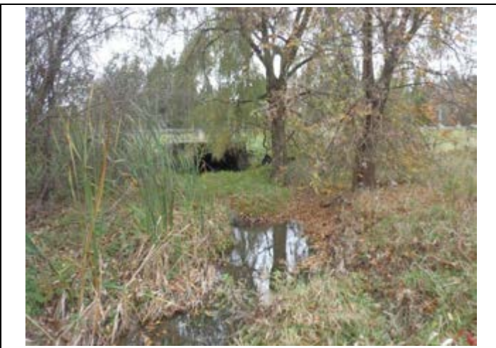
Photo 3: Crossing 5 downstream – looking upstream toward Mayfield Road
