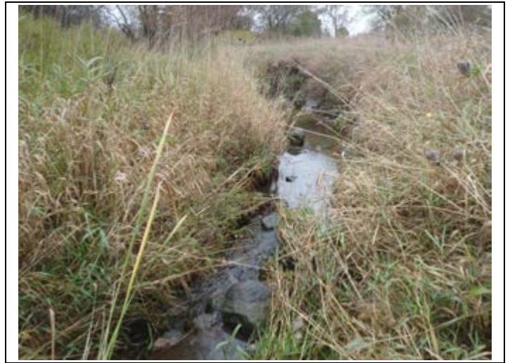
Photo 16: Crossing 14 downstream - looking downstream
