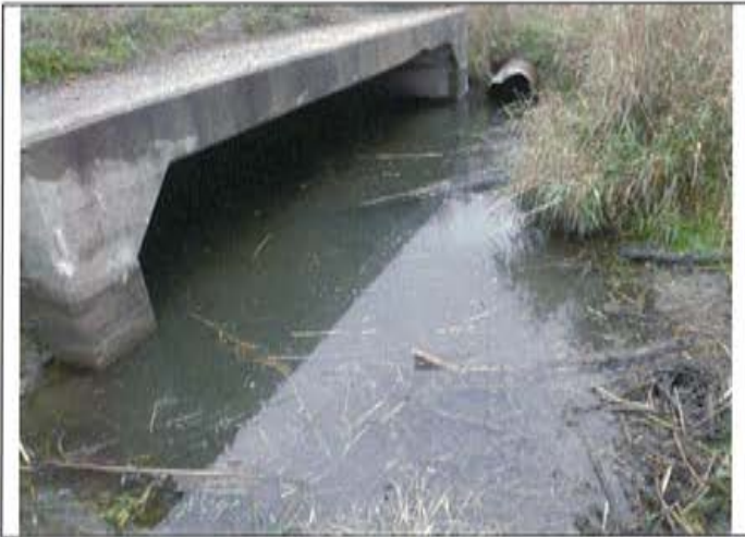
Photo 9: Crossing 12 downstream – looking upstream at beaver dam and culvert
