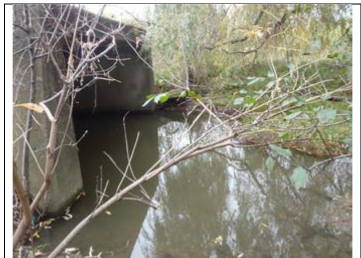
Photo 6: Crossing 5 downstream – downstream end of culvert
