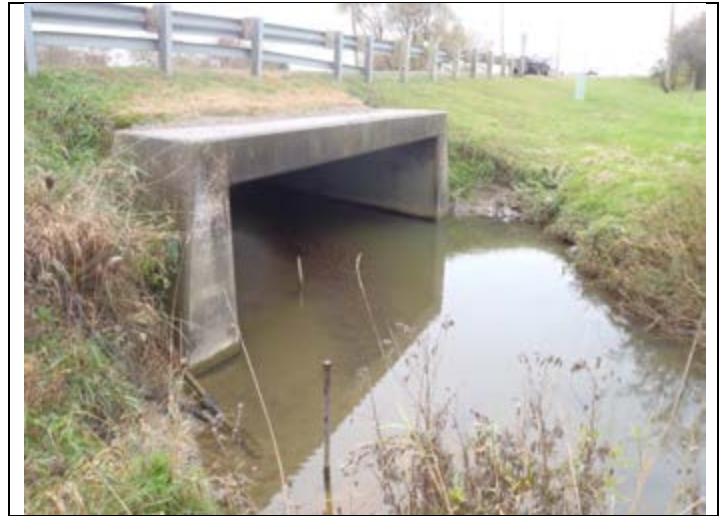
Photo 8: Crossing 14 upstream – upstream end of culvert
