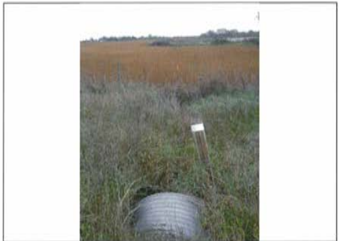
Photo 12: Crossing 13 downstream – looking downstream
