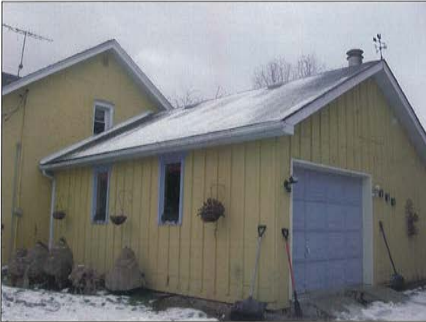
Plate 11: Full view of northern elevation
