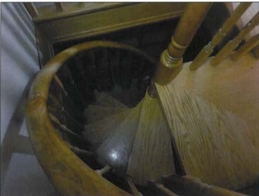
Plate 45: Detail of spiral staircase.
