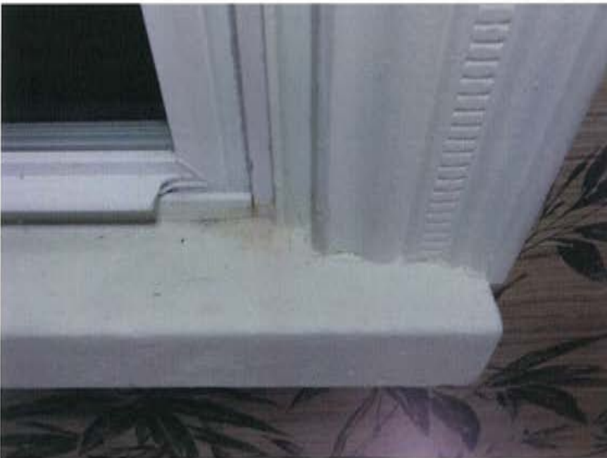
Plate 37: Detail of wooden sill found in the Living Room.
