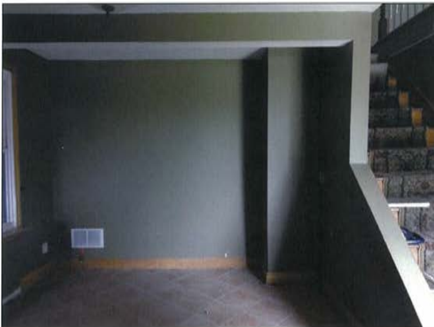
Plate 51: View from south of main entrance looking west showing Family Room and location of previous partition wall adjacent to staircase.
