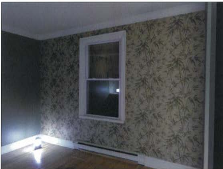
Plate 35: View of original window opening in Living Room on first floor.
