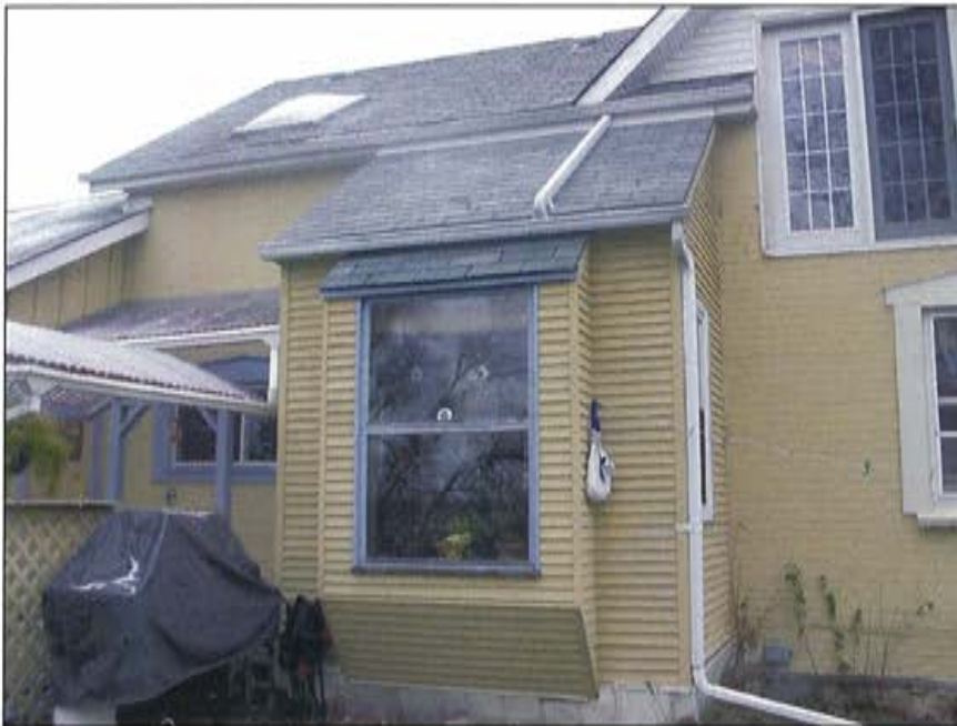
Plate 17: View of small extension on western elevation.
