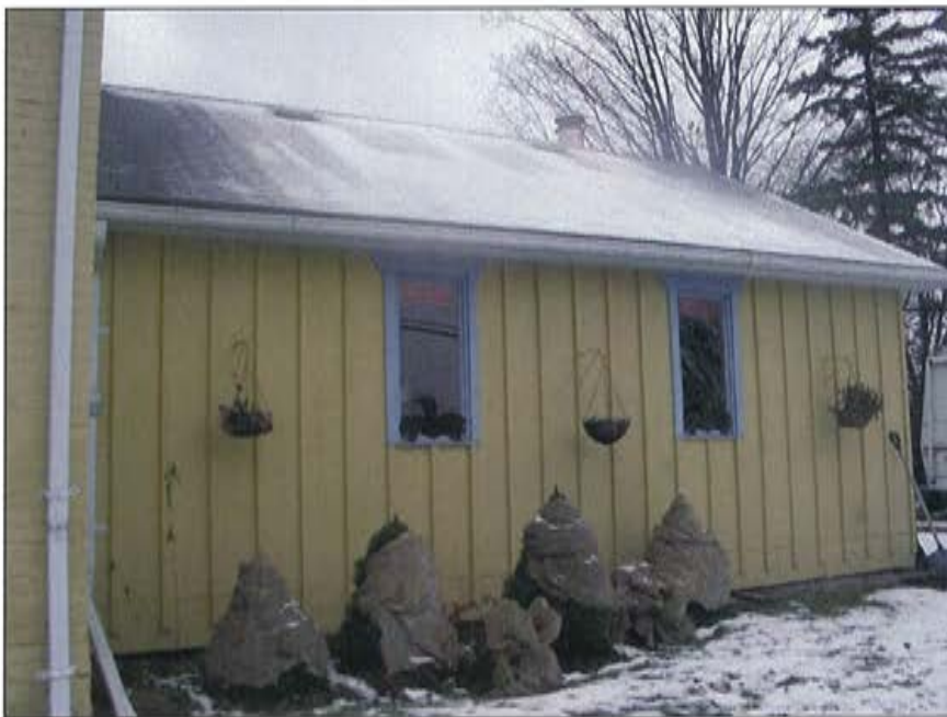
Plate 10: Extension on northern elevation
