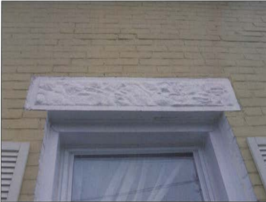
Plate 5: Dressed concrete lintels above windows on eastern elevation
