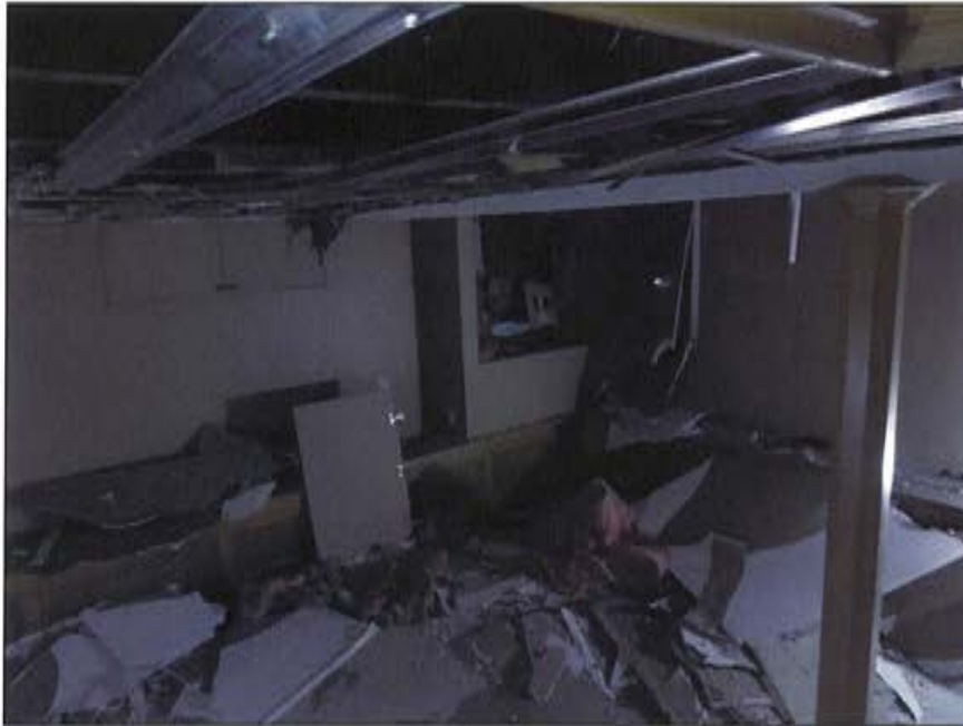
Plate 62: View of Area 1 looking northeast from spiral staircase.
