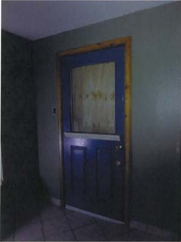
Plate 50: View of wooden door located on northern elevation of rear addition.
