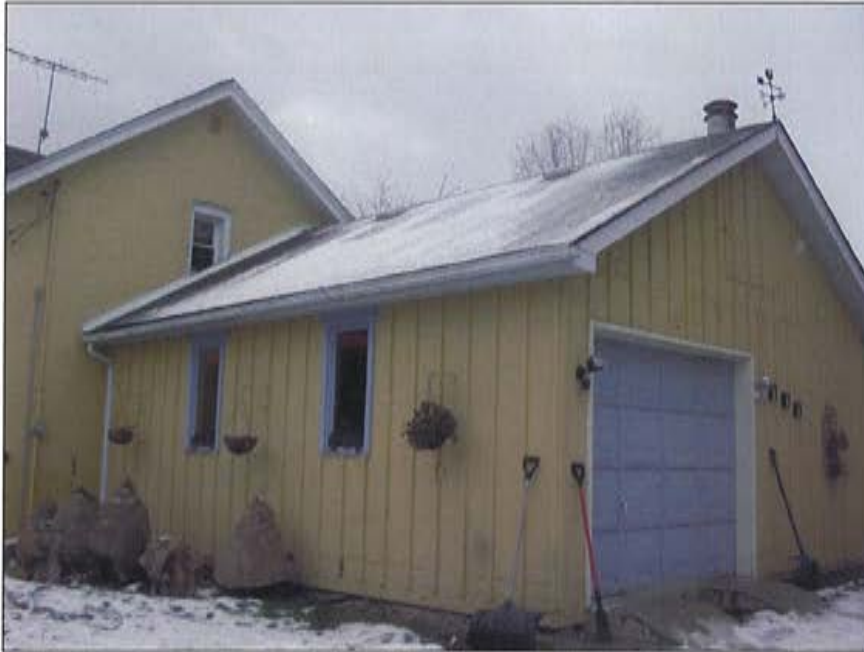
Plate 11: Full view of northern elevation
