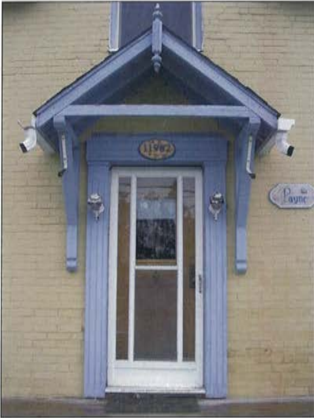
Plate 9: Front entrance detail
