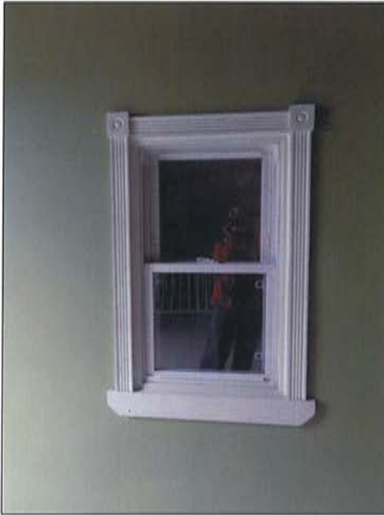
Plate 60: View of double-hung window on north wall of upper floor; the size of this structural opening has been altered through filling in of brick on the east side.
