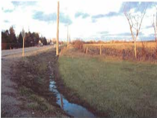
Plate 33: View to northeast along Mayfield Rd towards open fields. Potential exists beyond disturbed ROW.
