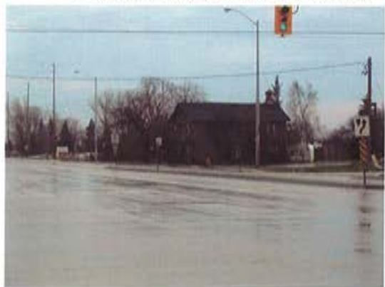
Plate 4: View to south-southeast along Airport Rd looking at former Blacksmith Shop.
