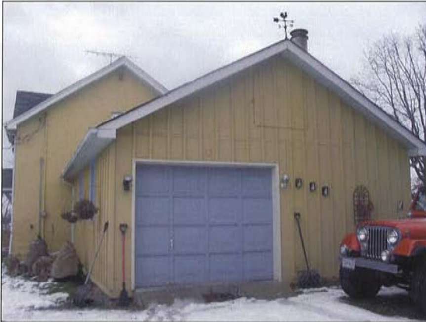
Plate 13: View of extension and upper storey opening
