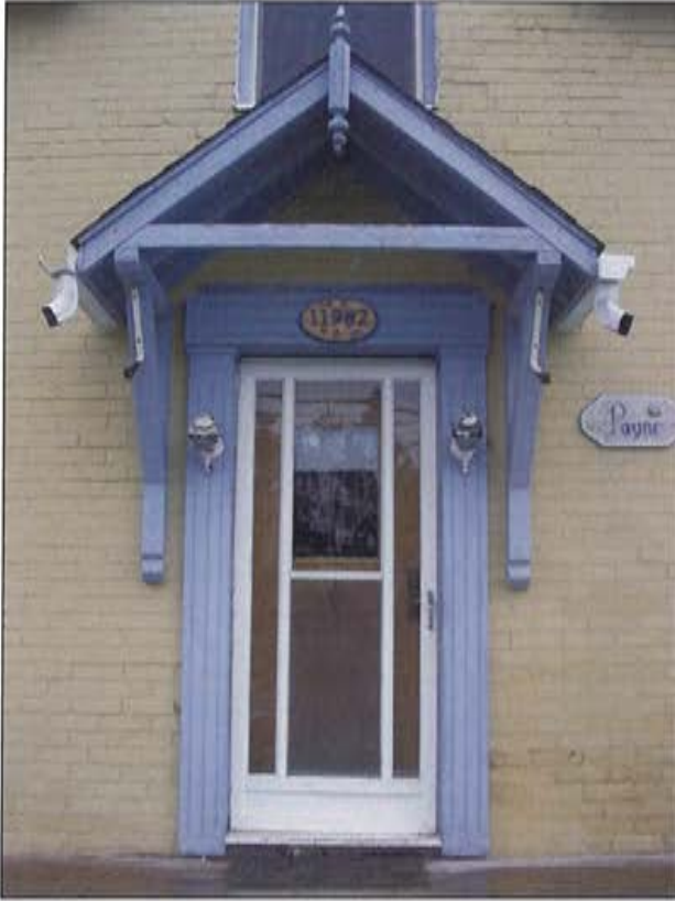
Plate 9: Front entrance detail
