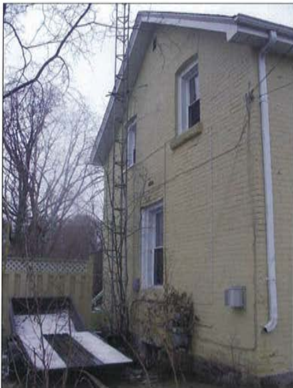
Plate 21: View of unaltered southern elevation.
