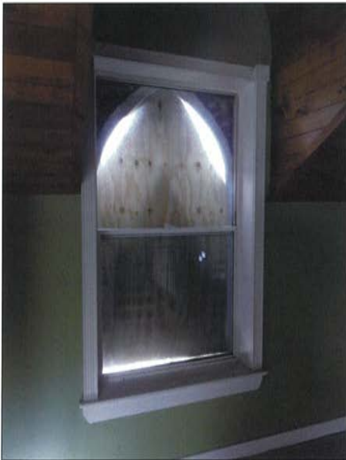
Plate 57: View of pointed window on east wall showing rectangular window and pointed structural opening.
