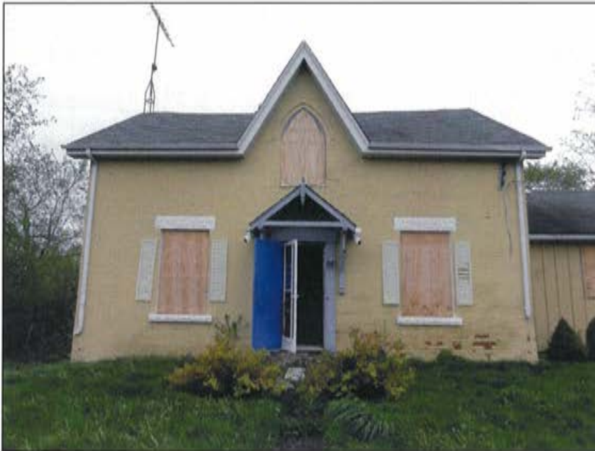
Plate 30: View of eastern elevation of residence in May 2011.
