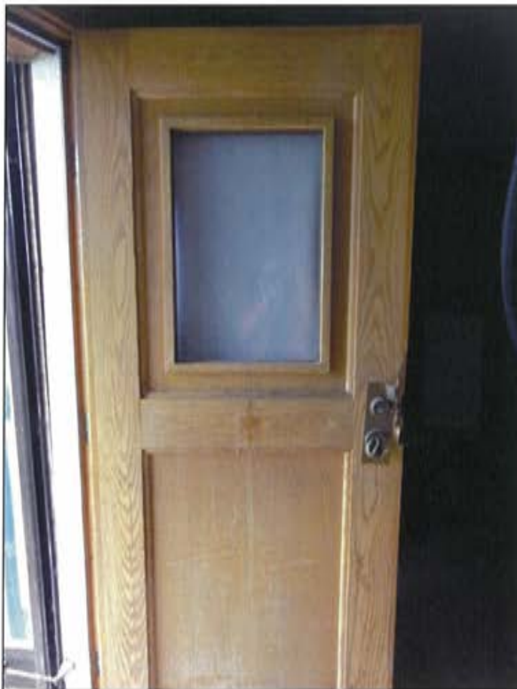
Plate 33: View of modern wood door located on eastern elevation, showing recessing panels and single pane of glass.
