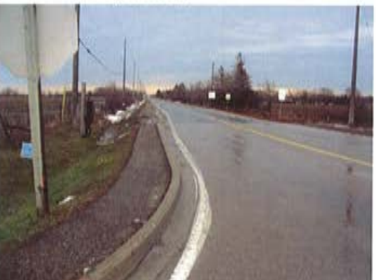
Plate 17: View to southeast along McVean Dr. Potential exists beyond graded shoulder.
