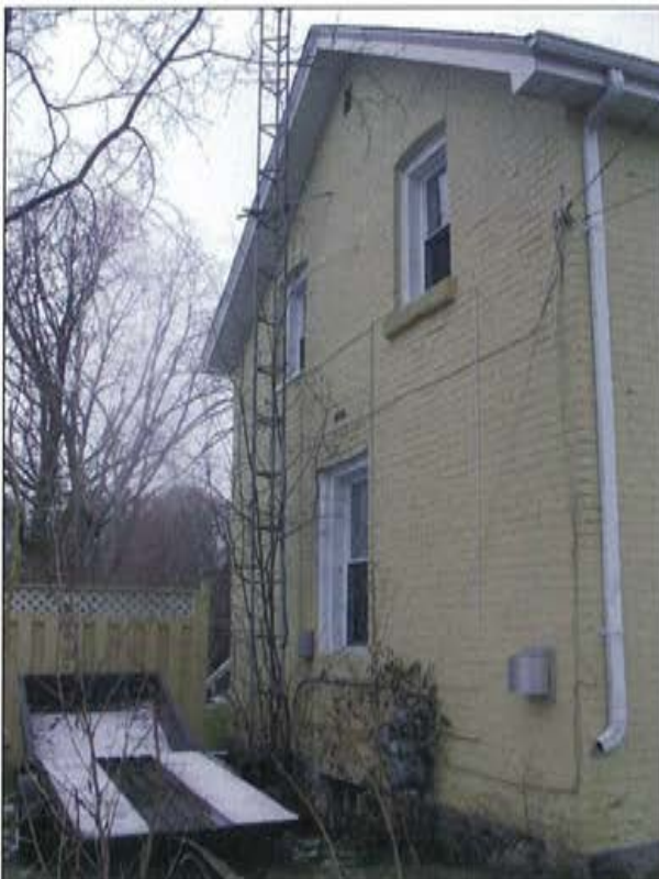
Plate 21: View of unaltered southern elevation.
