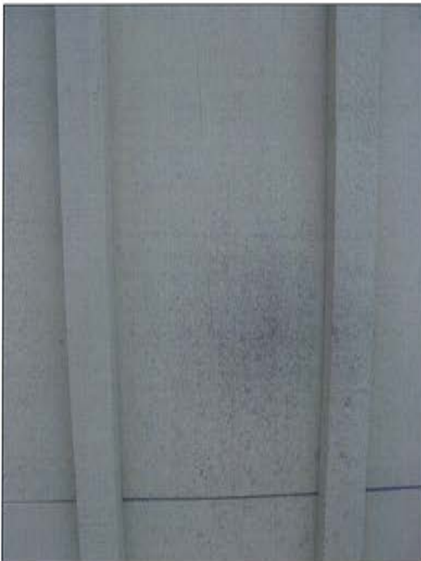
Plate 12: Board and batten detail on extension
