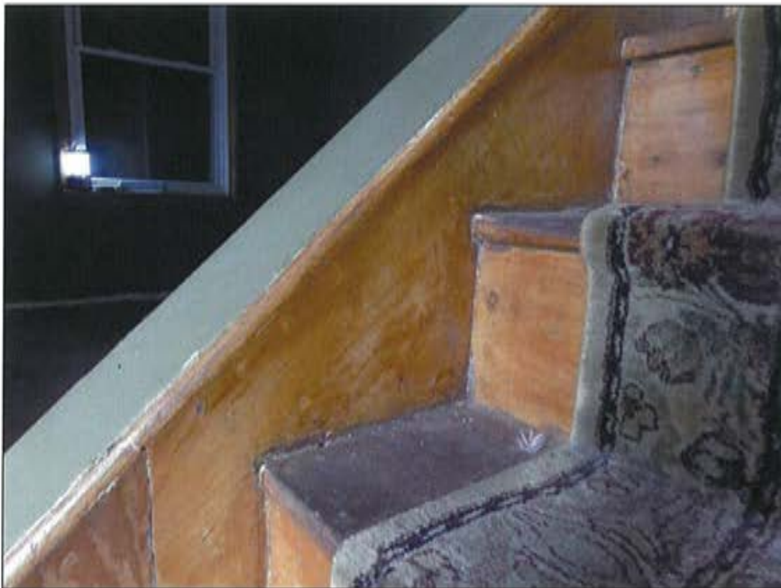
Plate 55: Detail of central staircase showing solid wood wall string, nosing, tread, and risers that appear to date to construction of the house.
