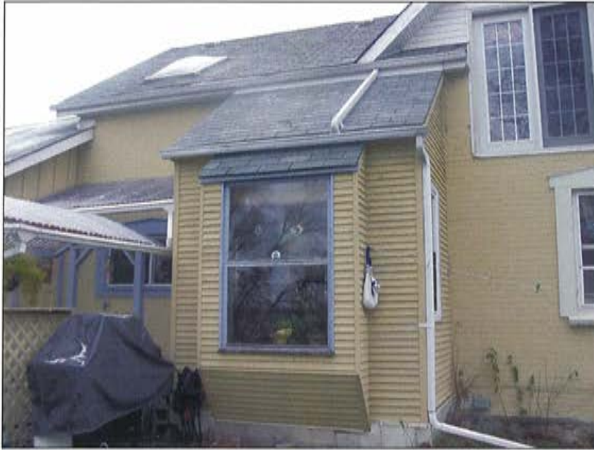
Plate 17: View of small extension on western elevation.
