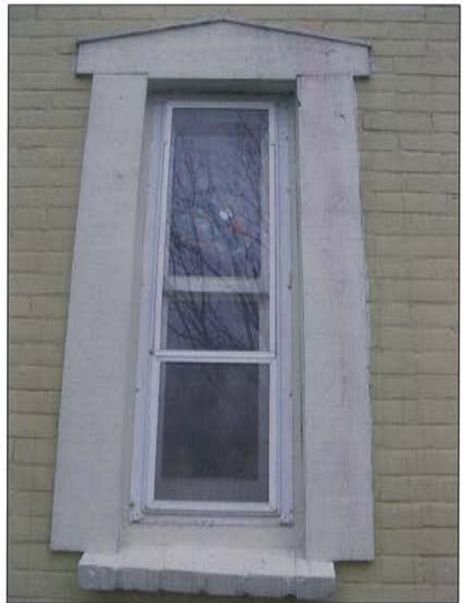
Plate 19: View of structural opening, featuring brick sills.
