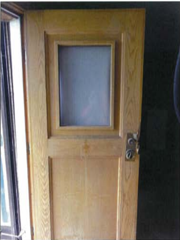
Plate 33: View of modern wood door located on eastern elevation, showing recessing panels and single pane of glass.
