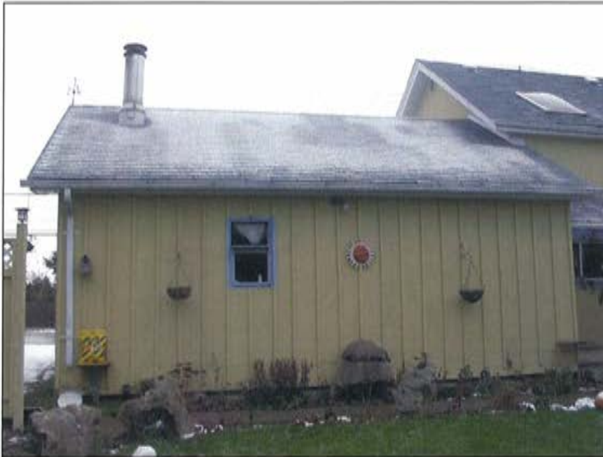
Plate 15: Western elevation of extension
