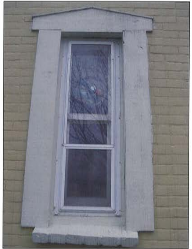
Plate 19: View of structural opening, featuring brick sills.
