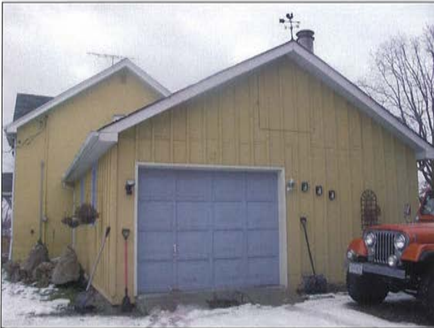
Plate 13: View of extension and upper storey opening
