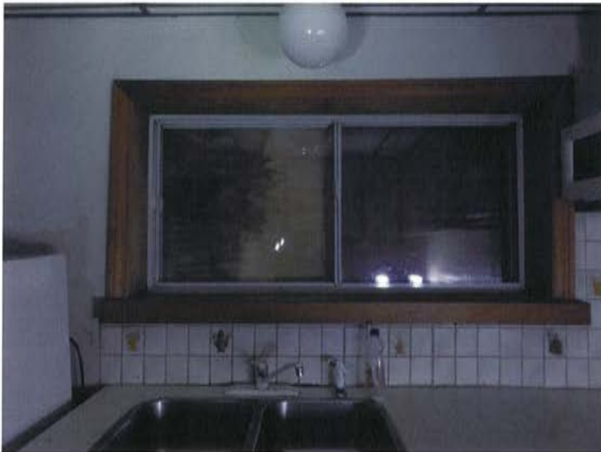
Plate 43: Detail of horizontal window (new structural opening) in the Kitchen.
