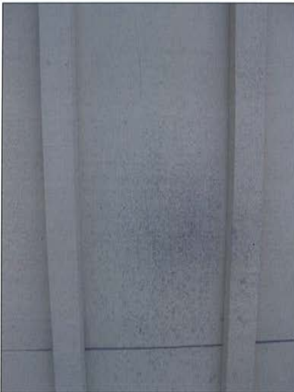
Plate 12: Board and batten detail on extension
