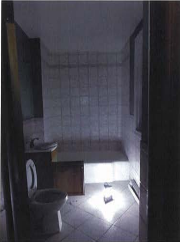
Plate 46: View of bathroom from Kitchen.
