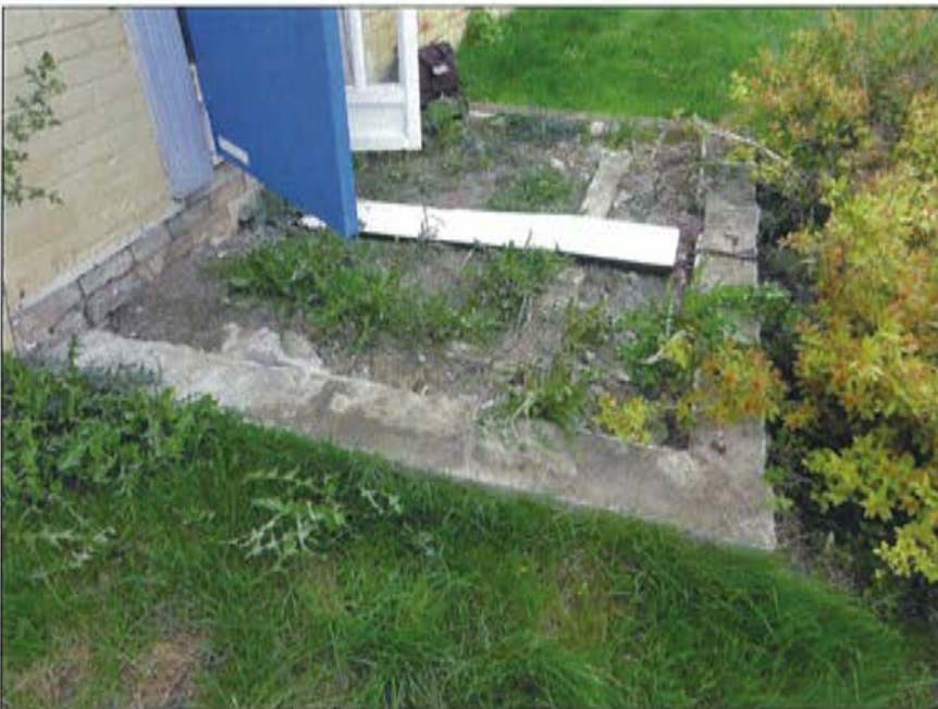
Plate 31: Detail of primary entrance to residence in May 2011 showing location of previous wooden deck and detail of poured concrete base.
