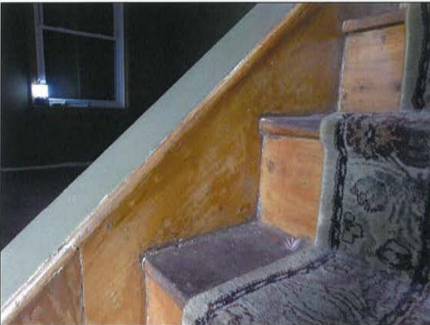
Plate 55: Detail of central staircase showing solid wood wall string, nosing, tread, and risers that appear to date to construction of the house.
