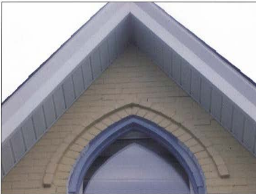
Plate 6: Inset, arched window and brick voussoirs, eastern elevation.
