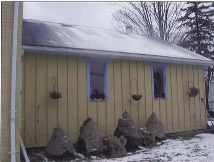
Plate 10: Extension on northern elevation
