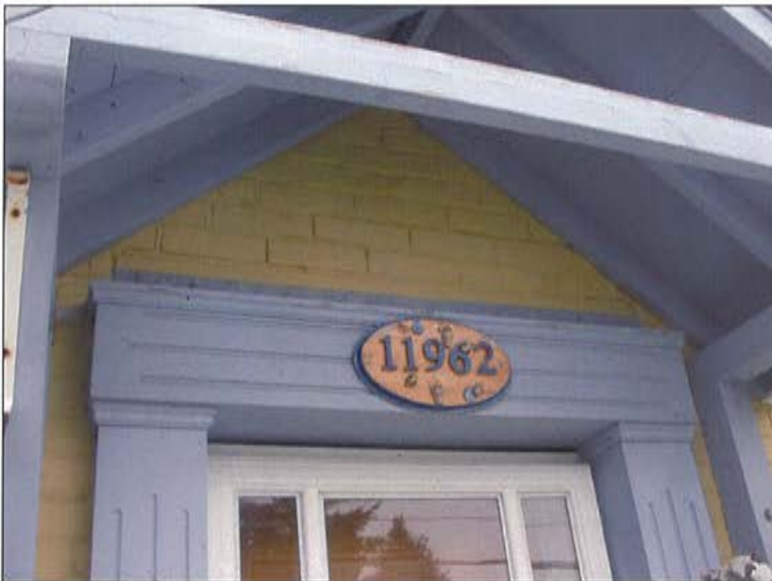
Plate 8: Front entrance, eastern elevation, showing dressed concrete lintel
