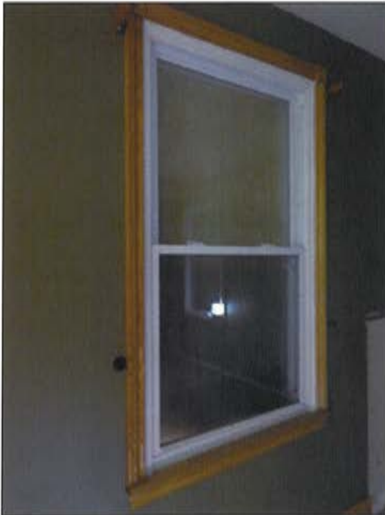
Plate 52: View of original structural opening on east wall of Family Room showing new window, trim and sill.
