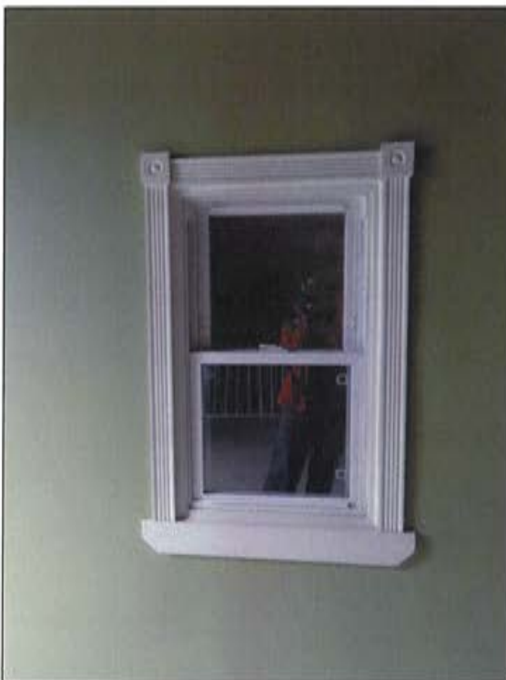
Plate 60: View of double-hung window on north wall of upper floor; the size of this structural opening has been altered through filling in of brick on the east side.
