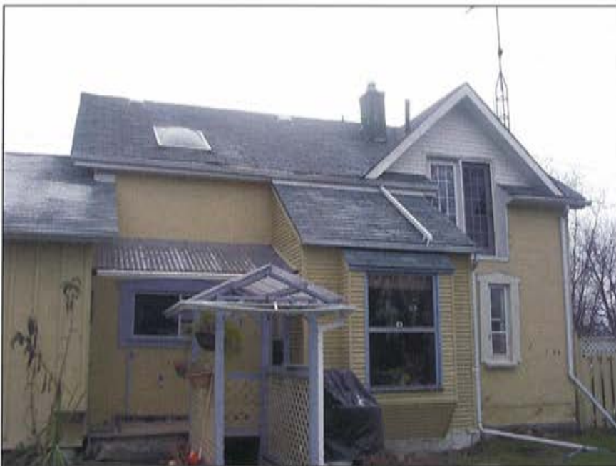
Plate 16: Western elevation of original portion of residence, showing remnant veranda
