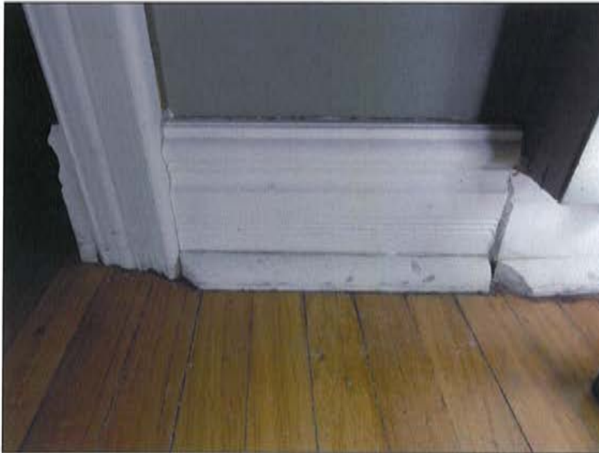
Plate 38: Detail of narrow hardwood flooring found in the living room.
