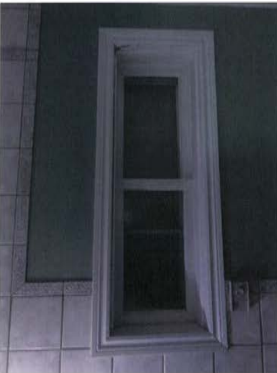
Plate 47: View of window in bathroom showing wooden sashes and older wooden trim.
