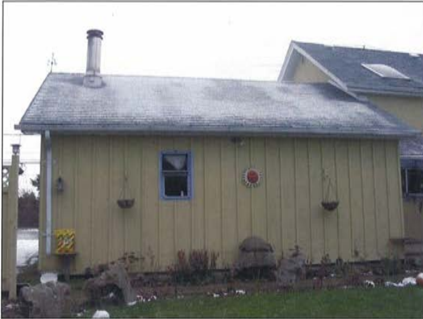
Plate 15: Western elevation of extension
