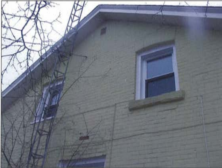
Plate 22: View of upper storey windows on southern elevation, showing new windows and retention of original structural opening and brick voussoirs in the upper storey.
