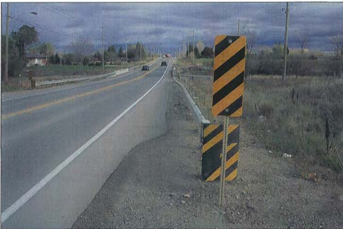
Photo 18: West approach, south side, looking east.
