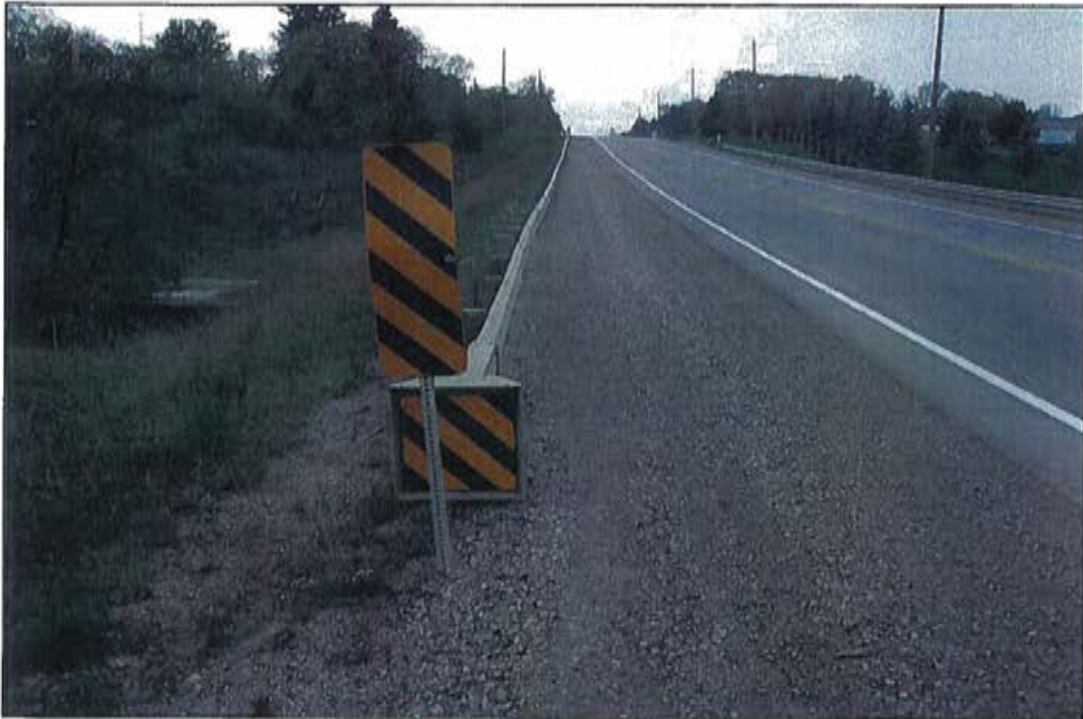
Photo 5: East approach, south side.
