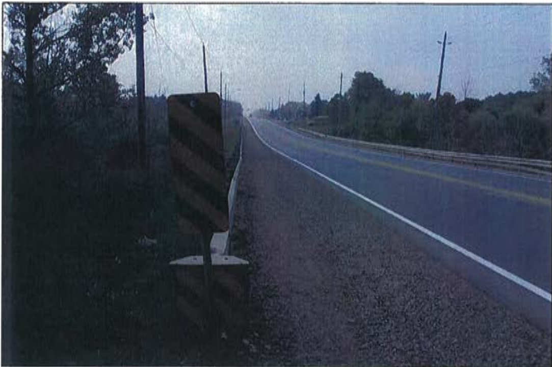
Photo 5: East approach, south side.
