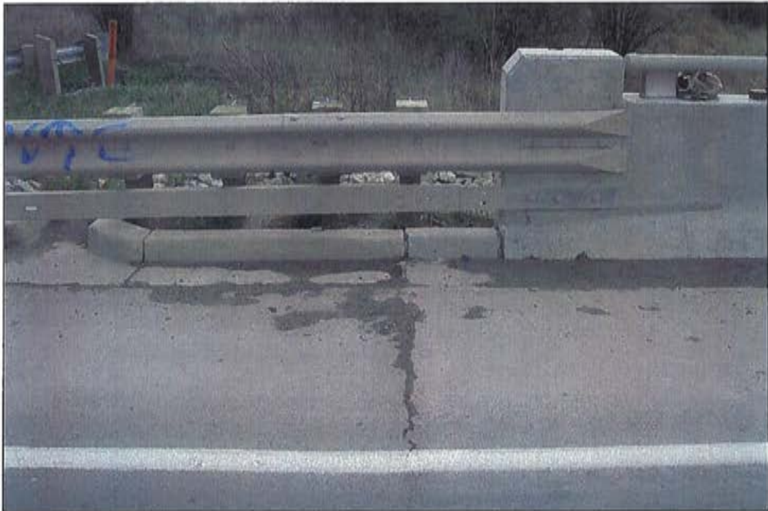
Photo 9: Steel beam guide rail connection, east approach, south side.
