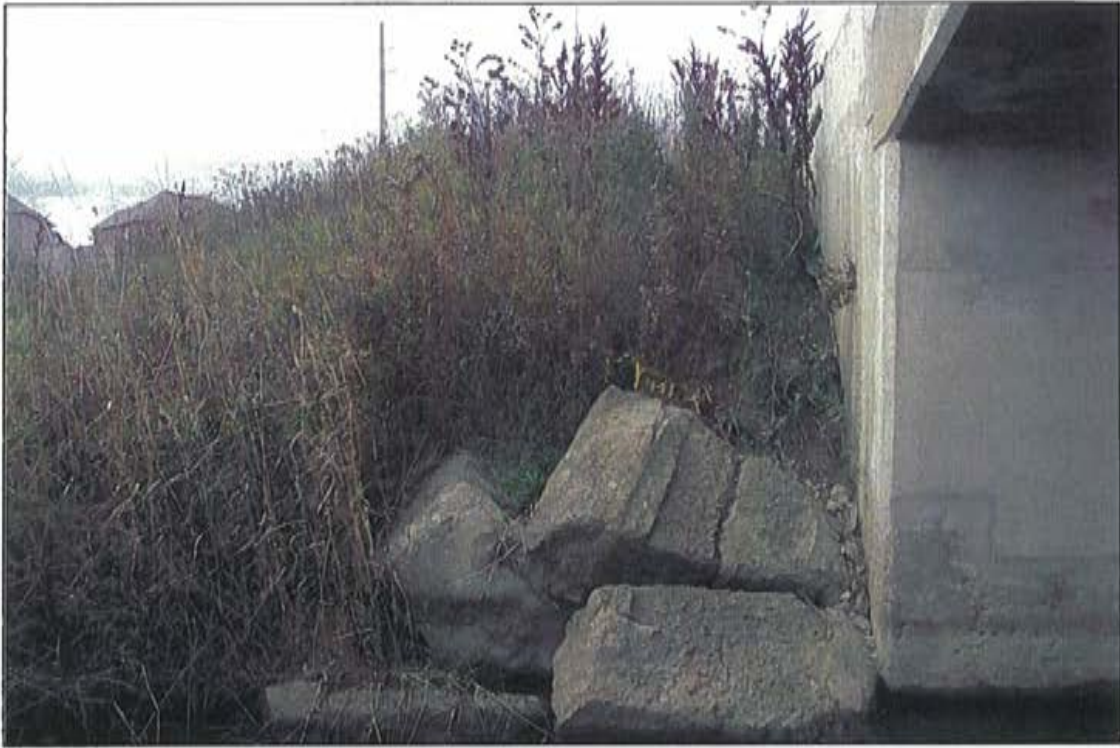
Photo 33: Embankment, west approach, south side.
