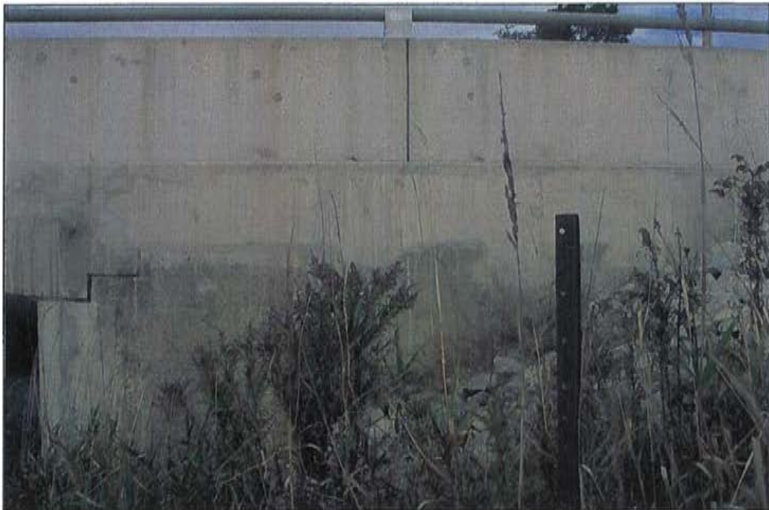
Photo 38: Wingwall, east approach, south side.
