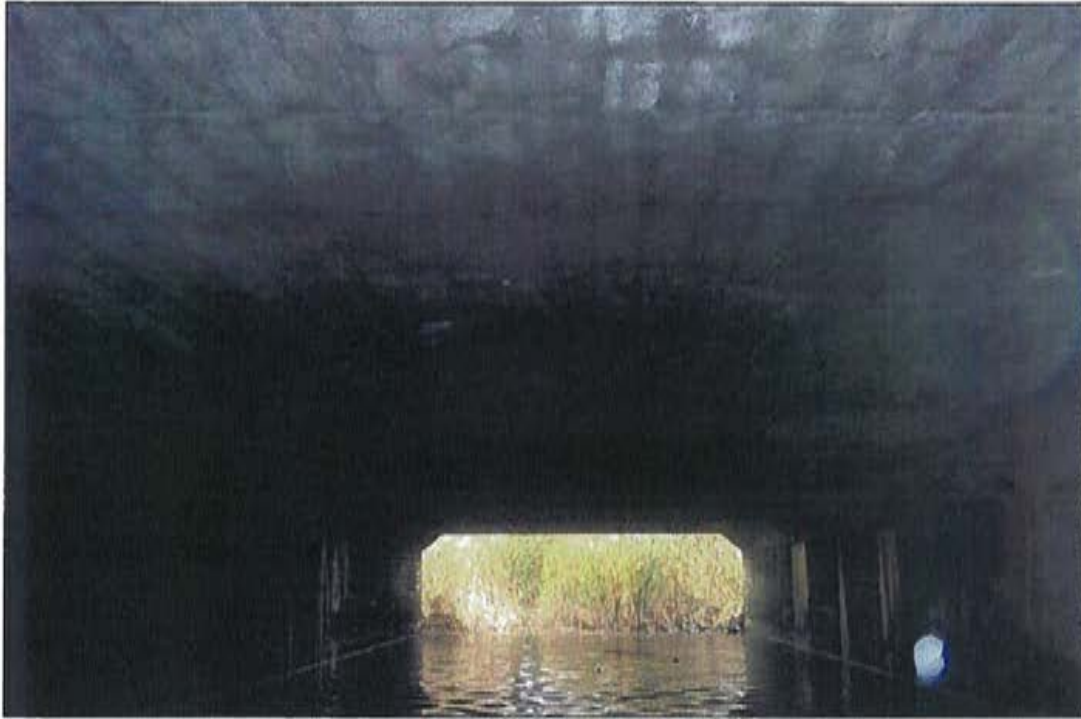
Photo 13: Culvert barrel, looking north.
