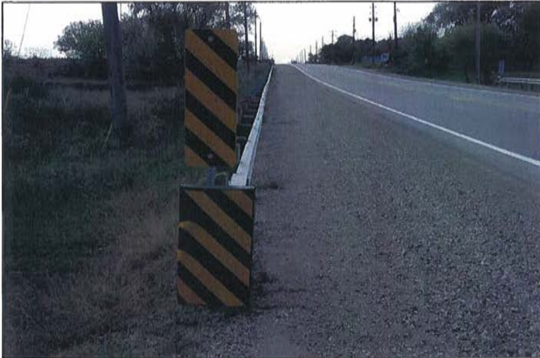
Photo 5: East approach, south side.
