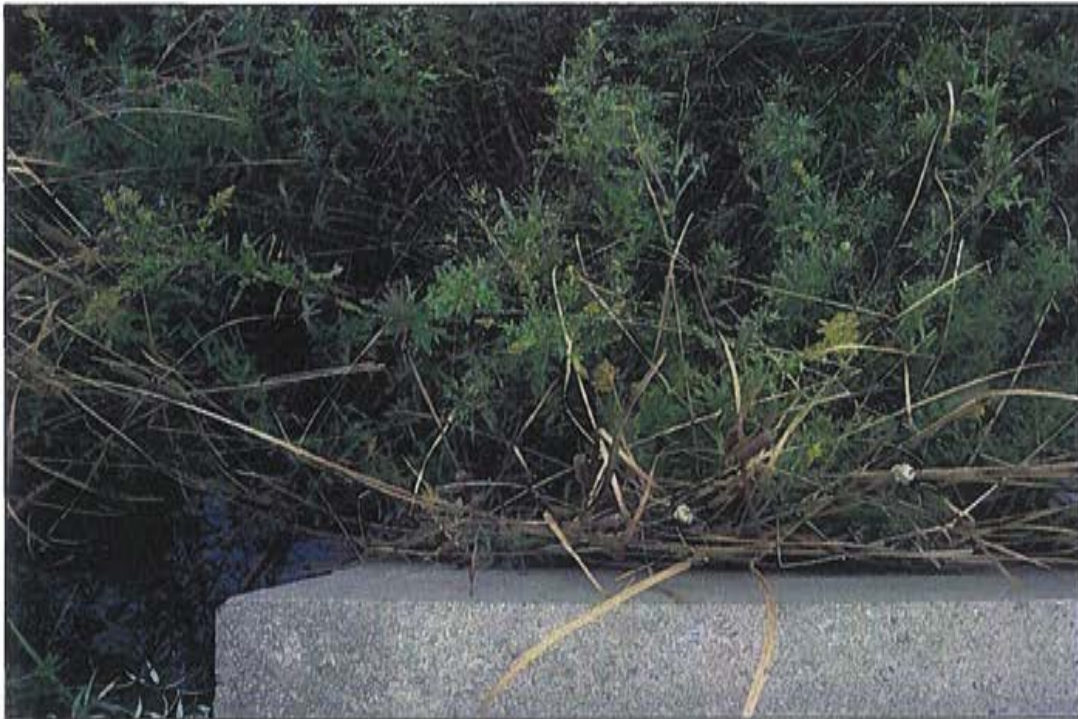
Photo 19: Embankment, west approach, south side.
