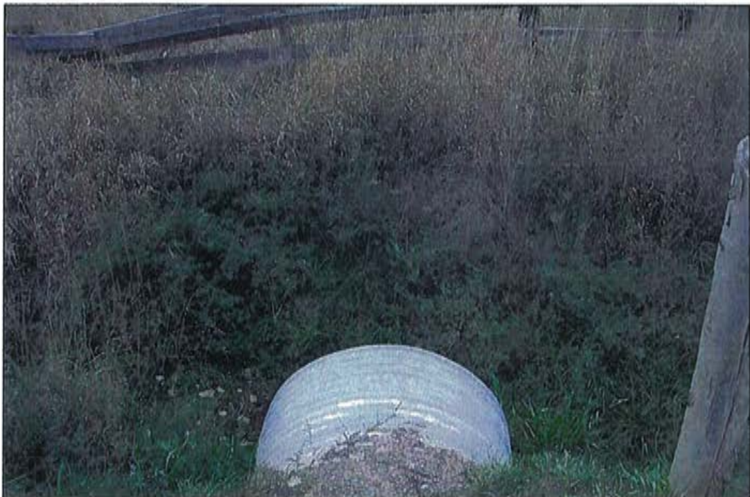
Photo 2: Inlet, looking north.
