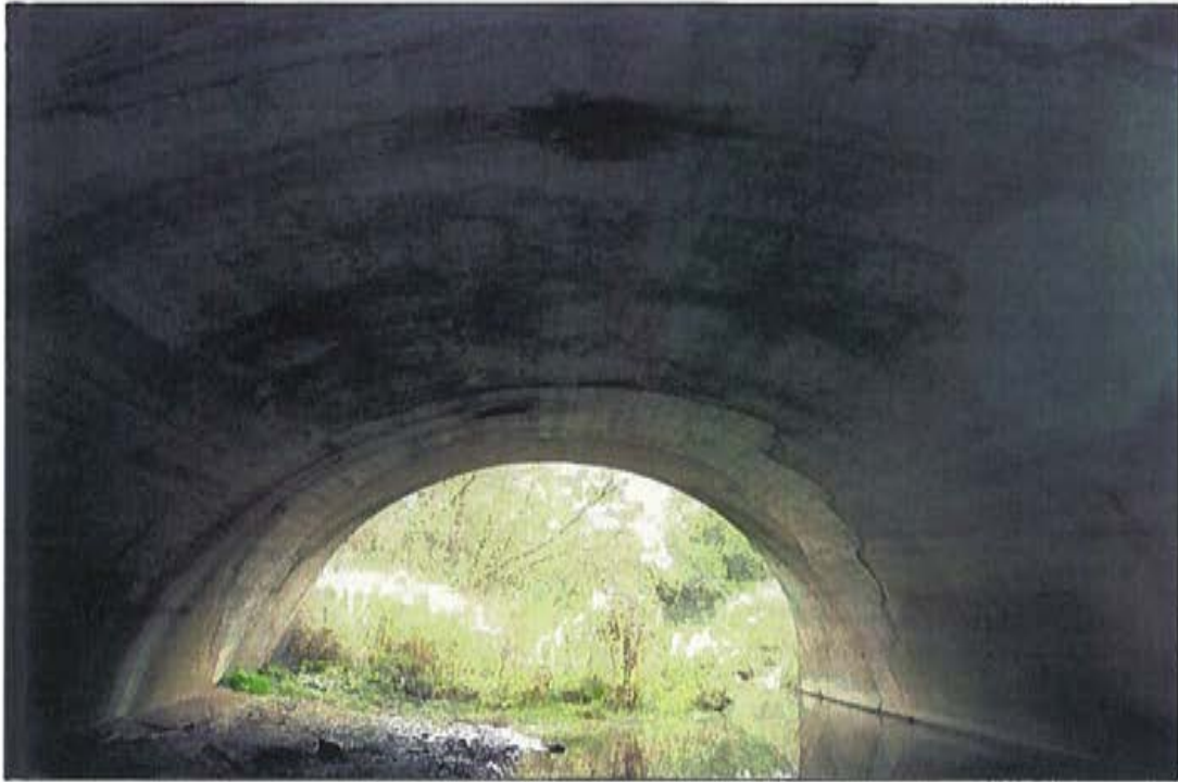
Photo 13: Culvert barrel, looking south.
