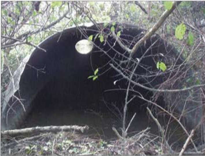
Photo 2g: Stn 2, culvert at north side of Mayfield rd. Nov 08, 2007.
