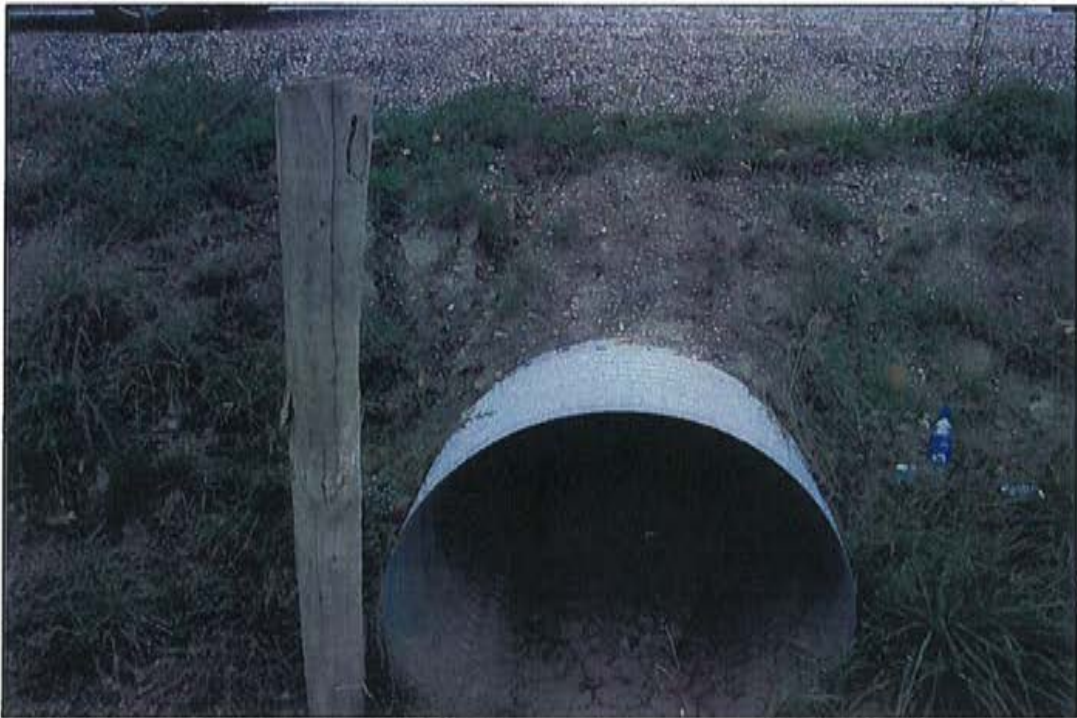
Photo 1: 15+249, outlet, looking north.
