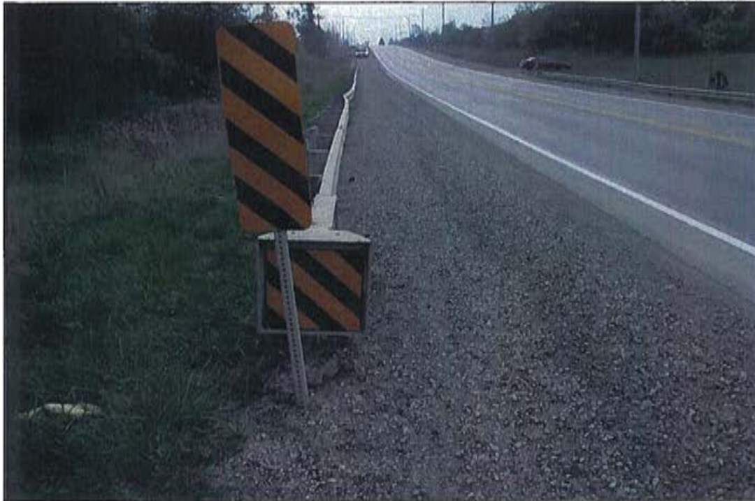
Photo 7: East approach, south side, looking west.
