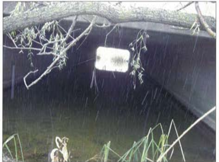
Photo 6e: Stn 6, looking from north (u-s) end of culvert downstream. Nov 08, 2007.
