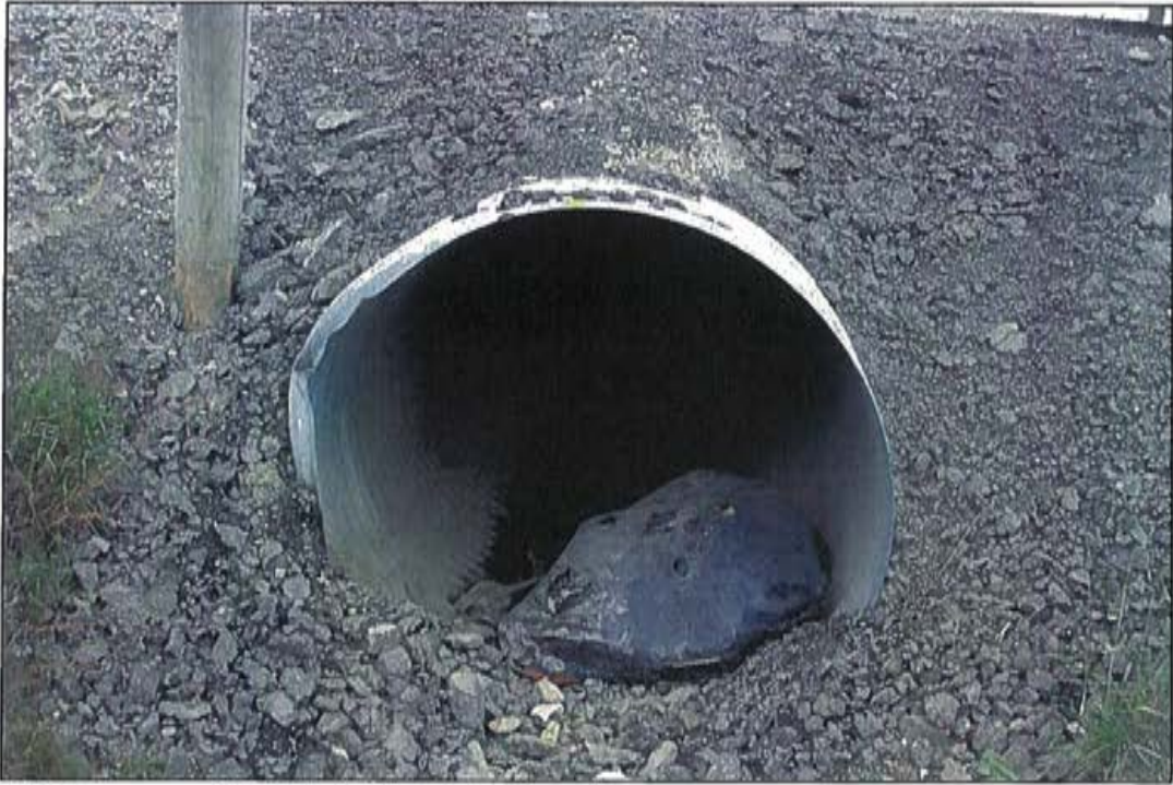
Photo 1: CSP at 10+425, outlet end, south.
