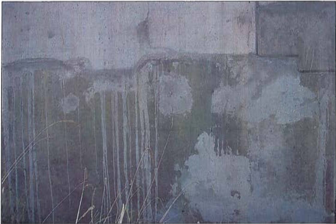
Photo 37: Wingwall, east approach, north side.
