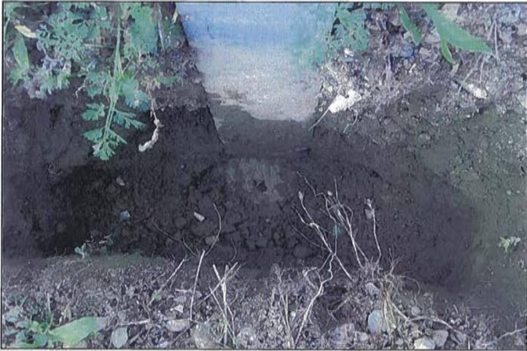
Photo 15: Post anchorage at concrete deck.
