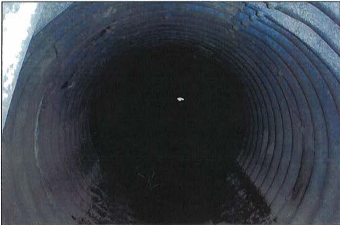
Photo 4: CSP, looking south.
