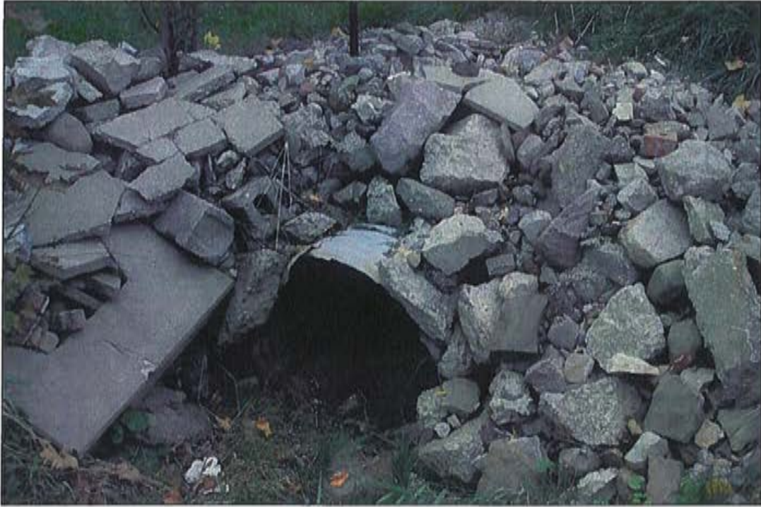
Photo 3: Inlet, looking south.
