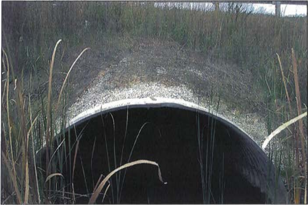
Photo 1: 10+689, outlet end, looking north.
