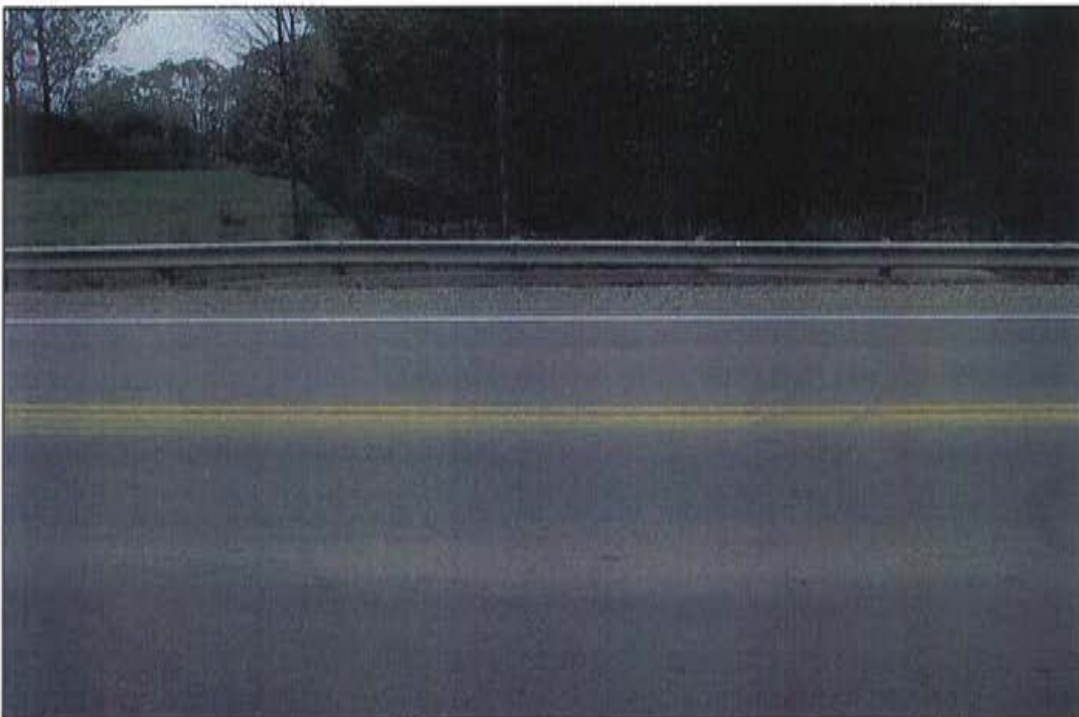
Photo 10: Steel beam guide rail with channel, north side.
