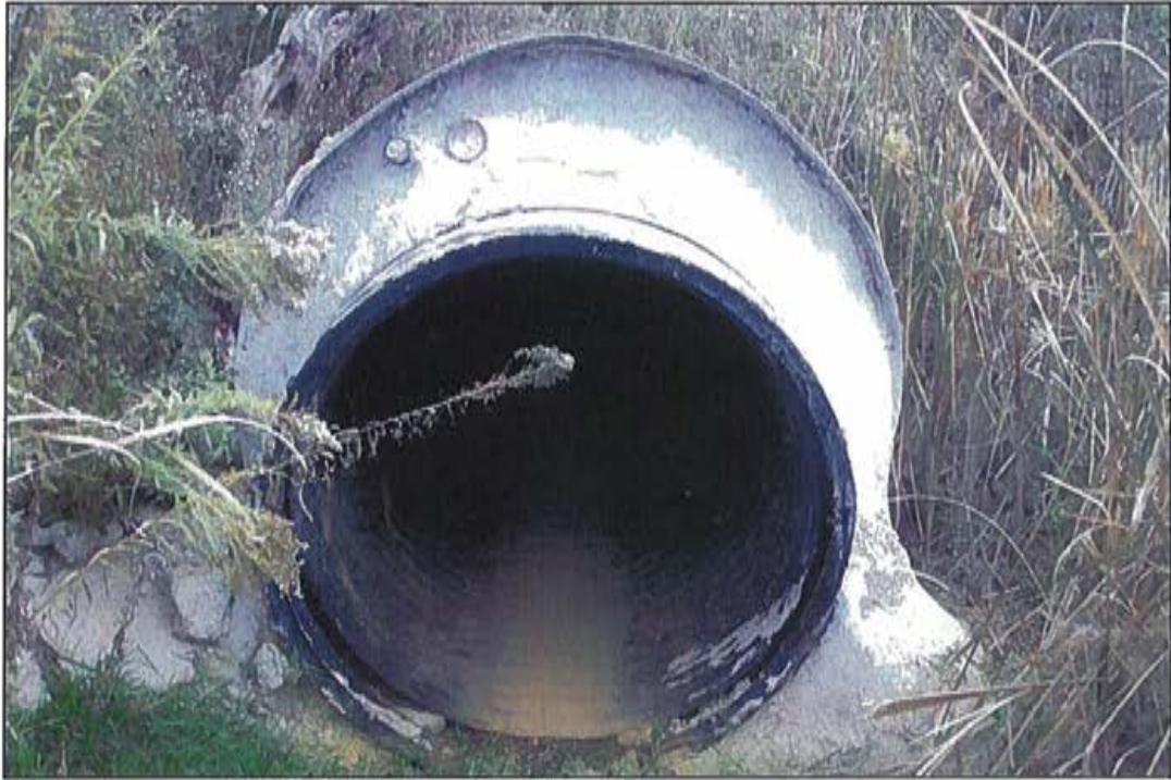
Photo 1: Sta. 14+177, inlet end, looking south.
