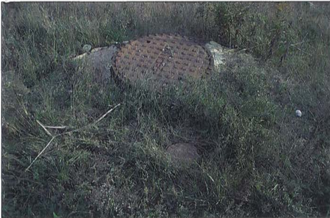
Photo 23: Water service, east approach, south side.
