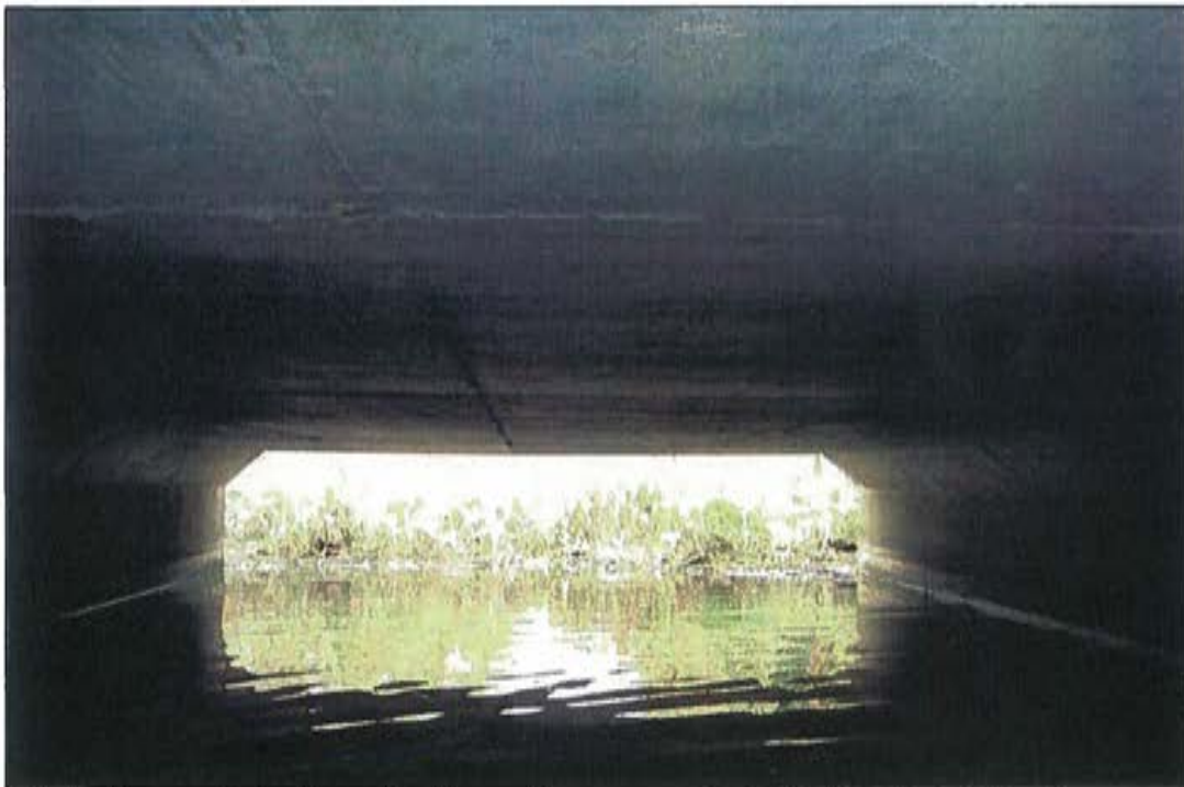
Photo 14: Culvert barrel, looking north.
