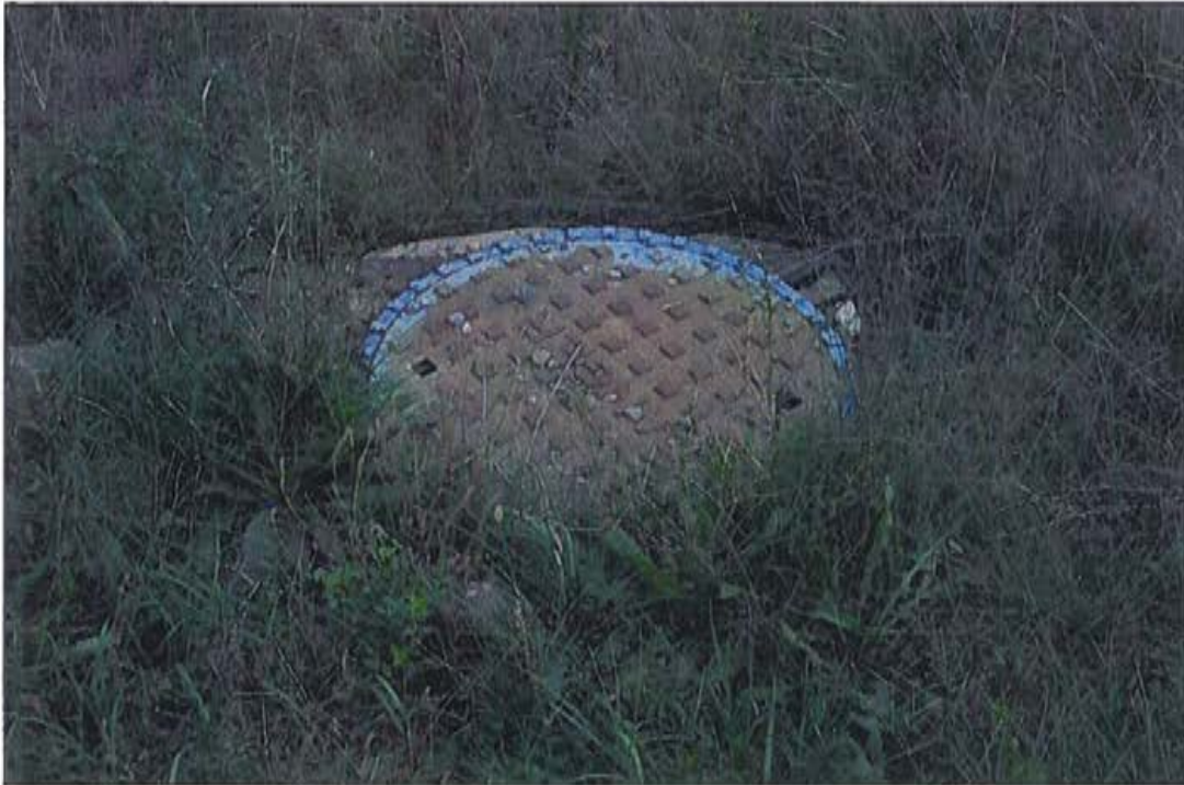
Photo 13: Manhole, west approach, south side.
