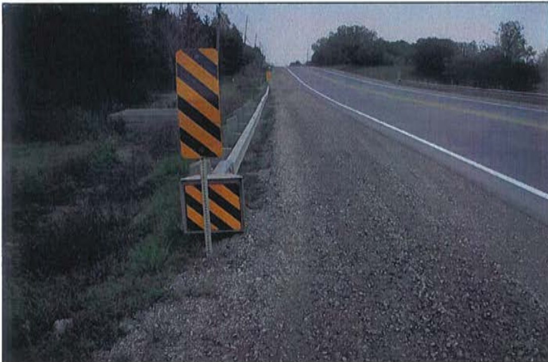
Photo 6: West approach, north side, looking east.
