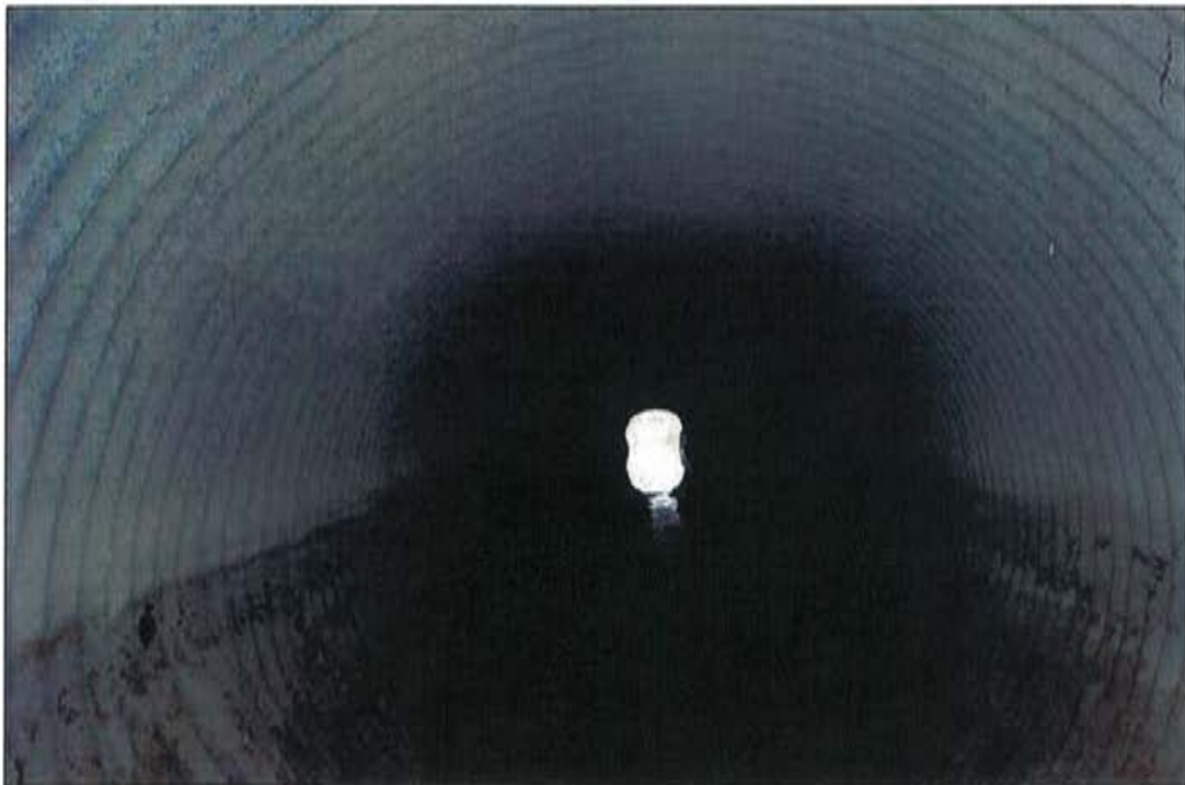
Photo 4: CSP, looking south.
