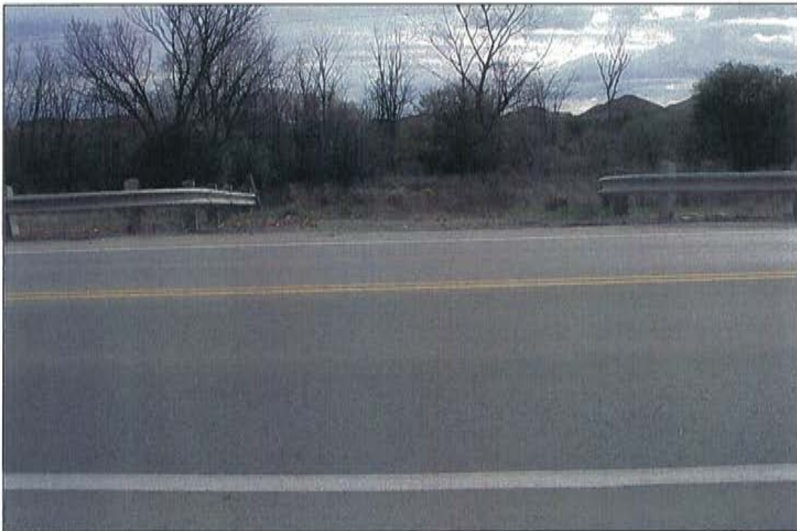
Photo 24: Field entrance, west approach, south side.
