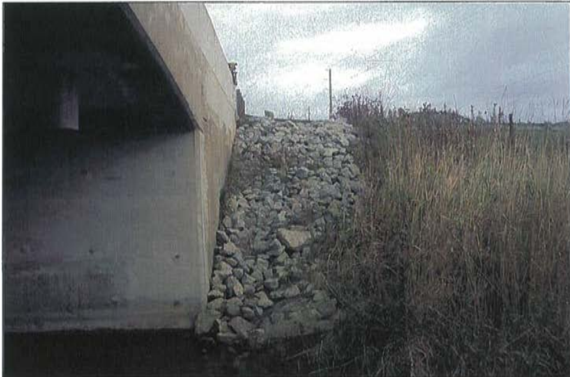
Photo 34: Embankment, east approach, south side.
