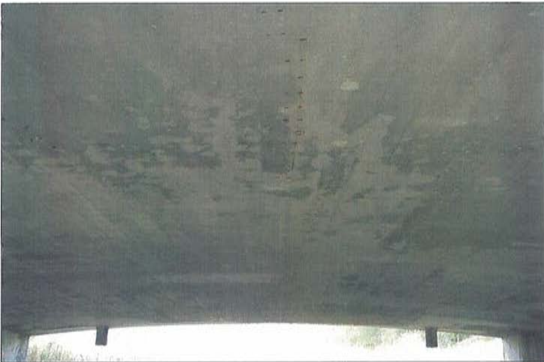
Photo 26: Underside of deck, looking north.
