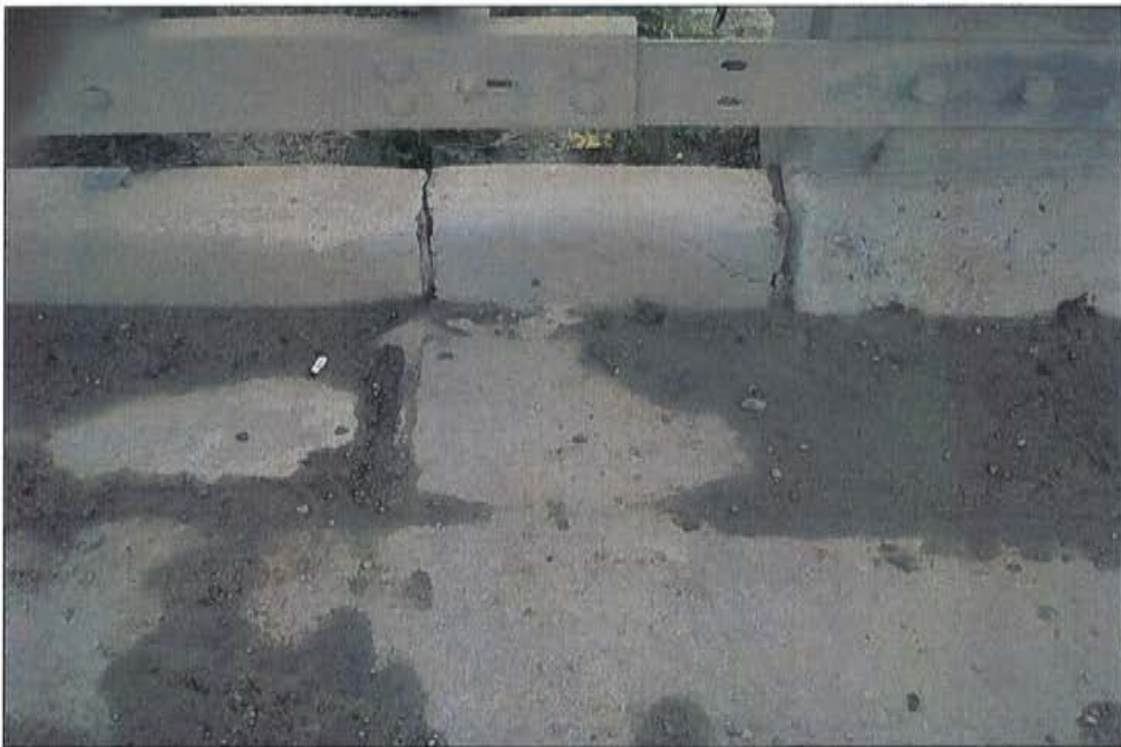
Photo 12: Curb, east approach, south side.
