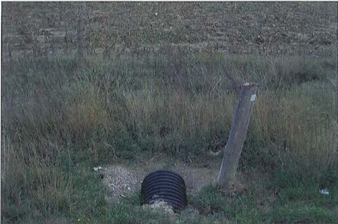
Photo 2: Outlet end, looking south.
