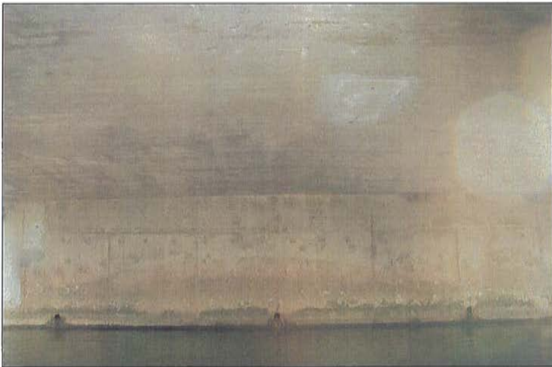
Photo 28: West abutment wall.
