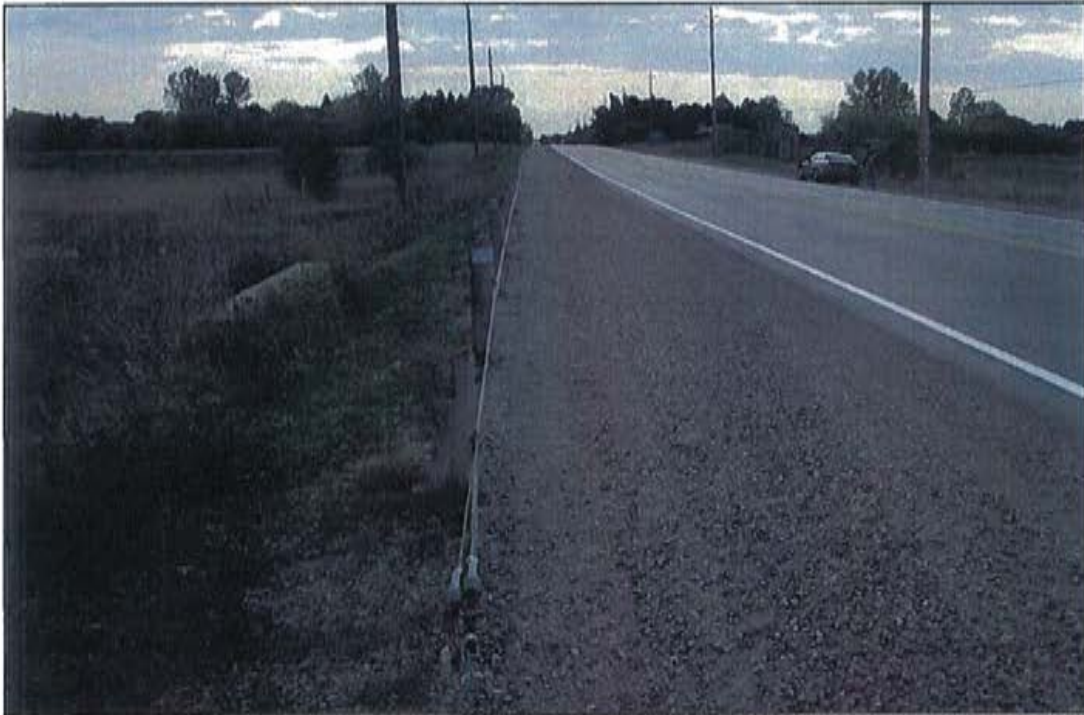
Photo 18: East approach, south side.
