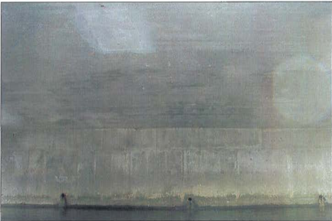
Photo 30: East abutment wall.
