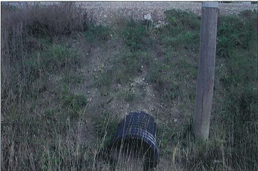
Photo 4: Culvert inlet, looking south.
