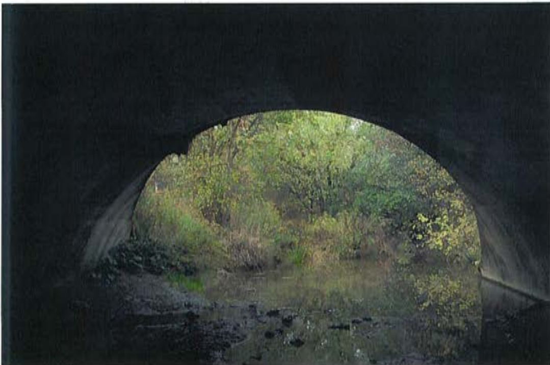
Photo 12: Site 14380, looking north, upstream.
