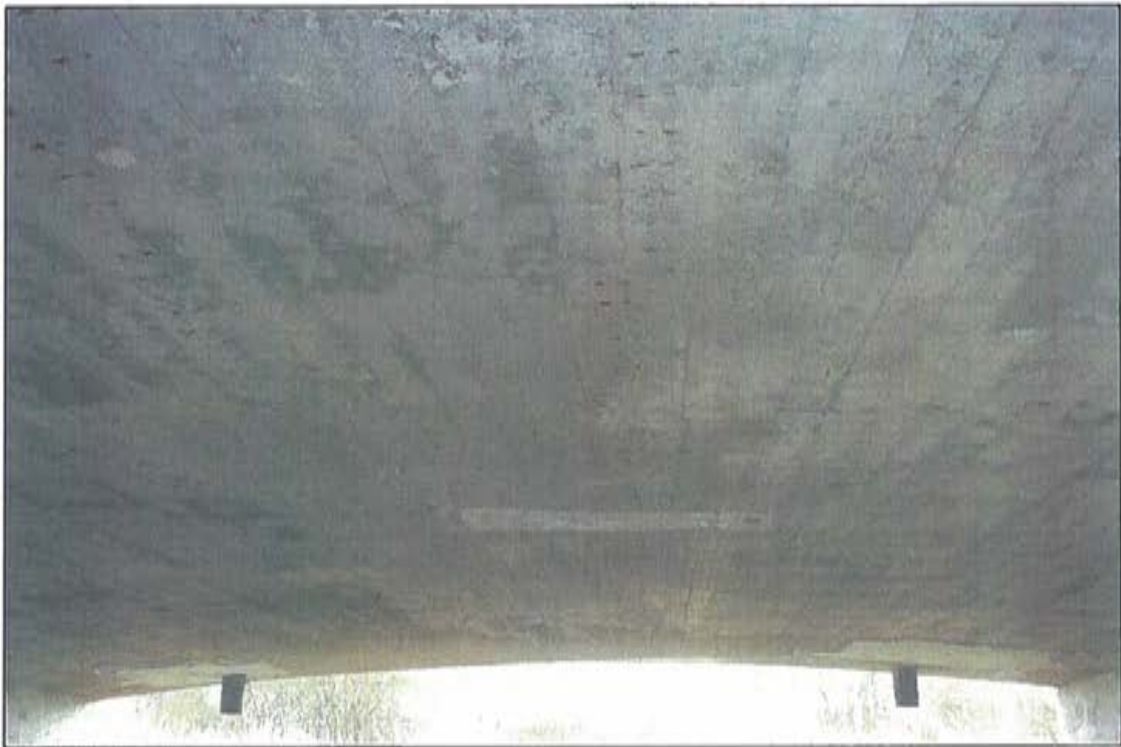
Photo 25: Underside of deck, looking south.
