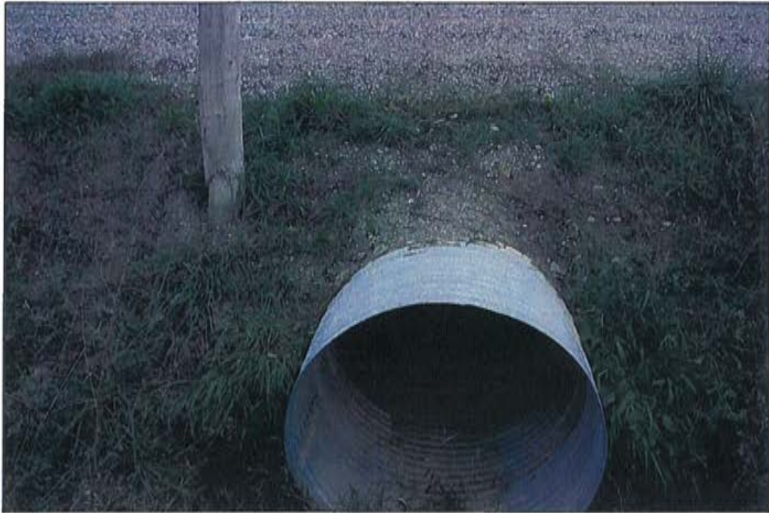
Photo 3: Inlet end, looking south.
