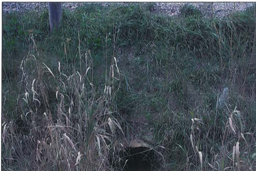
Photo 1: 15+693, outlet, looking north.
