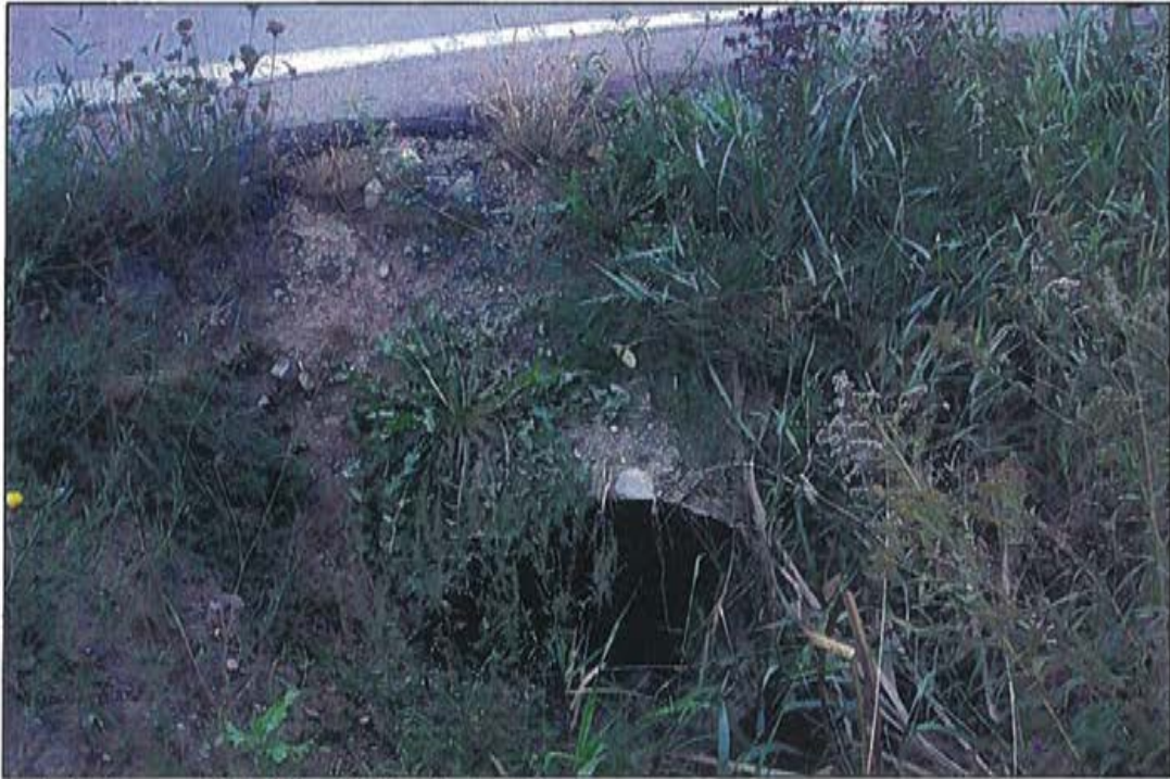
Photo 1: 14+567 outlet, looking east.
