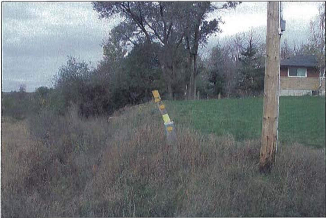
Photo 19: Bell service, east approach, north side.
