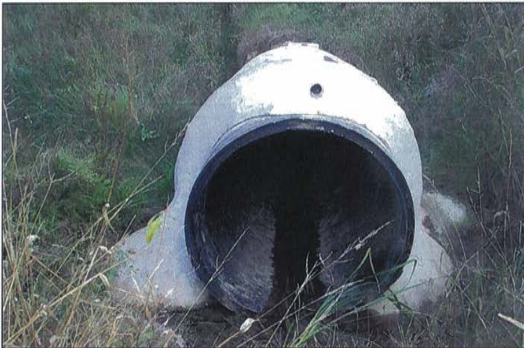
Photo 4: Inlet end, looking south: liner.
