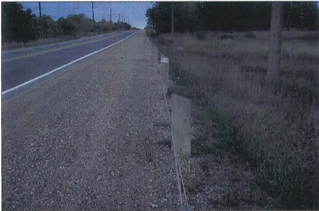
Photo 6: West approach, south side, looking east.
