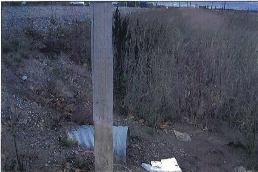
Photo 2: Outlet, looking east.
