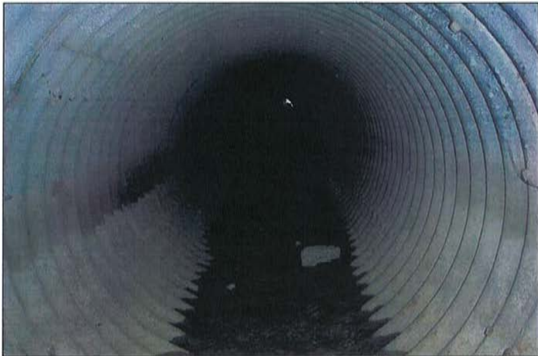
Photo 2: Culvert, looking east.
