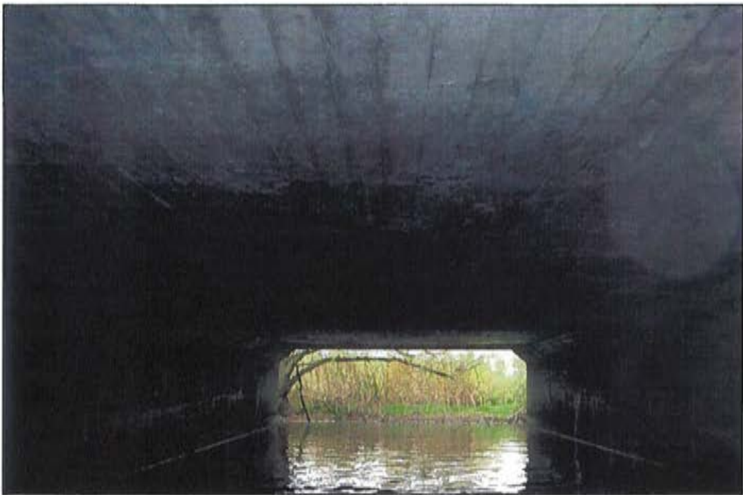
Photo 12: Culvert barrel, looking south.
