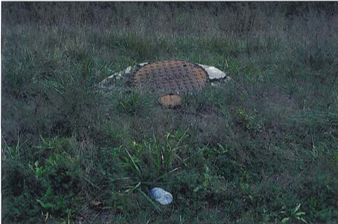
Photo 10: Water service, south side, east approach.
