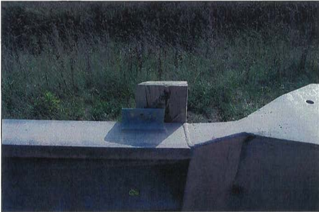
Photo 9: Eccentric loader connection, west approach, south side.
