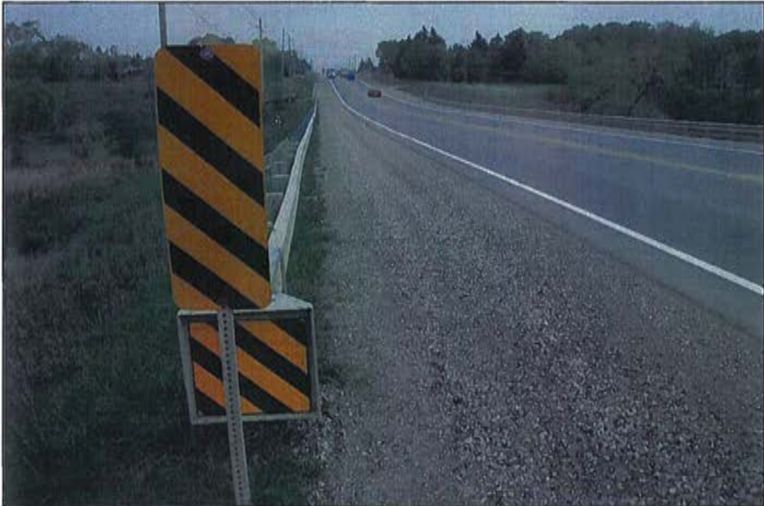
Photo 7: West approach, north side.
