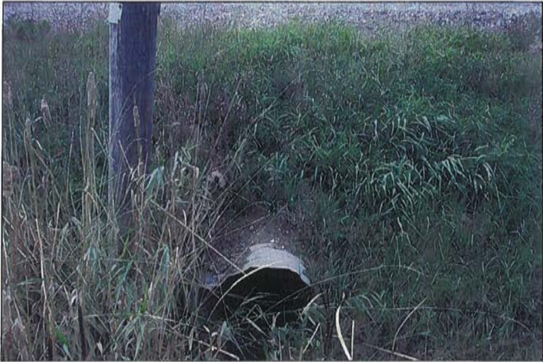
Photo 1: 15+454, outlet, looking north.
