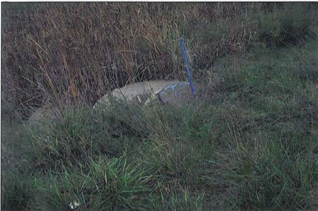
Photo 12: Water service, east approach, south side.
