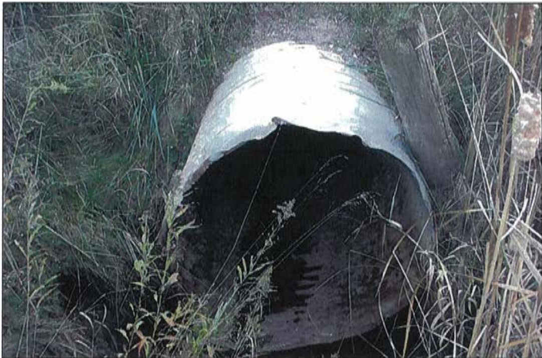
Photo 2: Inlet end, looking south.
