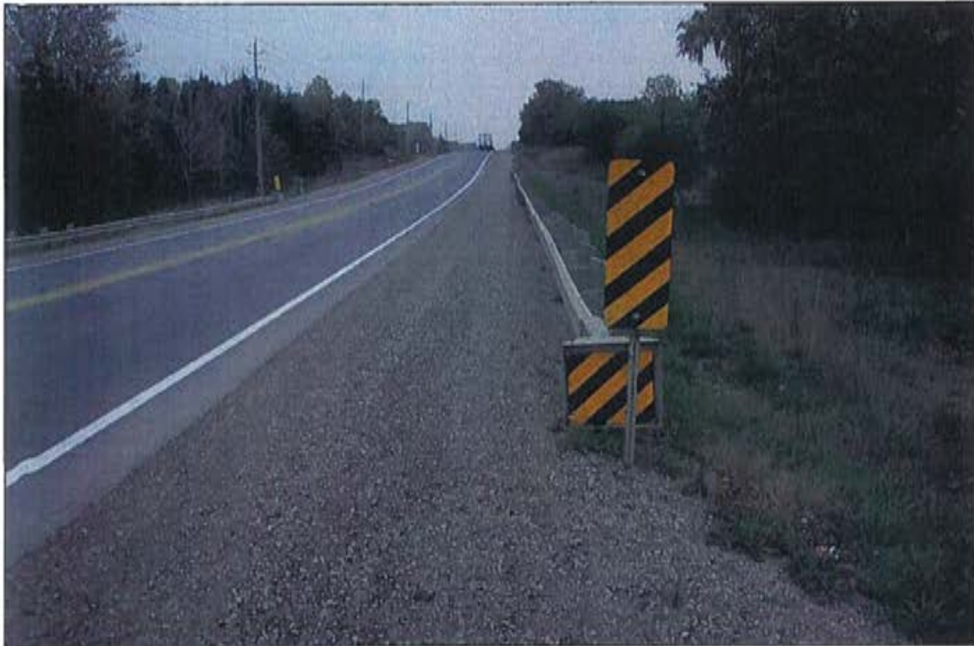
Photo 5: West approach, south side, looking east.
