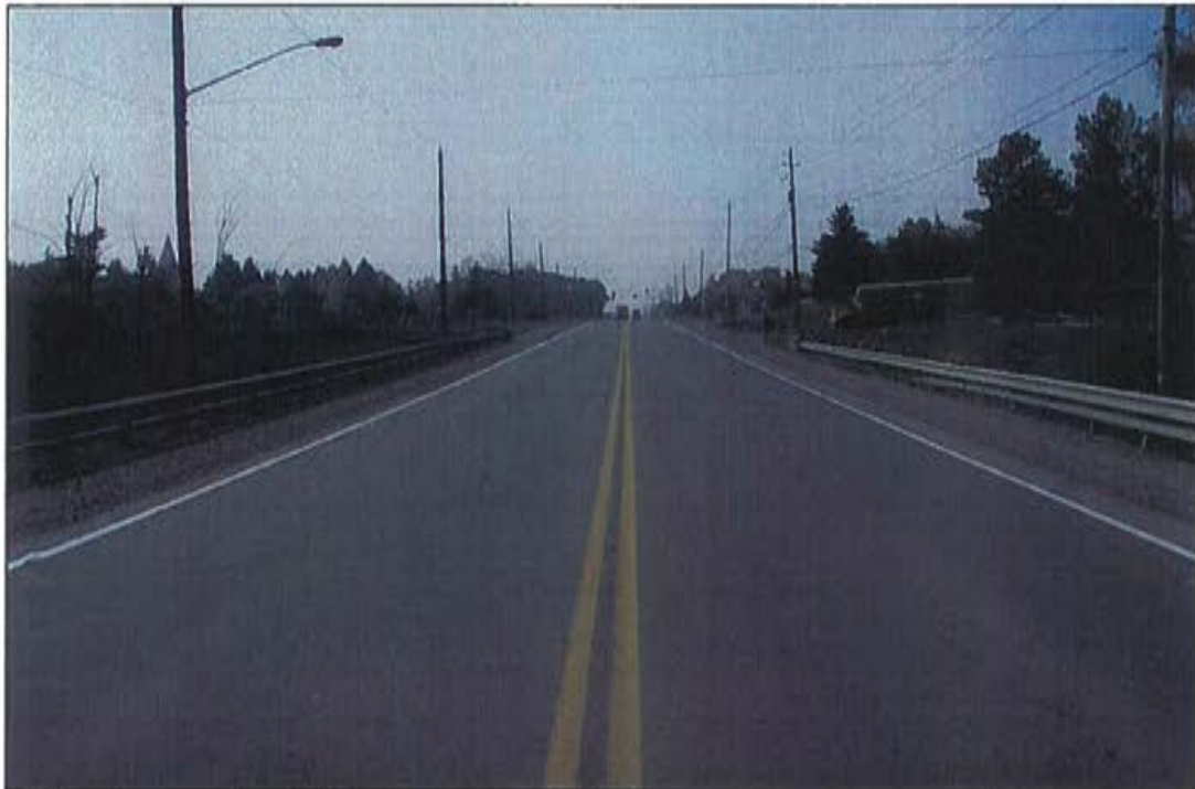
Photo 2: Mayfield Road, general view, looking west.
