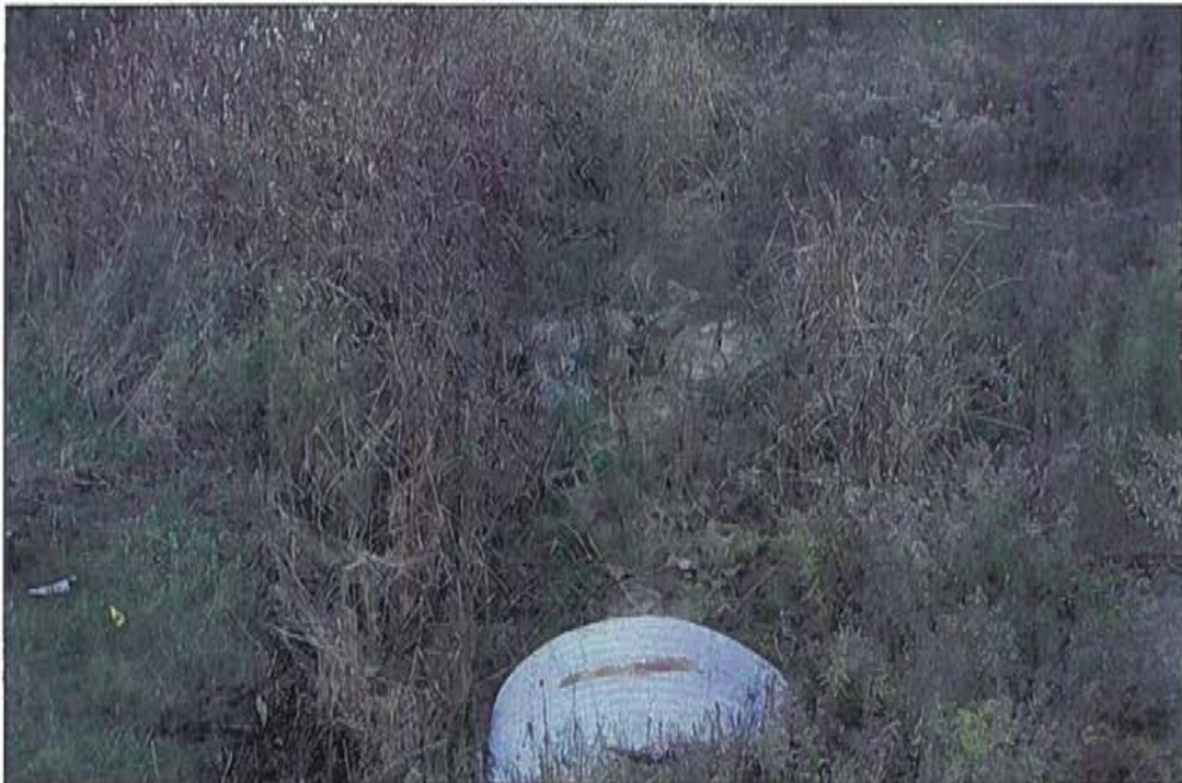
Photo 2: Culvert inlet, looking north.
