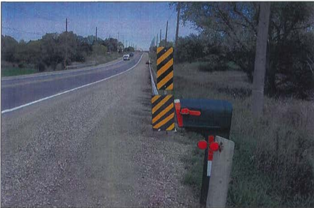
Photo 12: West approach, south side.
