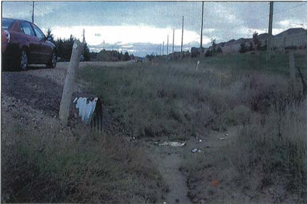
Photo 4: CSP 1, south side, looking east.
