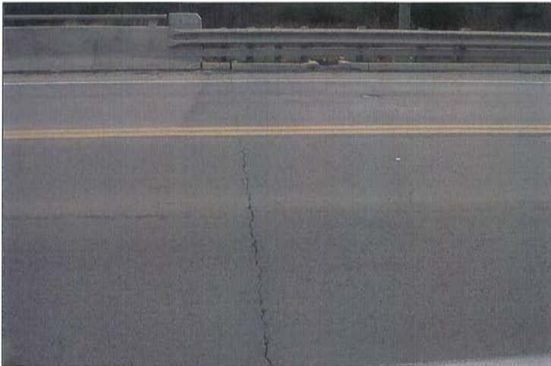
Photo 16: Approach wearing surface, east abutment, looking south.
