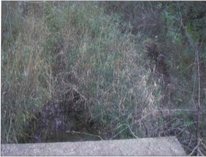
Photo 5e: Stn 5, facing south (d-s) Mayfield rd culvert. Nov 08, 2007.
