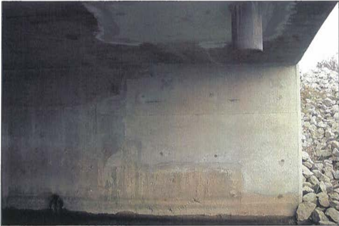
Photo 31: Abutment wall, east approach, south side.
