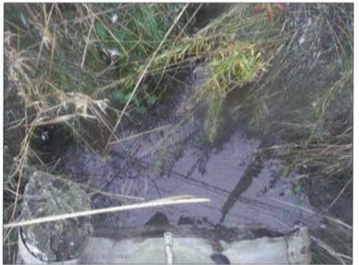
Photo 8b: Stn 8, water at north culvert. Nov 08, 2007.
