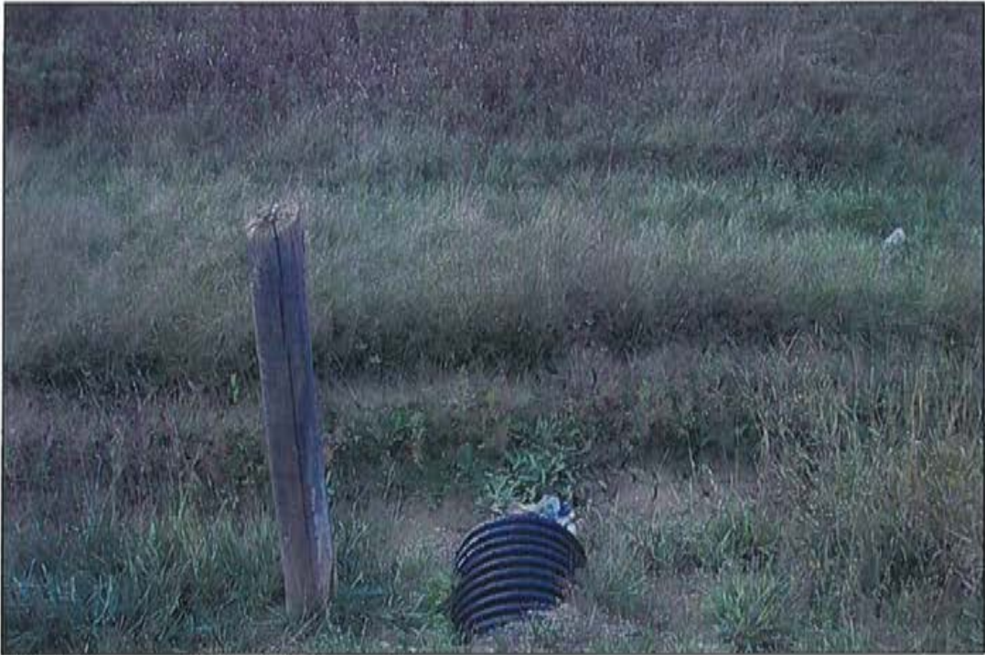
Photo 3: Inlet end, looking north.
