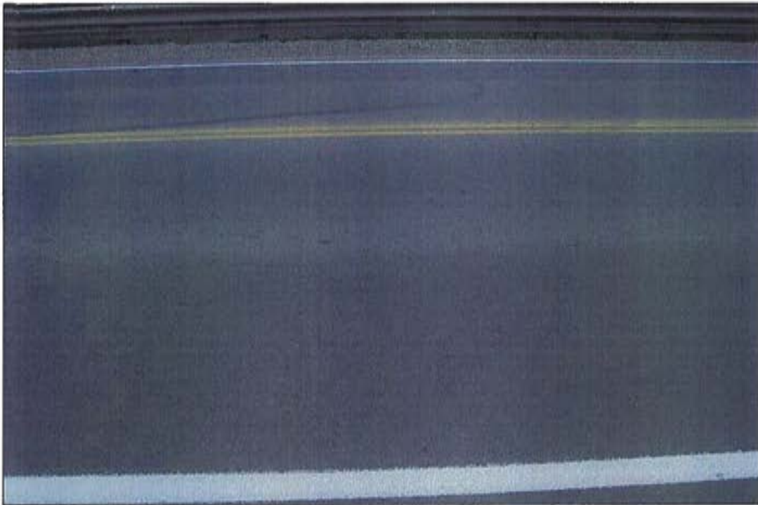
Photo 9: Wearing surface, looking south.
