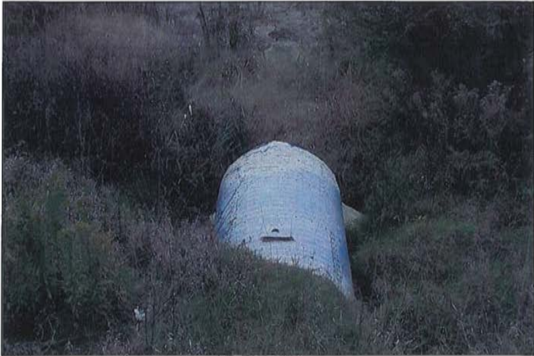
Photo 3: Outlet end, looking north.
