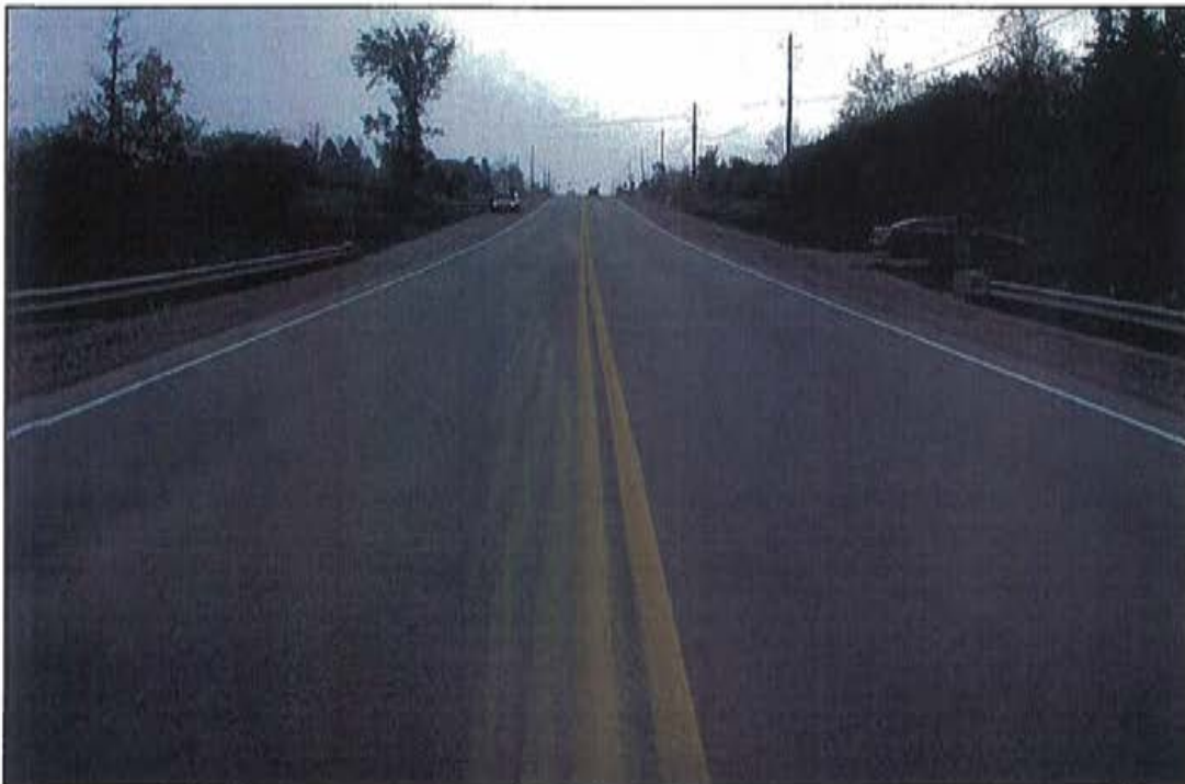
Photo 2: Mayfield Road, general view, looking west.
