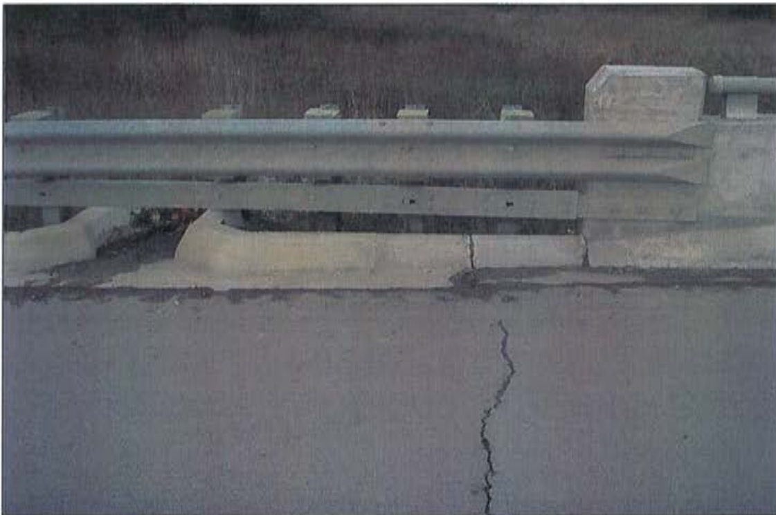
Photo 6: Steel beam guide rail connection, west approach, north side.
