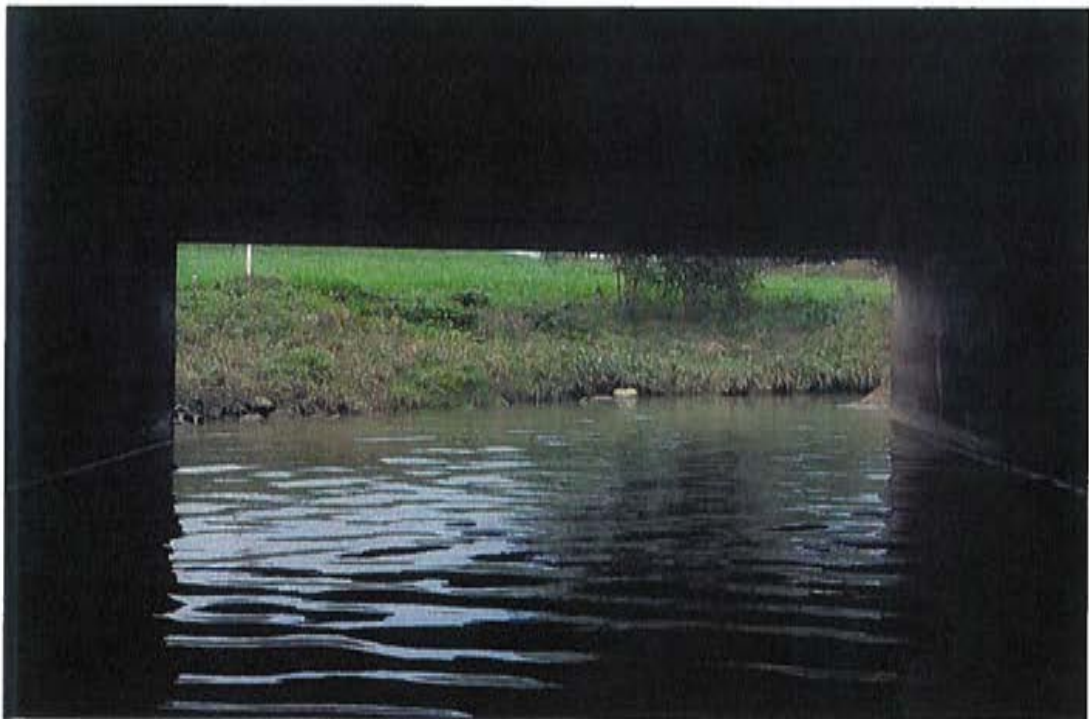
Photo 18: Culvert barrel, looking north.
