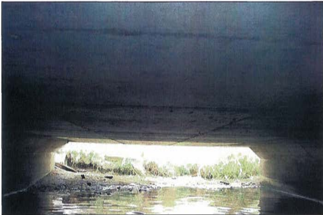
Photo 15: Culvert barrel, looking south.
