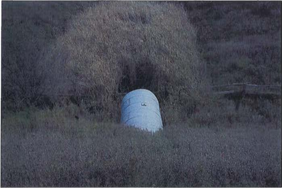
Photo 1: CSP 12+504, outlet end, looking south.
