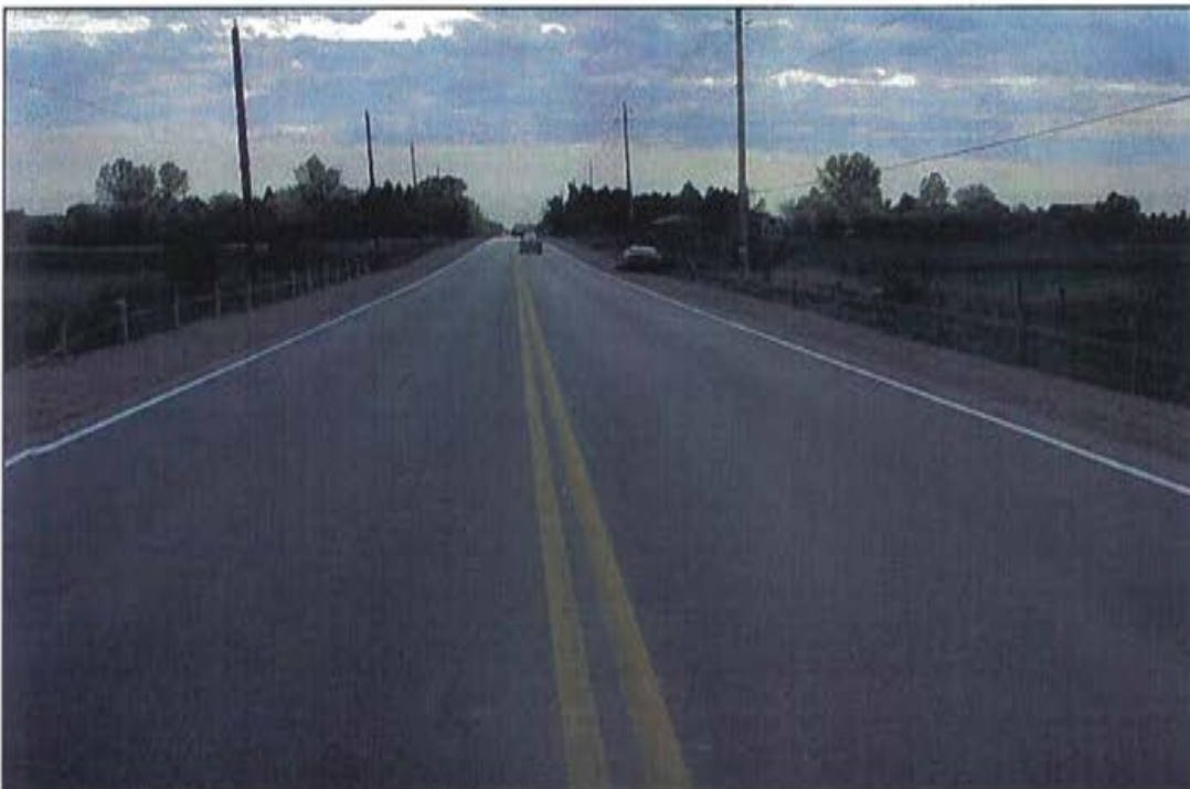
Photo 2: Mayfield Road, general view, looking west.
