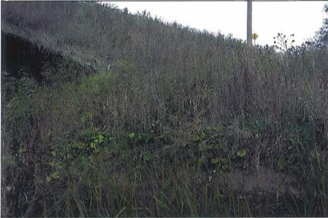
Photo 21: Embankment, southeast corner.
