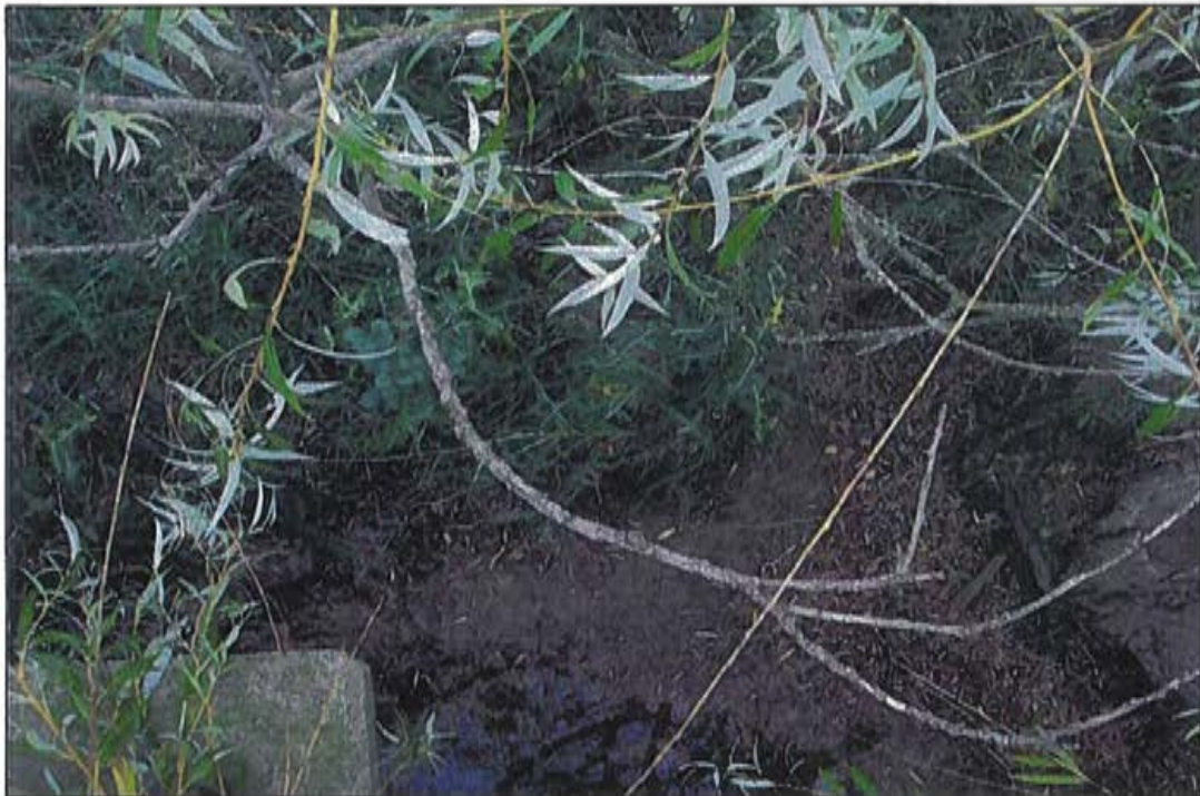
Photo 20: Embankment, east approach, south side.
