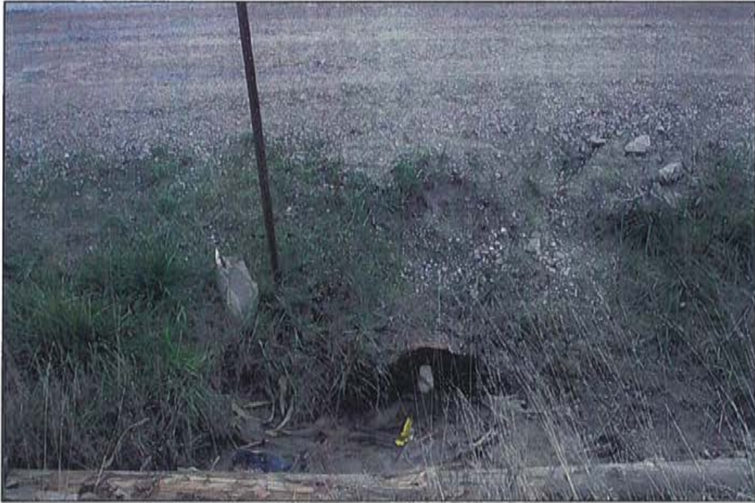
Photo 3: Culvert, looking north
