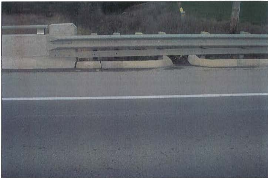
Photo 10: East approach, north side, steel beam guide rail connection.
