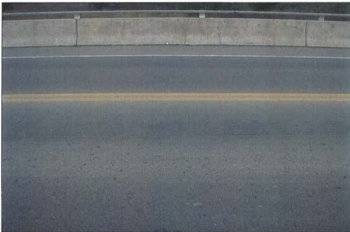
Photo 14: Wearing surface, deck, looking north.
