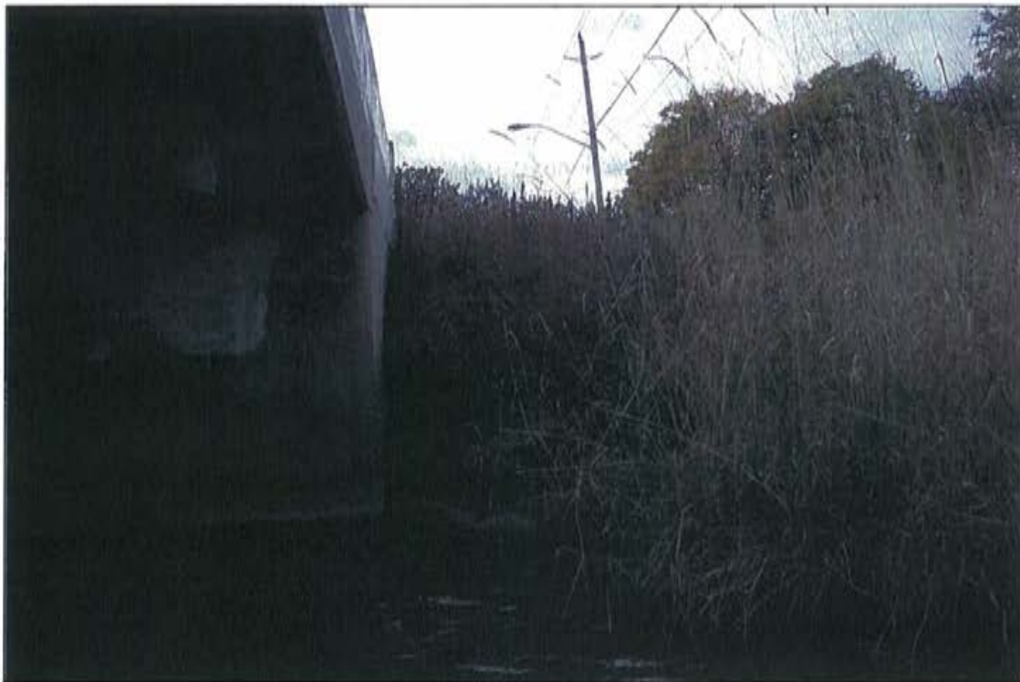
Photo 35: Embankment, west approach, north side.
