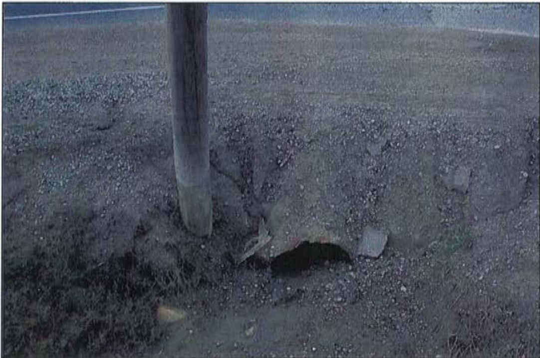
Photo 2: Outlet, looking north
