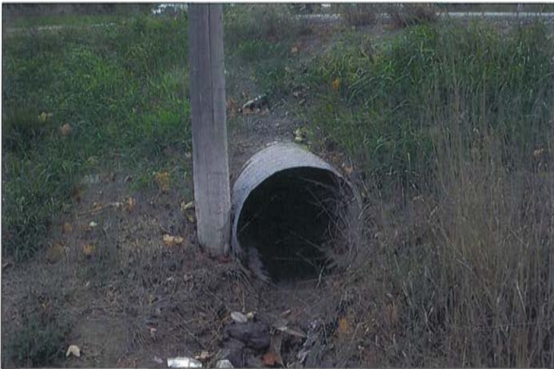
Photo 6: Degor Road, south of Mayfield, looking west.
