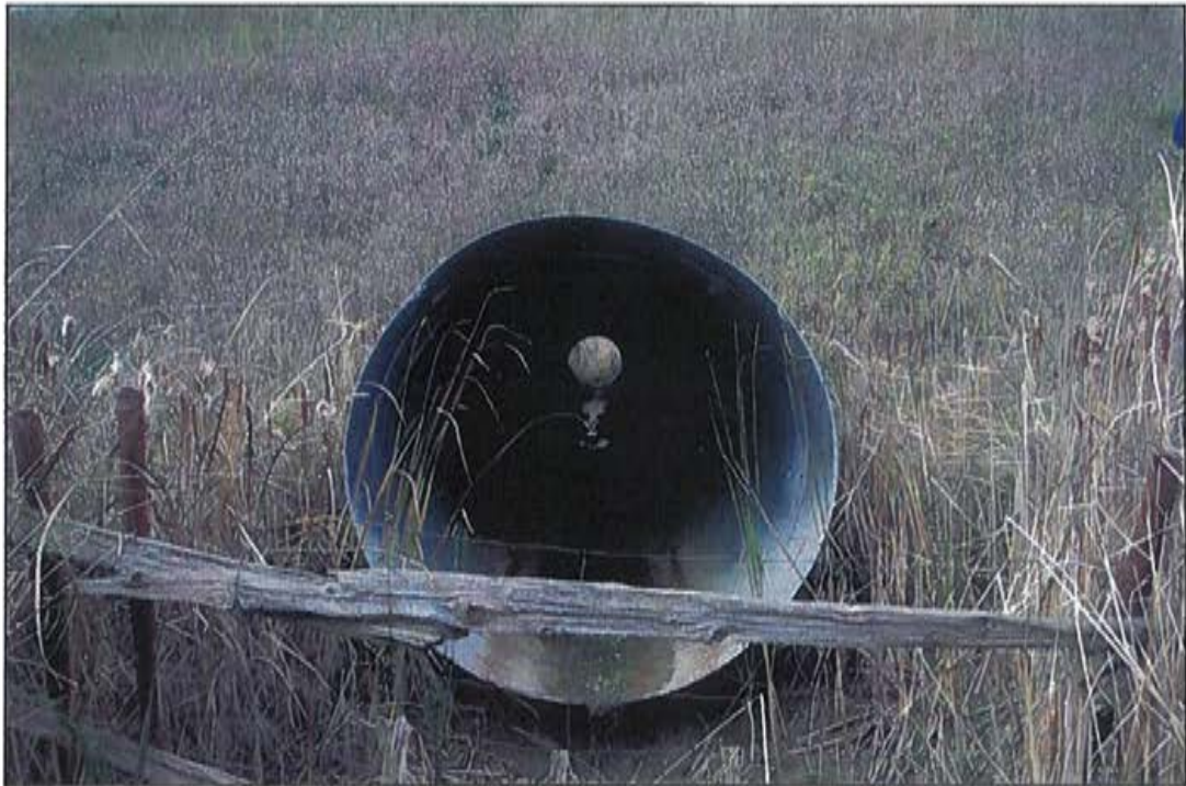
Photo 2: Outlet end, looking north.
