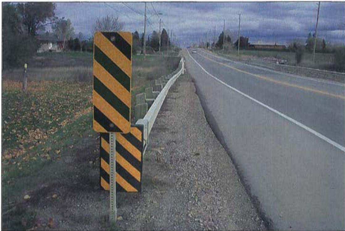
Photo 17: West approach, north side, looking east.
