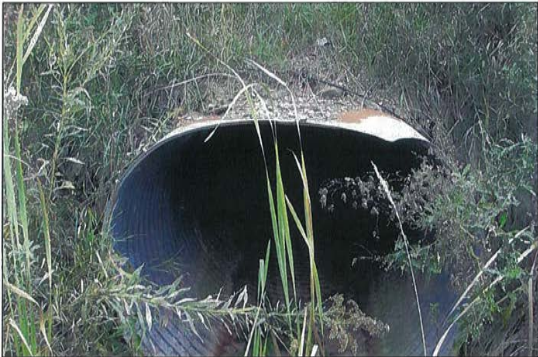
Photo 4: Inlet end, looking south.
