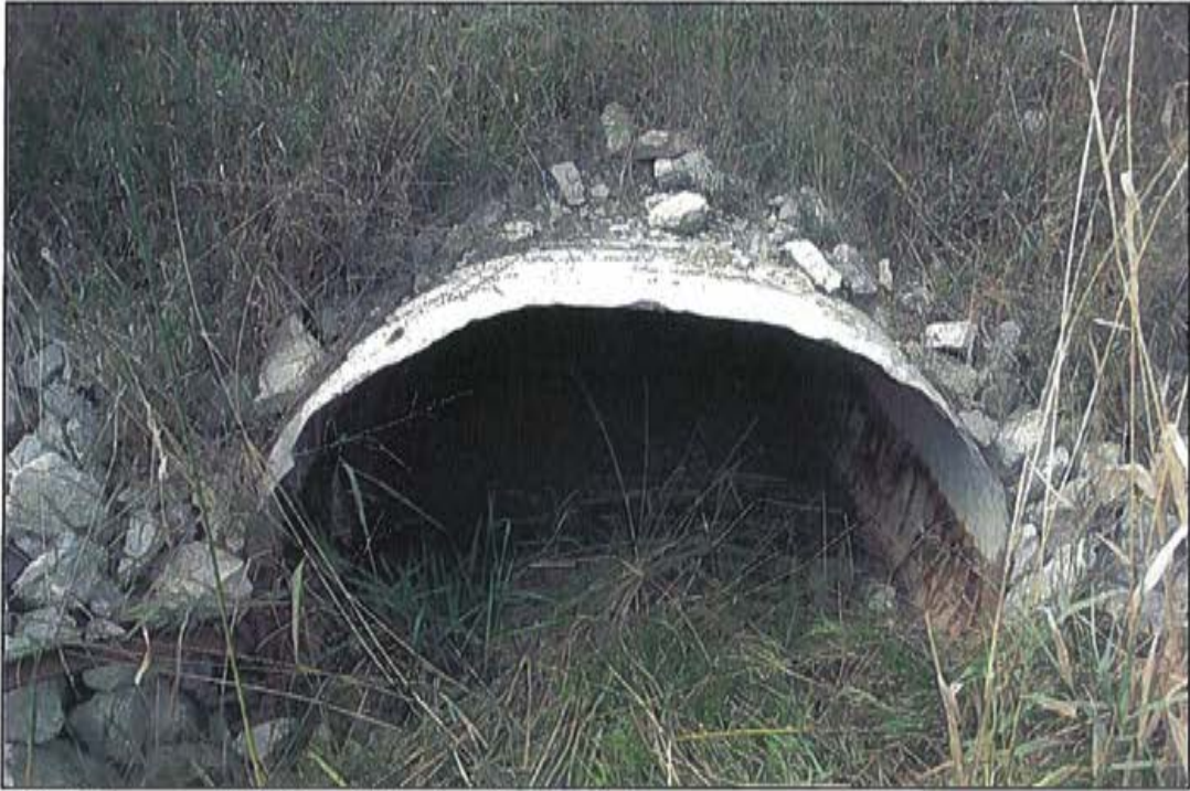
Photo 1: 11+603, outlet end, looking north.
