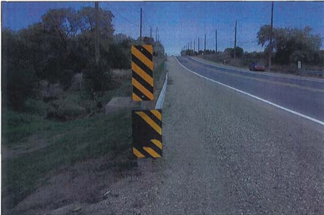
Photo 11: West approach, north side.
