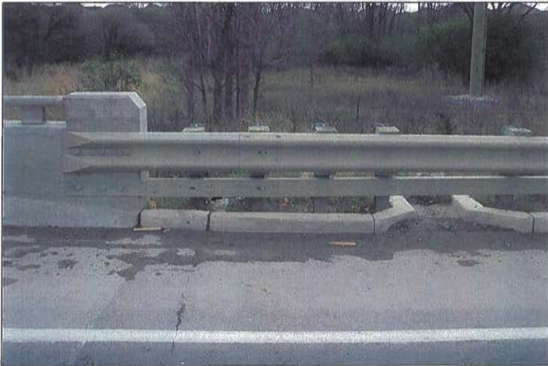
Photo 5: West approach, south side, steel beam guide rail connection.
