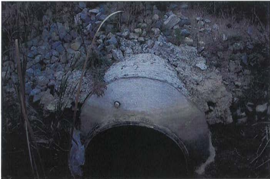
Photo 4: Culvert outlet, looking north.
