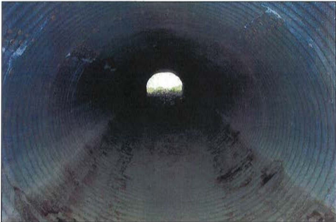
Photo 6: CSP, looking south (downstream).
