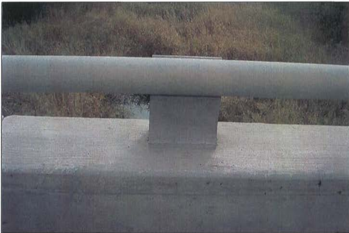
Photo 8: Steel rail and post.
