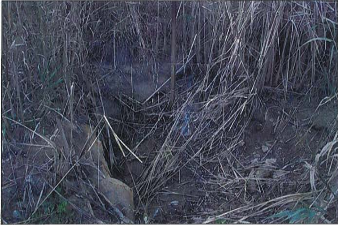
Photo 1: 15+885, outlet, looking east.
