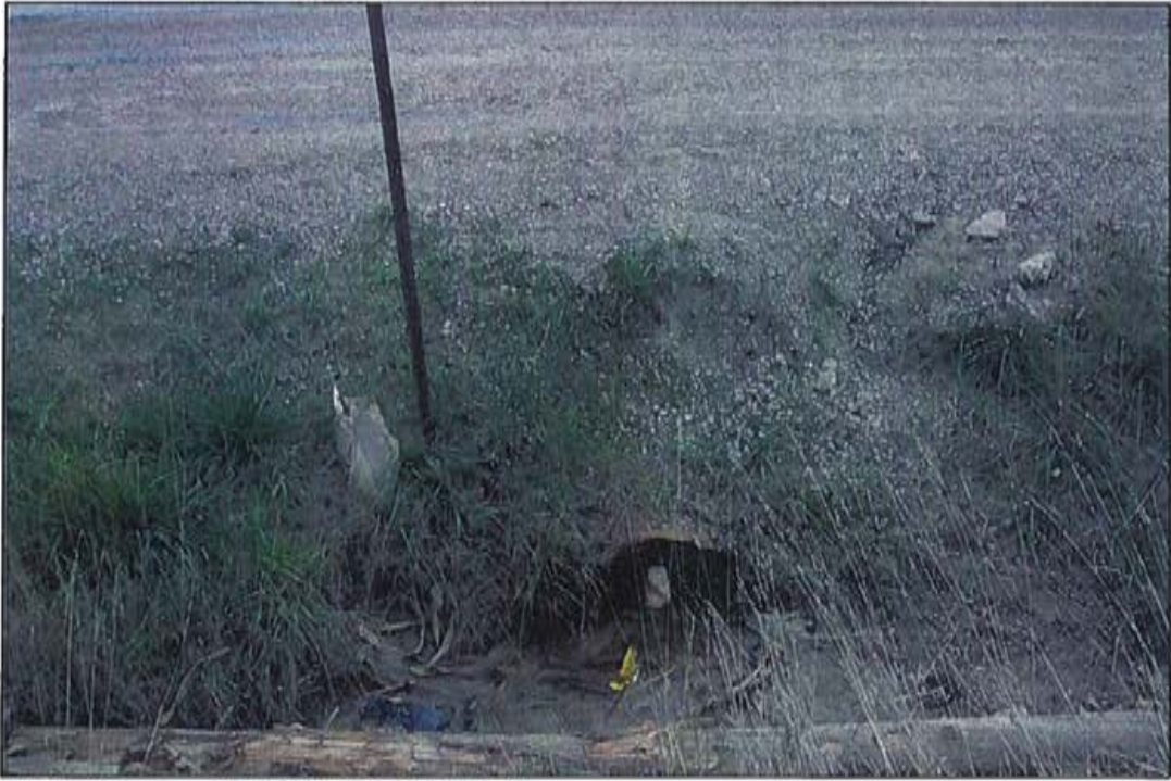
Photo 1: 16+842 inlet, looking south
