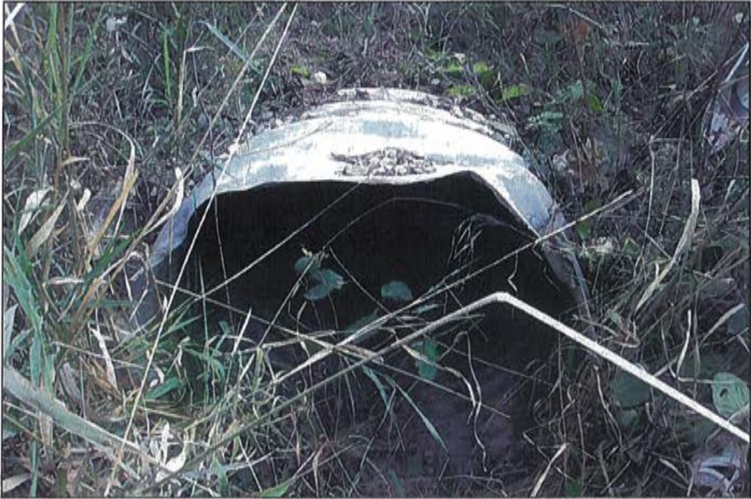
Photo 3: Inlet end, looking south.
