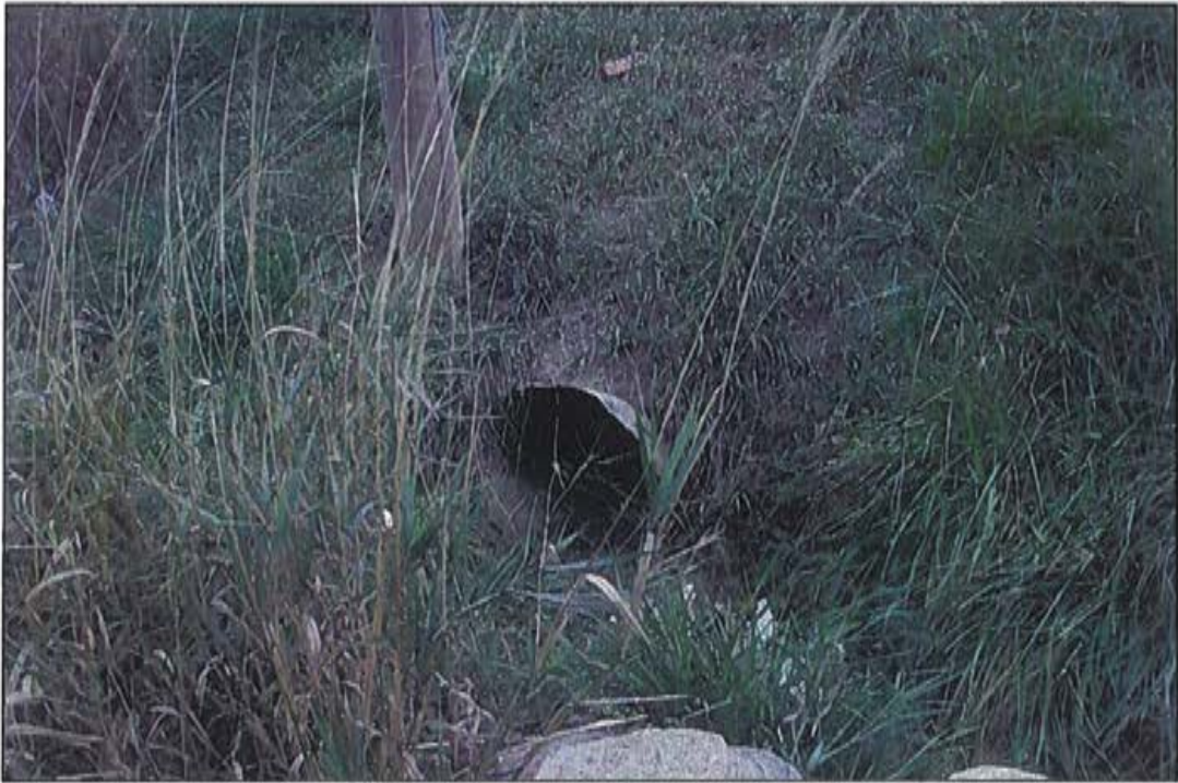
Photo 3: Inlet end, looking south.
