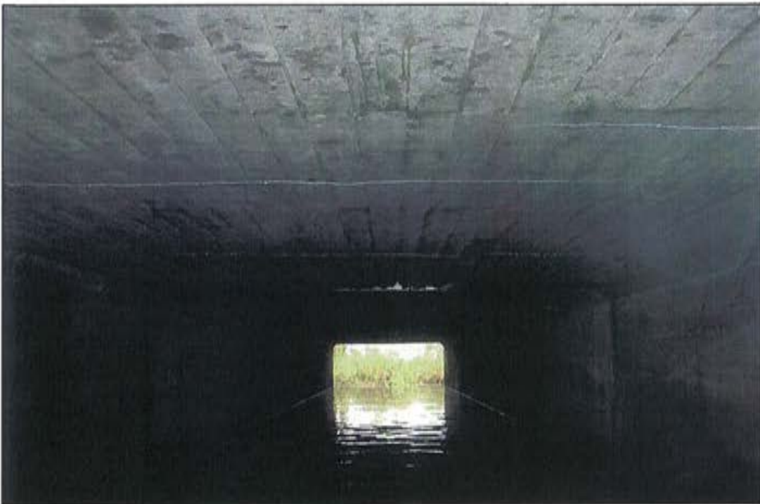
Photo 14: Culvert barrel, looking south.
