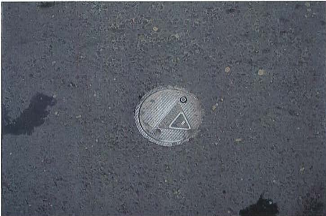
Photo 22: Observation monitoring well, east approach, south.
