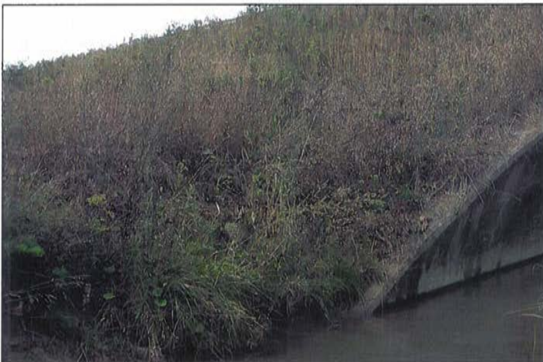
Photo 20: Embankment, southwest corner.
