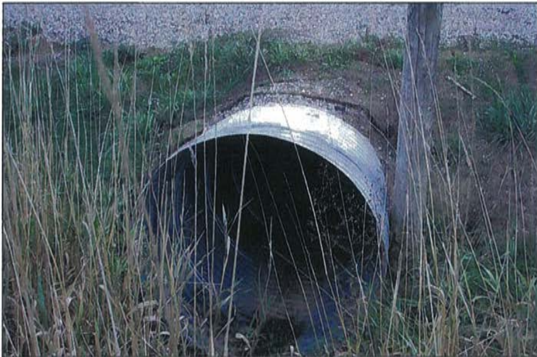
Photo 2: CSP, looking south.
