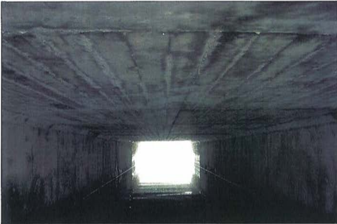
Photo 13: Culvert barrel, looking north.
