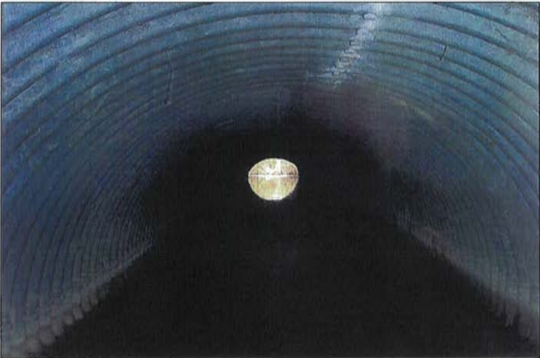
Photo 2: Culvert, looking south.
