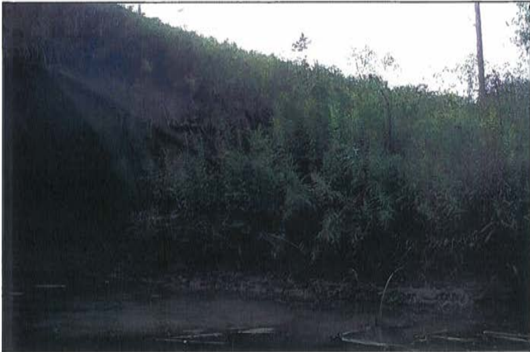
Photo 23: Embankment, northwest corner.
