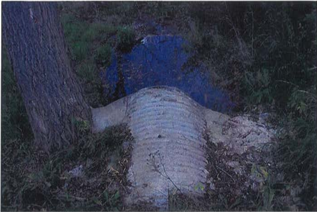
Photo 1: 13+970, outlet end, looking south.
