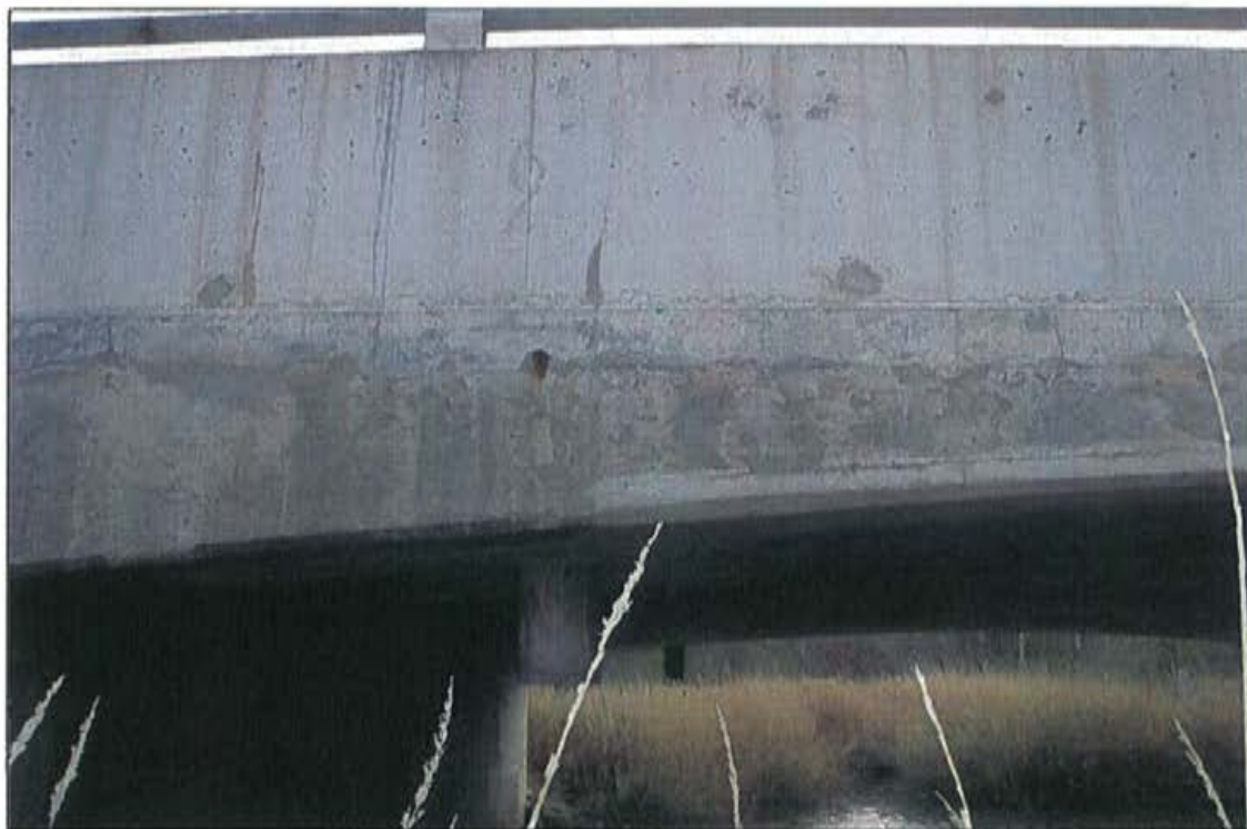
Photo 36: Deck barrier exterior, north side, looking south.
