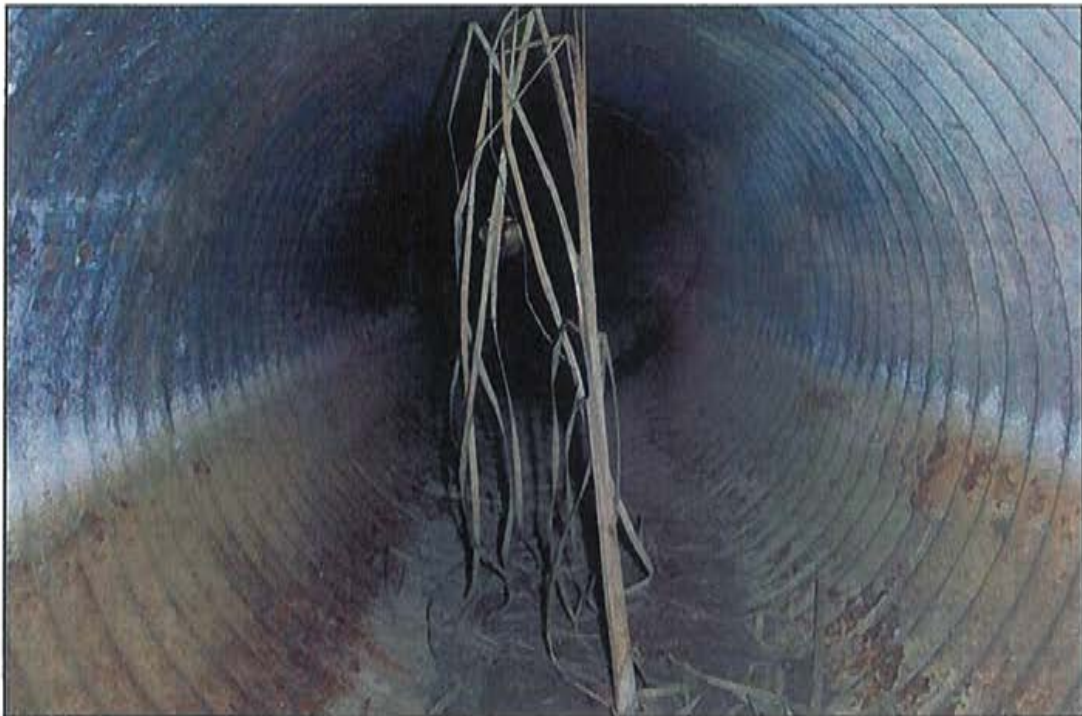
Photo 2: Outlet, looking north.
