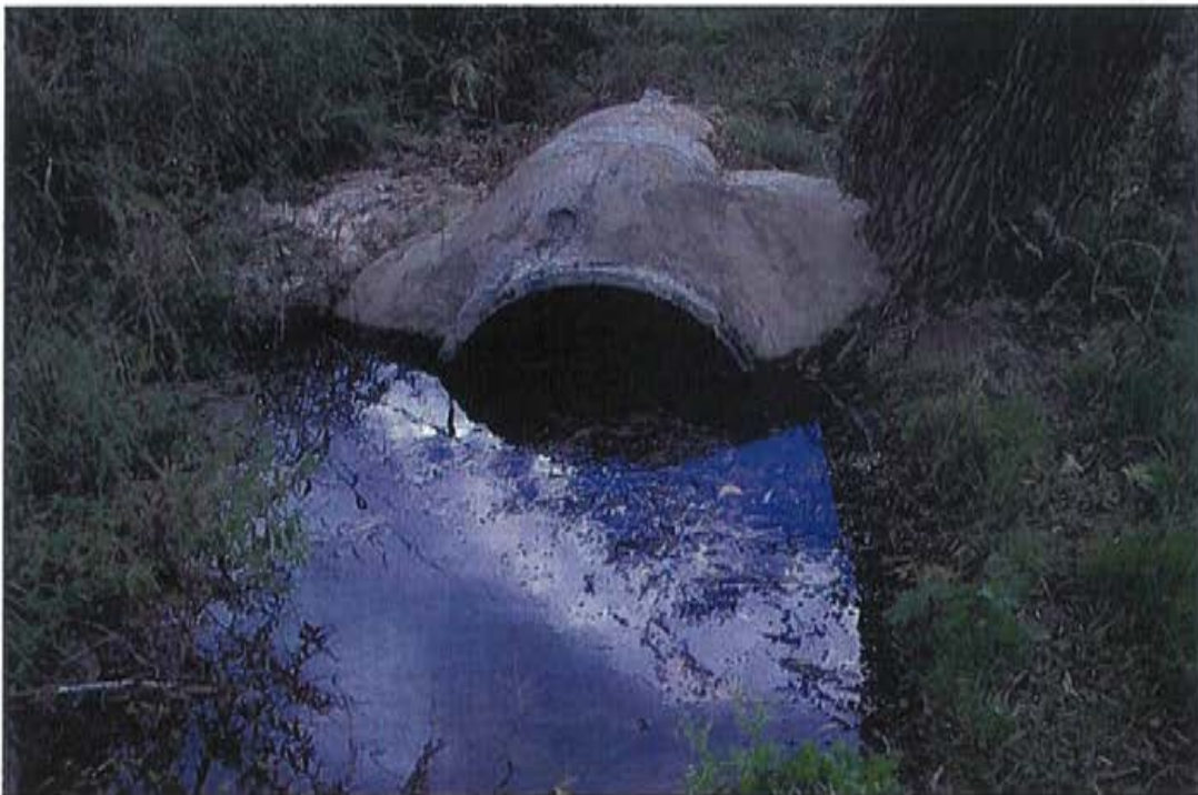
Photo 2: Outlet end, looking north: liner.
