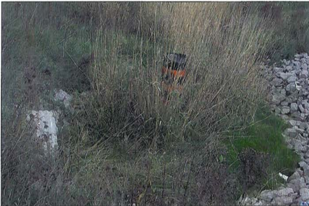
Photo 8: CSP, south side, looking east: rock protection.
