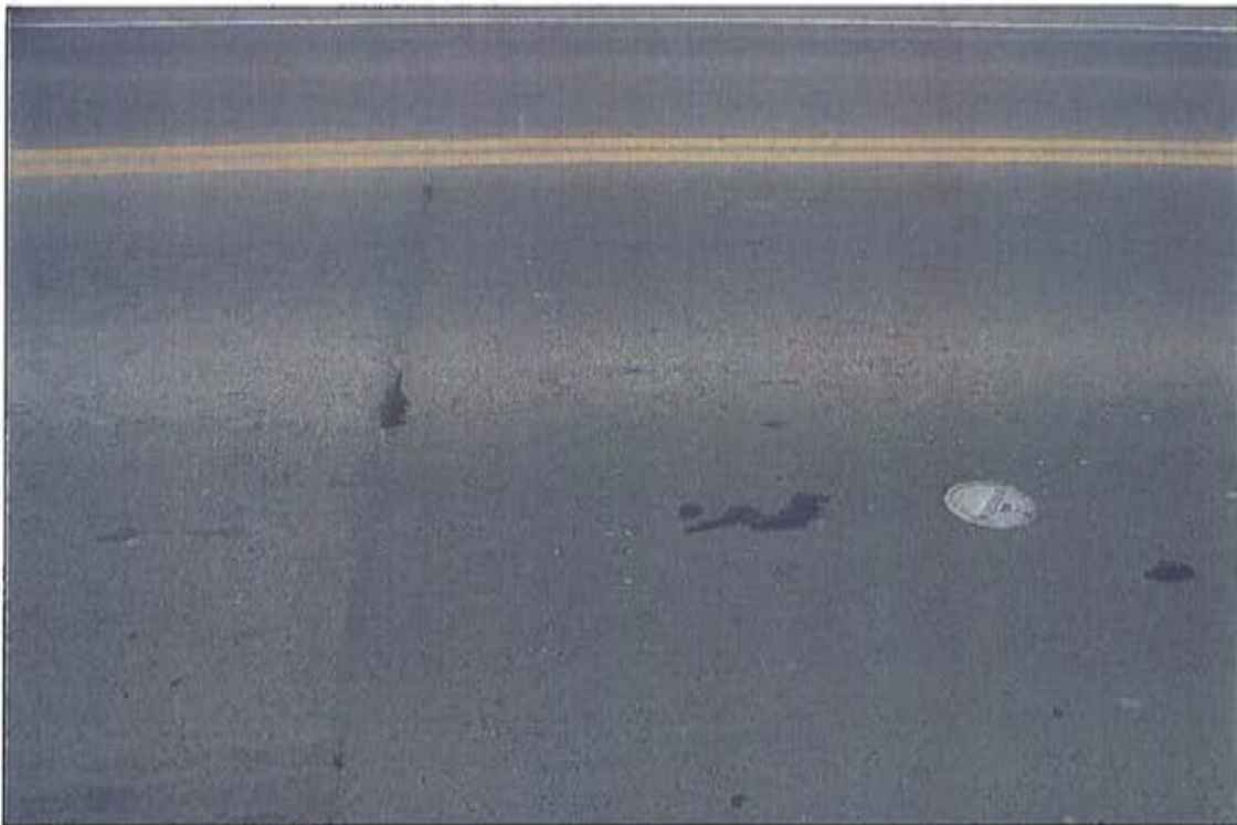
Photo 13: Wearing surface, east approach, looking north.
