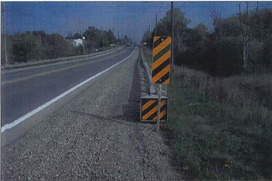
Photo 8: West approach, south side.
