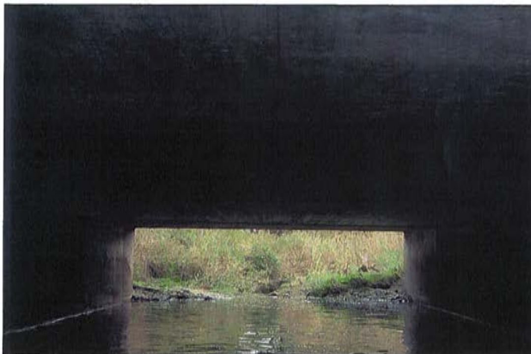
Photo 20: Culvert barrel, looking south.
