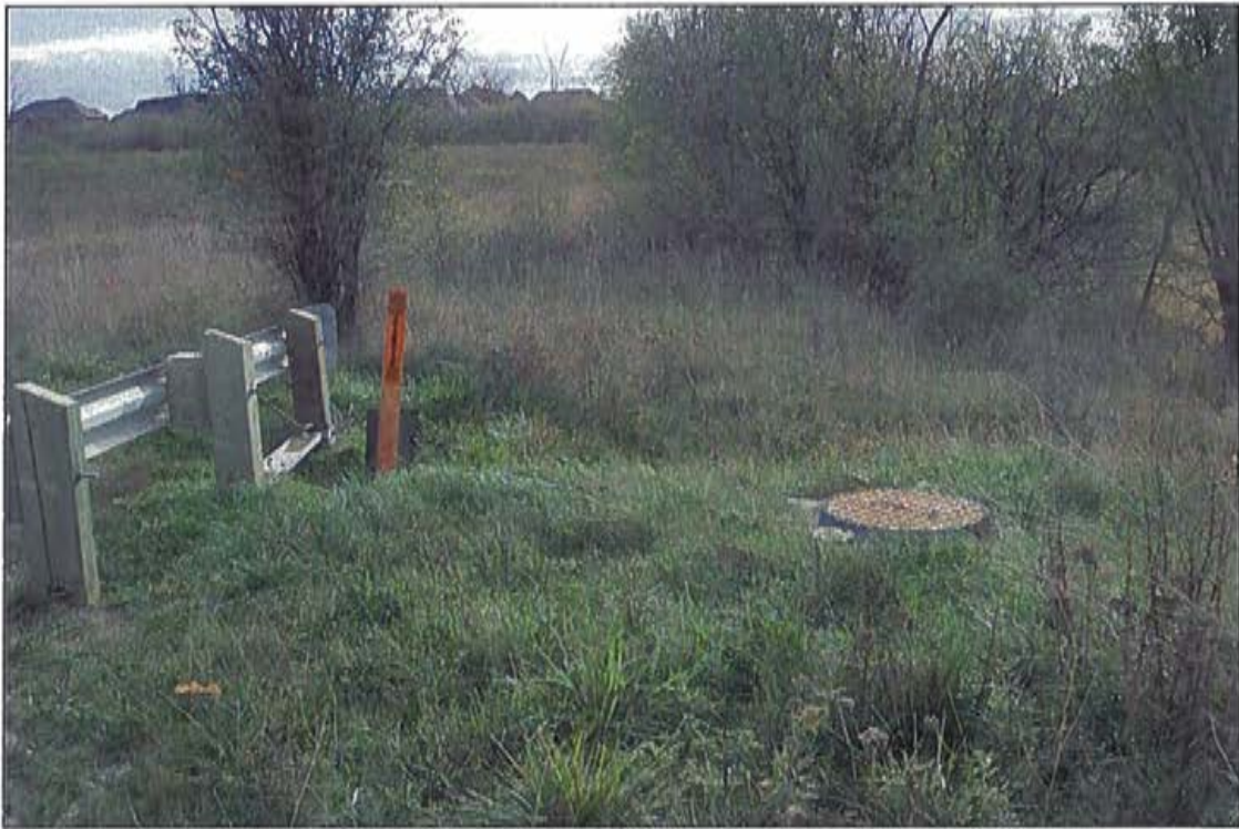
Photo 21: West approach, south side, Bell and water service.
