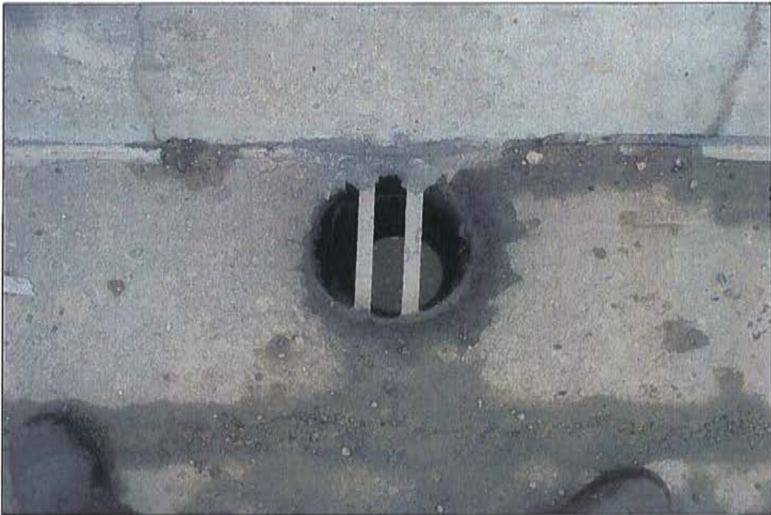
Photo 11: Deck drain (count 4).
