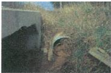
Existing Rigid Frame culvert at Sta. 15+156 (Crossing ID #12)
