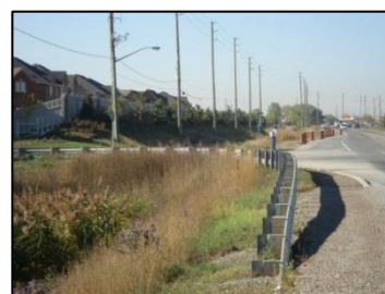
Existing Hydro One Brampton overhead hydro line.
