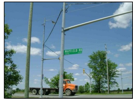
Mayfield Road Intersection
