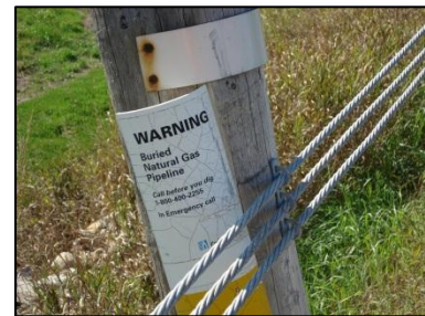
Underground Gas Line Marker at Mayfield Road
