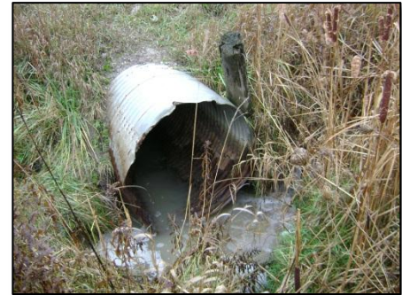
Mayfield Road CSP Culvert
