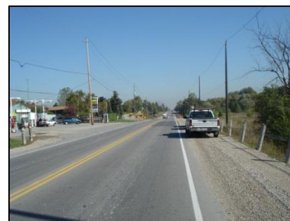
Existing Mayfield Road Section
