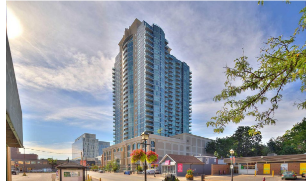
9 George Street North, Brampton
