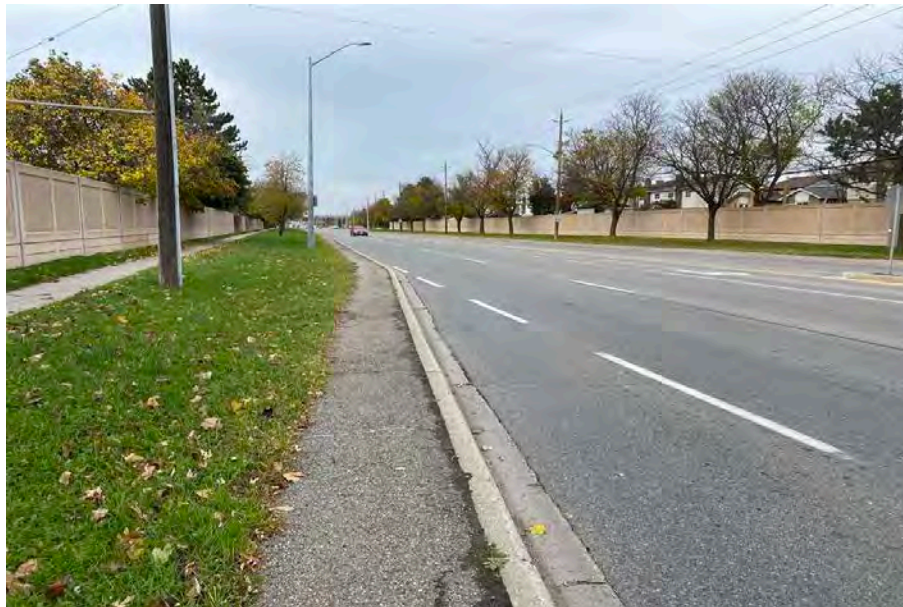
Image 53: LID area 17 showing disturbance, facing southeast
