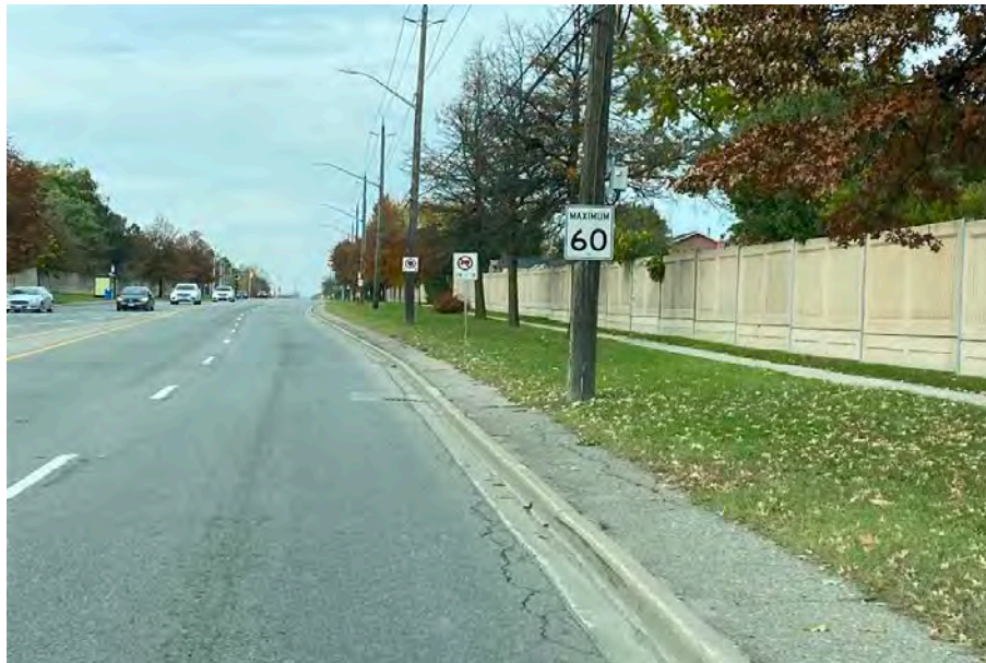
Image 55: LID area 17 showing disturbance, facing northwest
