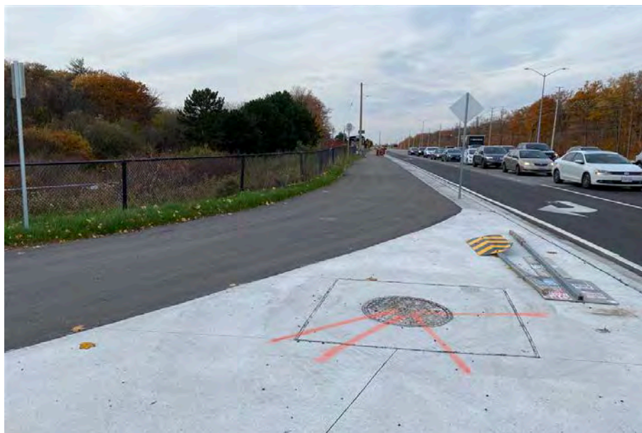
Image 20: LID area 11 showing paved disturbance, facing northwest
