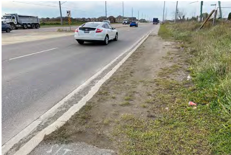
Image 13: LID area 5 showing disturbance along roadway, facing southwest
