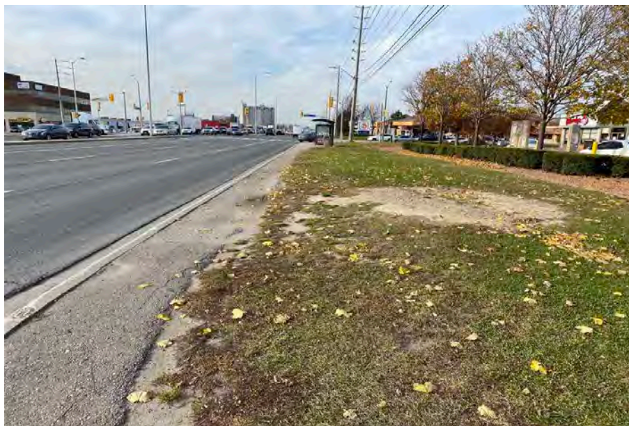
Image 36: LID area 13 showing disturbance, facing northwest
