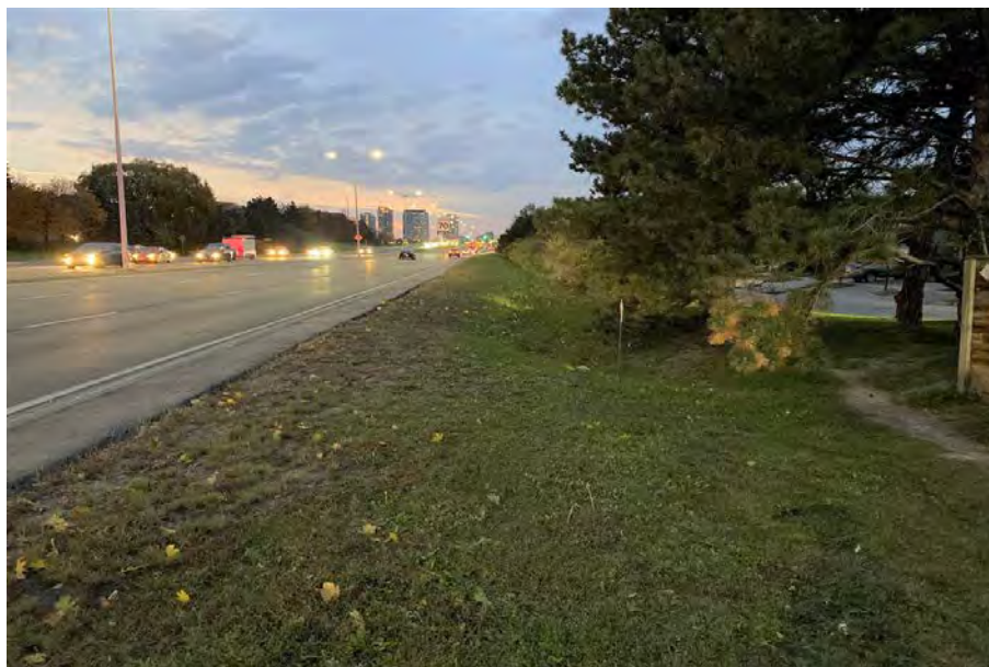
Image 46: LID area 16 showing slope, facing northwest
