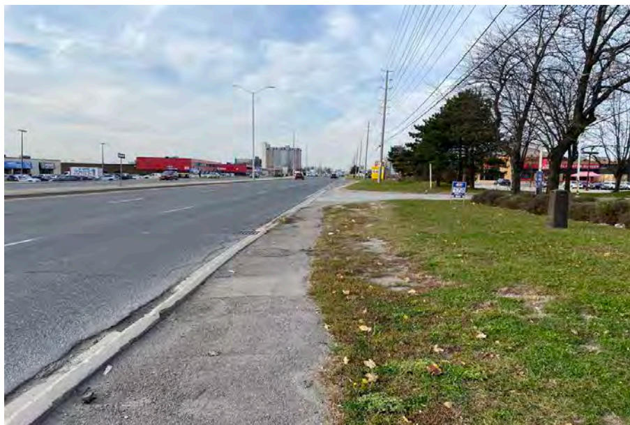
Image 38: LID area 13 showing disturbance, facing northwest
