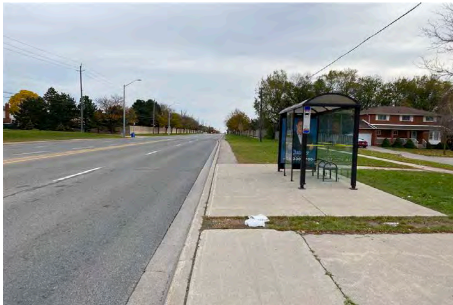
Image 52: LID area 17 showing disturbance, facing southeast
