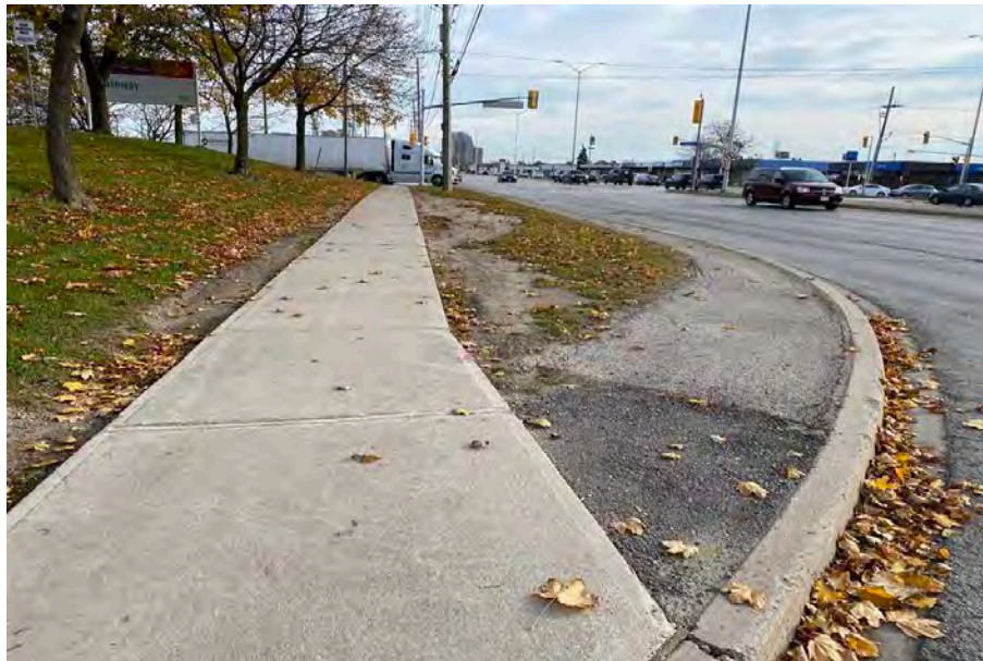
Image 31: LID area 13 showing paved disturbance, facing east
