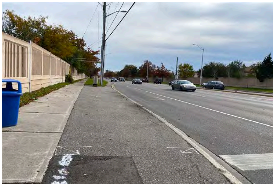
Image 54: LID area 17 showing disturbance, facing southeast
