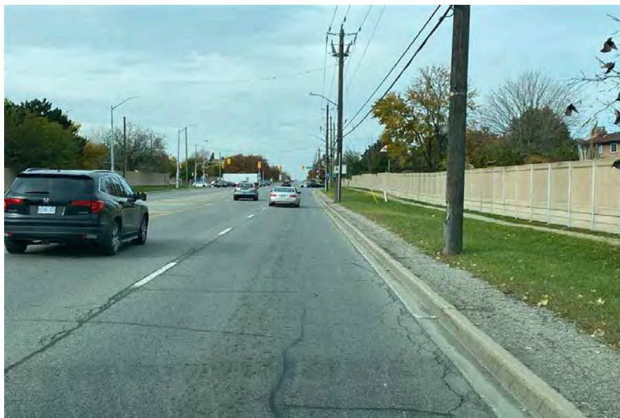
Image 56: LID area 17 showing disturbance, facing southeast
