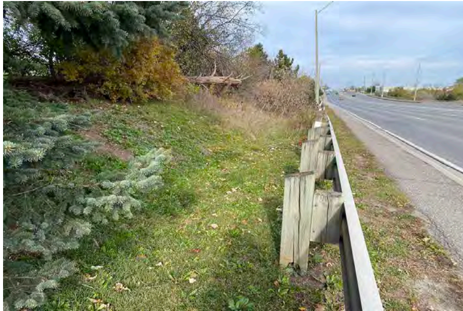
Image 7: LID area 2 showing built up and sloped area, facing east
