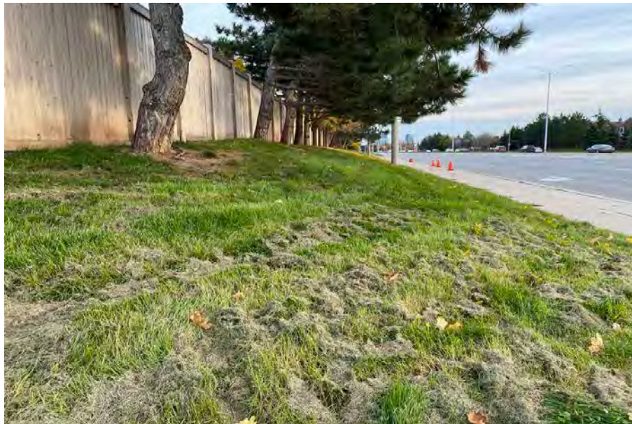
Image 25: LID area 11 showing slope, facing southeast
