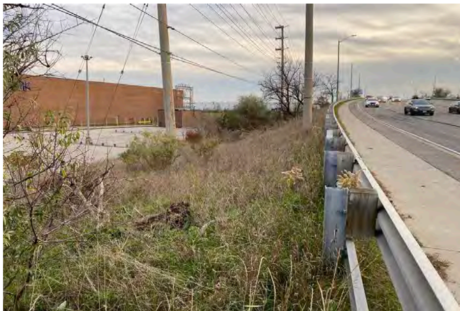
Image 6: LID area 1 showing slope down to parking lot, facing south
