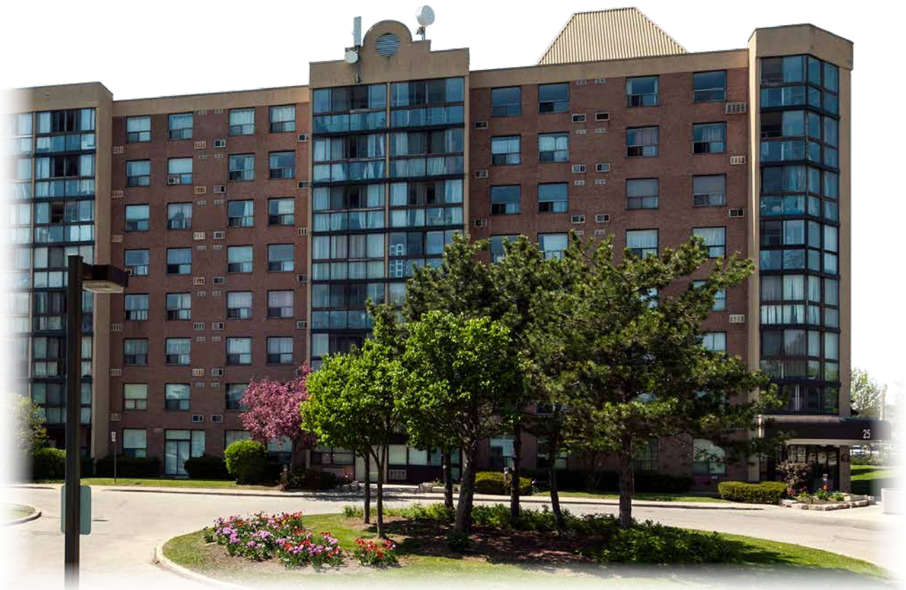
The Region of Peel's affordable housing community on Glenn Hawthorne Blvd., Mississauga
