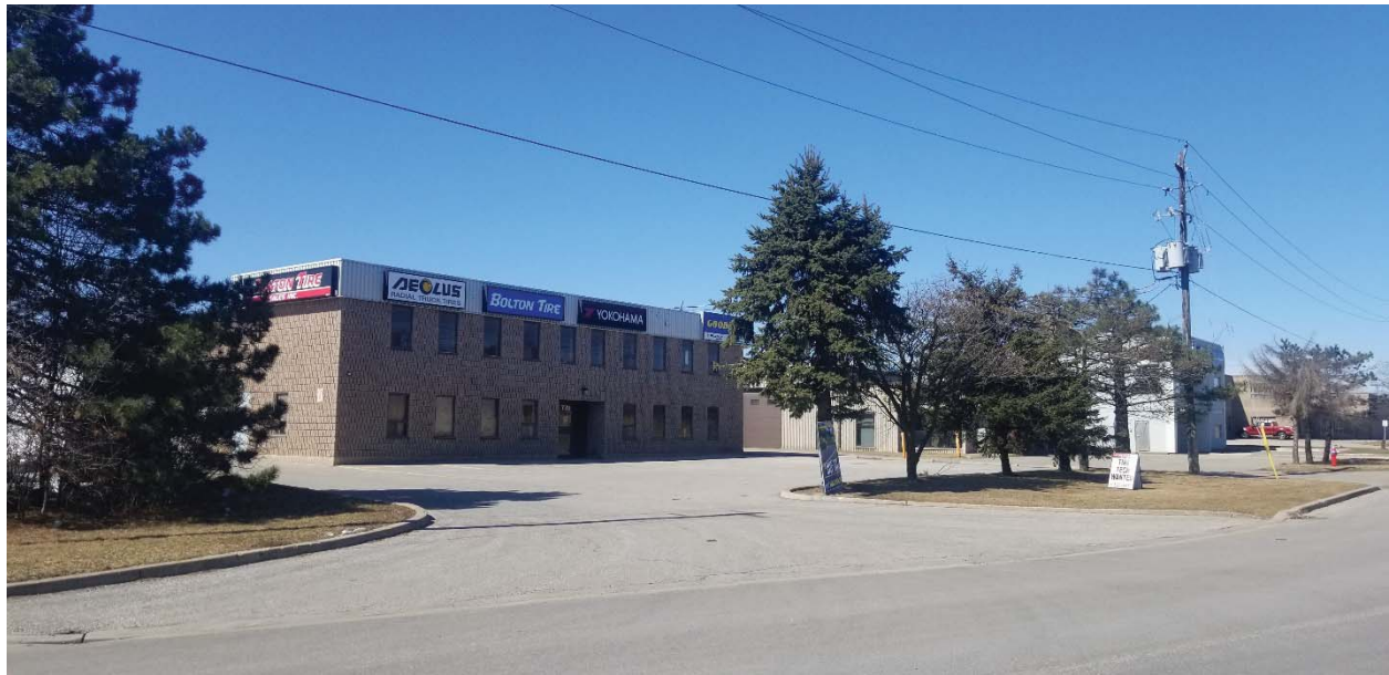
Photo 4: Bolton Tire Sales Inc auto service garage located at 770 Hardwick Road. Pole mounted hydro transformers are visible in the photo.
