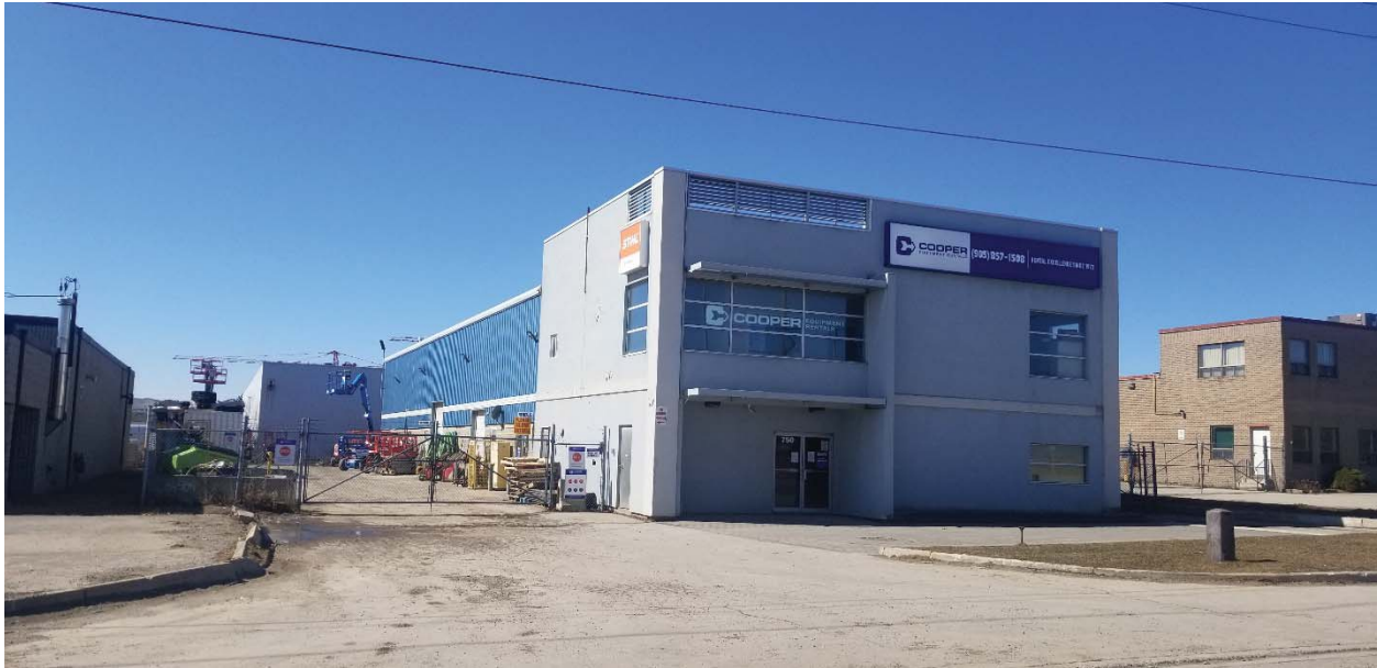
Photo 7: Cooper rental located at 750 Hardwick Road. Machinery, generators, compressors and fuel receptor storage cabinets were observed outside of the building.
