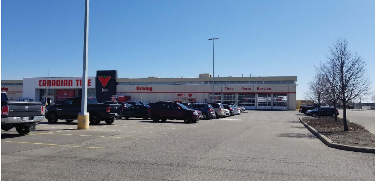
Photo 19: A Canadian Tire store with associated automotive garage was observed at 99 McEwan Drive. A large green pad transformer was observed in the south west quadrant of the property. A fenced enclosure was observed to the west of the automotive center with visible 205 L drums and oil containers being stored.
