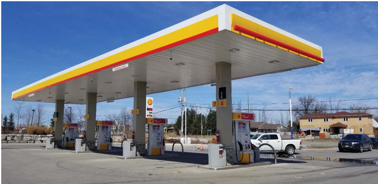
Photo 34: A Shell Gas Station was located at 12182 Highway 50. Several fuel storage tanks were reported for the property. The gas station is located adjacent to the Site.
