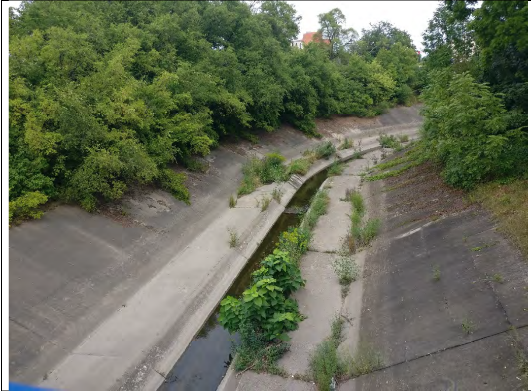
Photo 11. Concrete channel and bench, looking south from Scott St.
