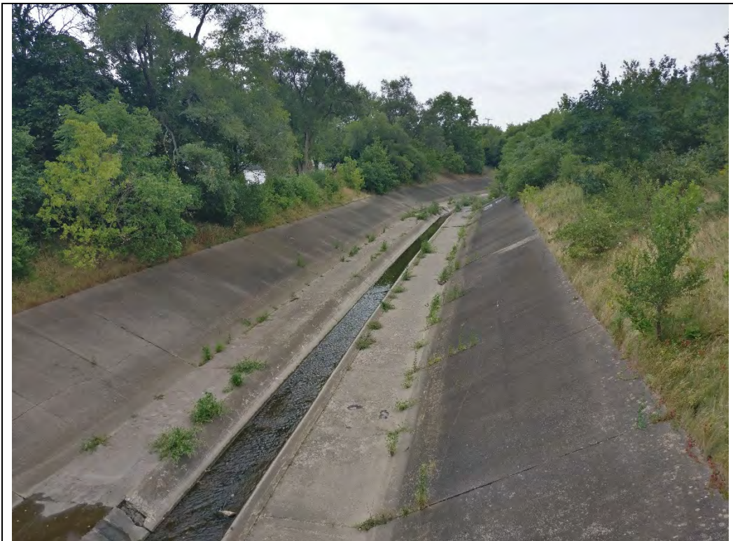
Photo 12. Concrete channel and bench, looking south from Queen St.
