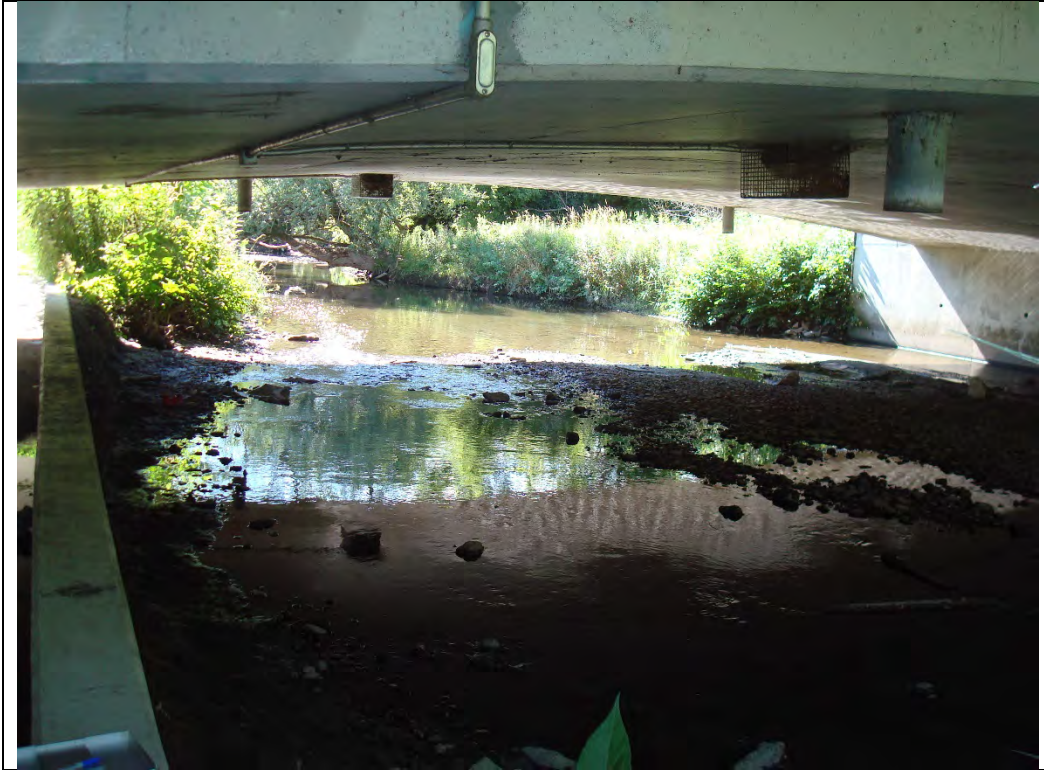
Photo 5. Beneath Vodden St. E bridge, looking south.
