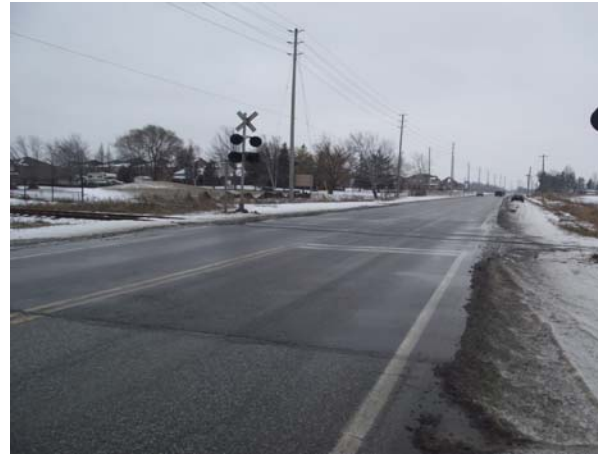
Figure 4-11 - Asphalt in good condition leading up to railway crossing
