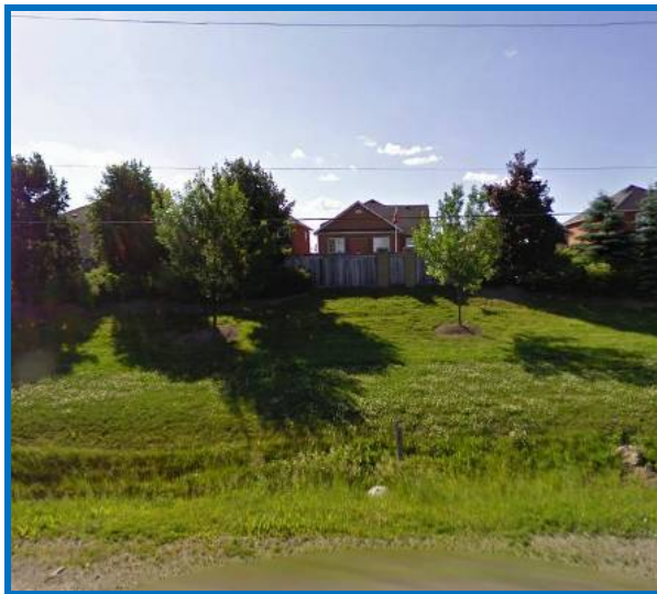
Figure 6-18 - Wooden fence constructed on an elevated slope, viewed from Mayfield Road
