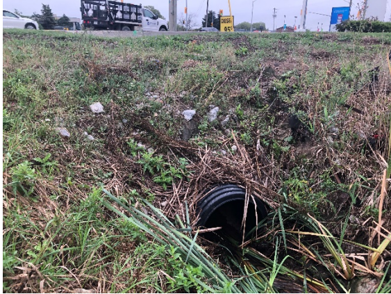
FIGURE 1 Culvert 1 Upstream End
