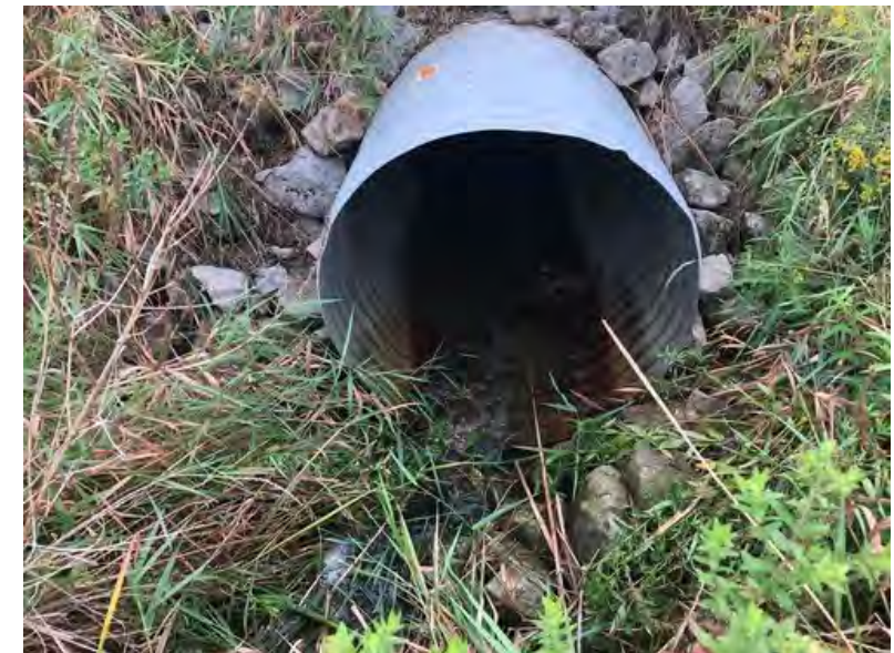
12. Culvert C1a (Inlet)
