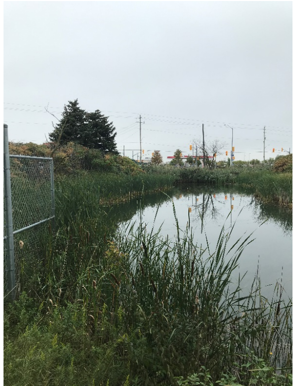
FIGURE 18 Existing Pond Looking Upstream
