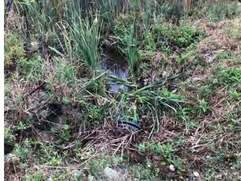
8. Culvert C1 (Inlet)
