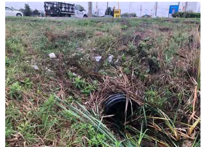
6. Culvert C1 (Inlet)
