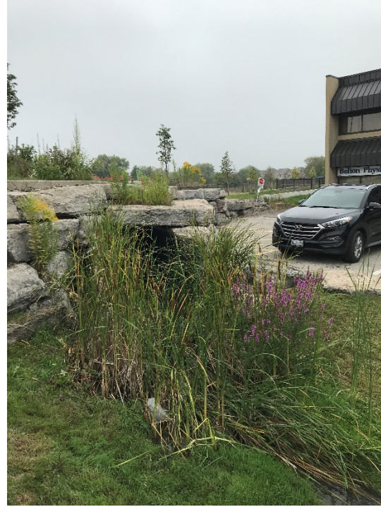
FIGURE 8 Culvert 3 Downstream End
