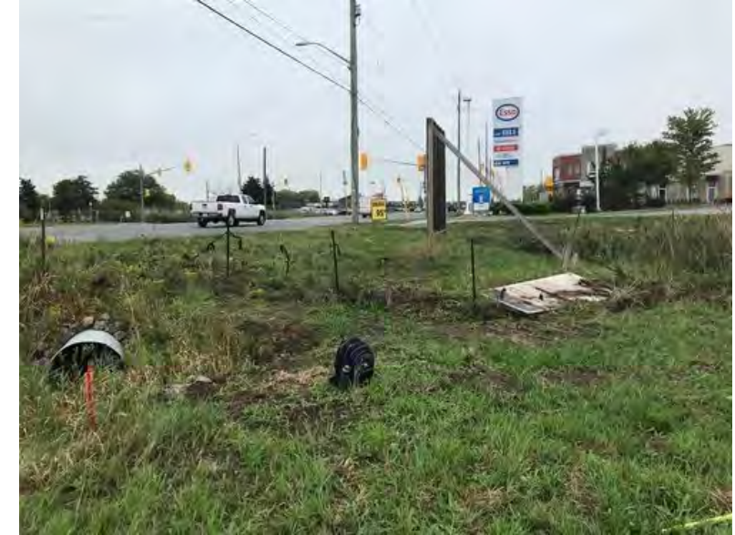
9. Culvert C1a (Inlet)
