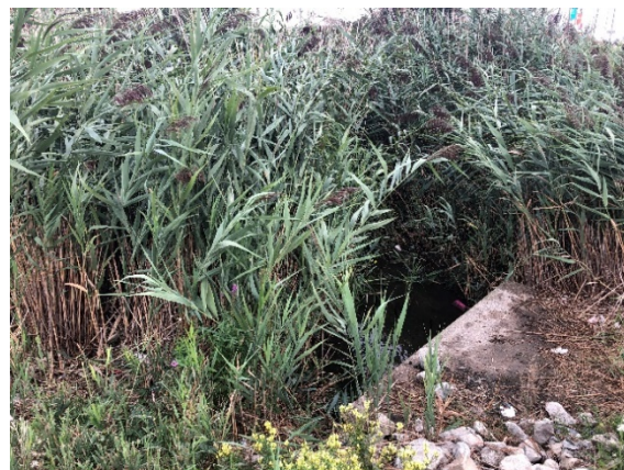
FIGURE 4 Culvert 1 Downstream End
