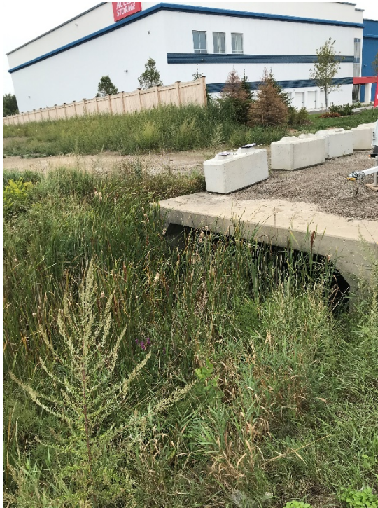
FIGURE 14 Culvert 7 Upstream End
