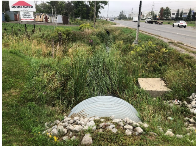
FIGURE 12 Culvert 5 Looking Downstream
