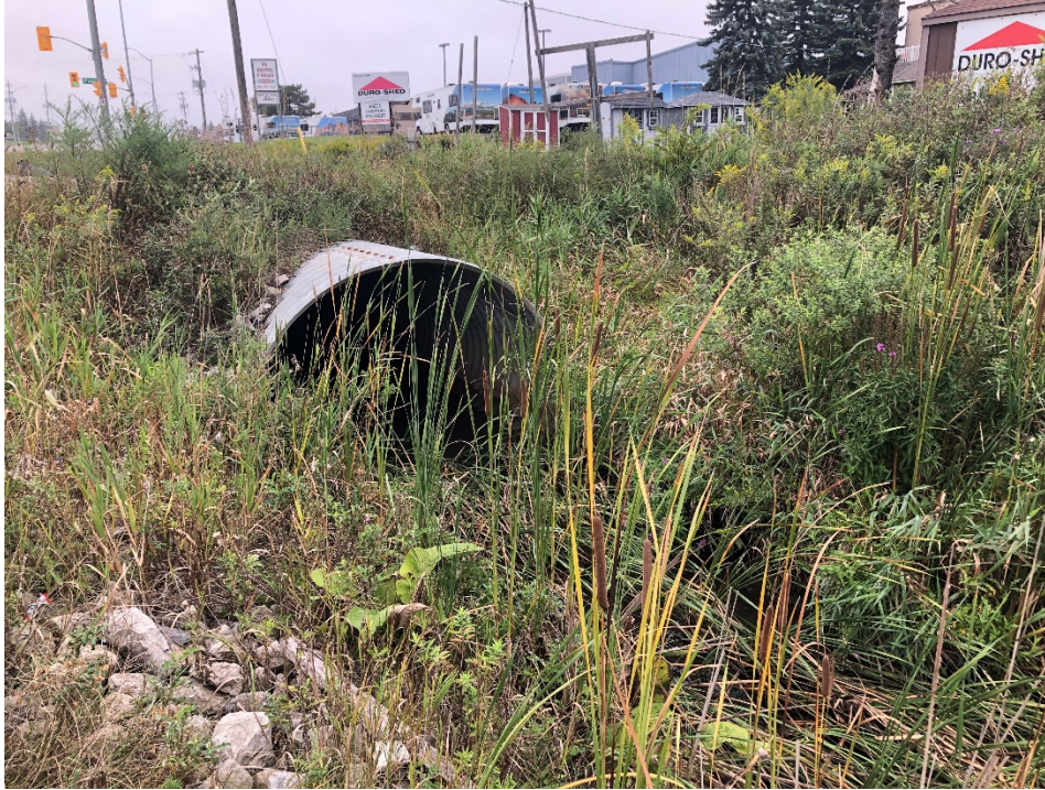
FIGURE 13 Culvert 6 Downstream End
