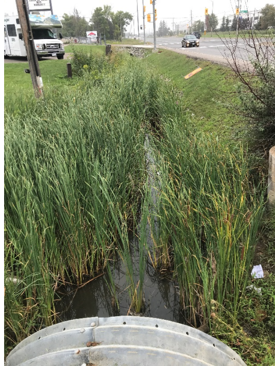
FIGURE 10 Culvert 4 Looking Downstream
