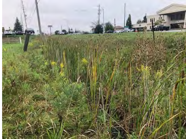
13. Culvert C1a (Inlet)
