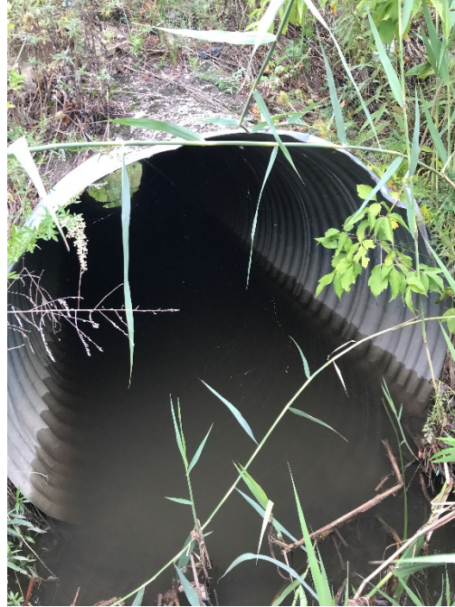
FIGURE 6 Culvert 2 Downstream End
