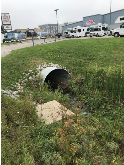
FIGURE 11 Culvert 5 Downstream End
