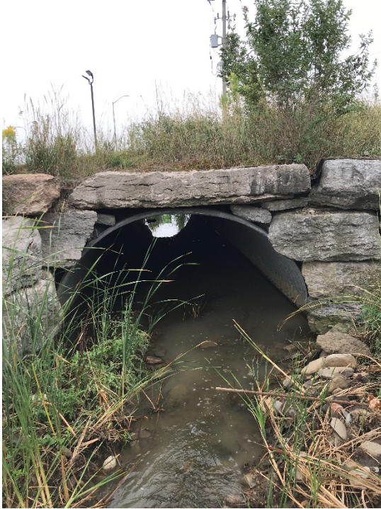
FIGURE 7 Culvert 3 Upstream End
