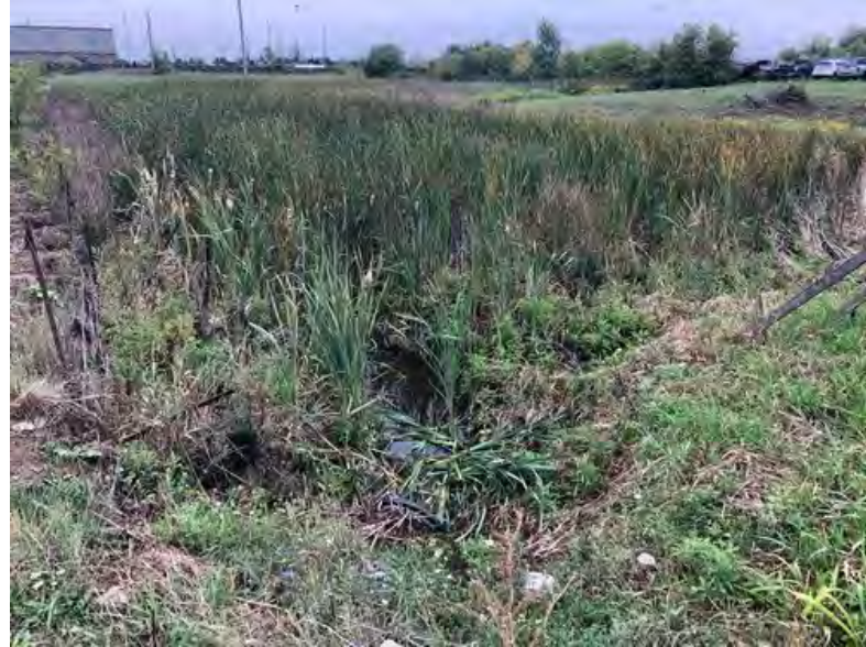
7. Culvert C1 (Inlet)
