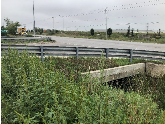
FIGURE 16 Culvert 8 Upstream End
