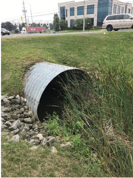
FIGURE 9 Culvert 4 Upstream End
