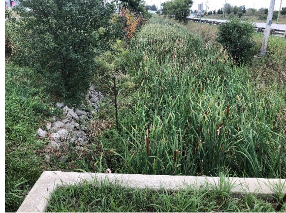
FIGURE 17 Culvert 8 Looking Downstream
