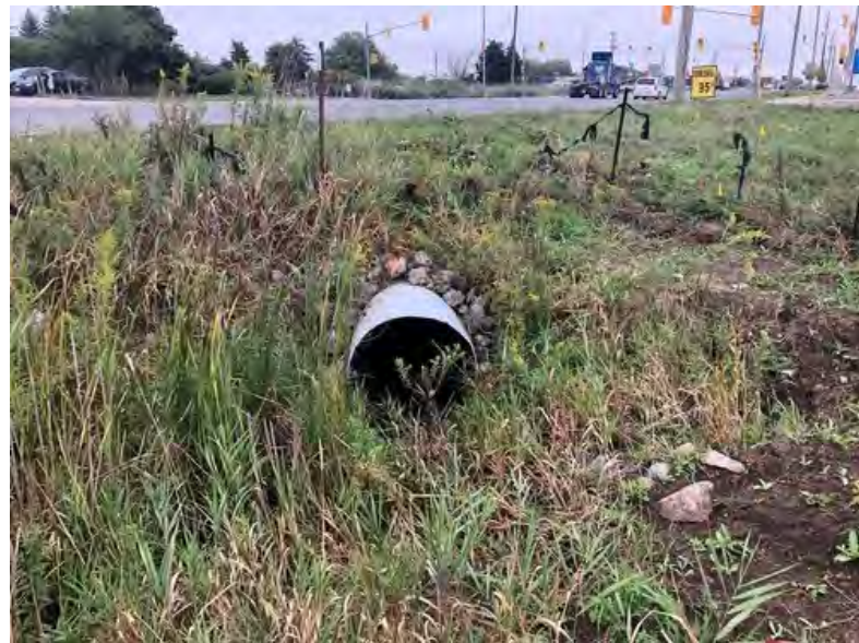
10. Culvert C1a (Inlet)
