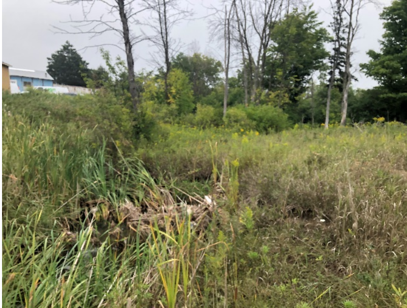
FIGURE 21 Looking Downstream from Culvert 6 (Subject Property on Right)
