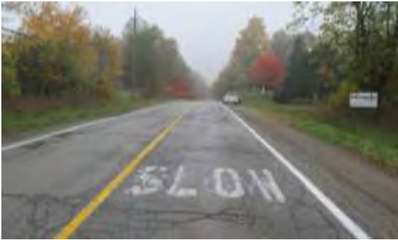
Figure 17: 'SLOW' Pavement Marking Painted on Previously Faded Marking
