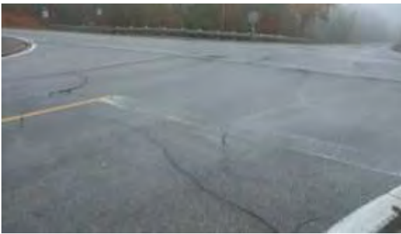
Figure 15: Faded Stop Bar Pavement Marking at Intersection of Mississauga Road and Olde Base Line Road
