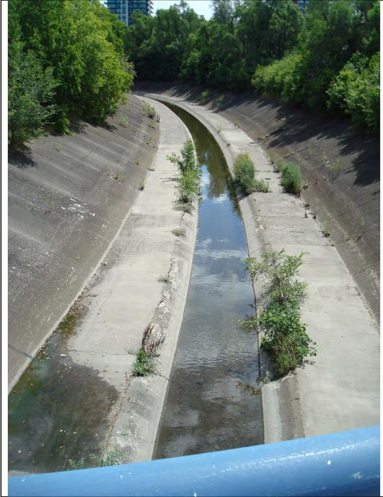
*Photo 10. Concrete channel and bench, looking south from Church St.*
