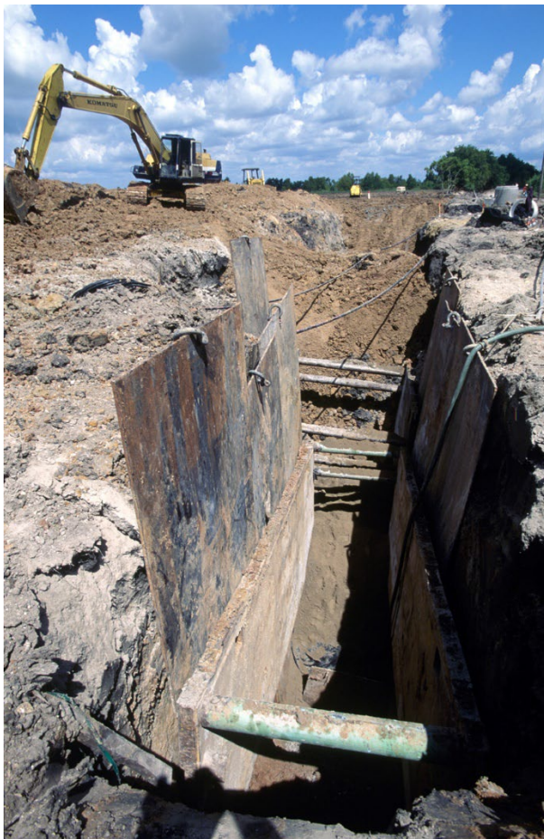
Figure 7-2. Open-Cut Construction
