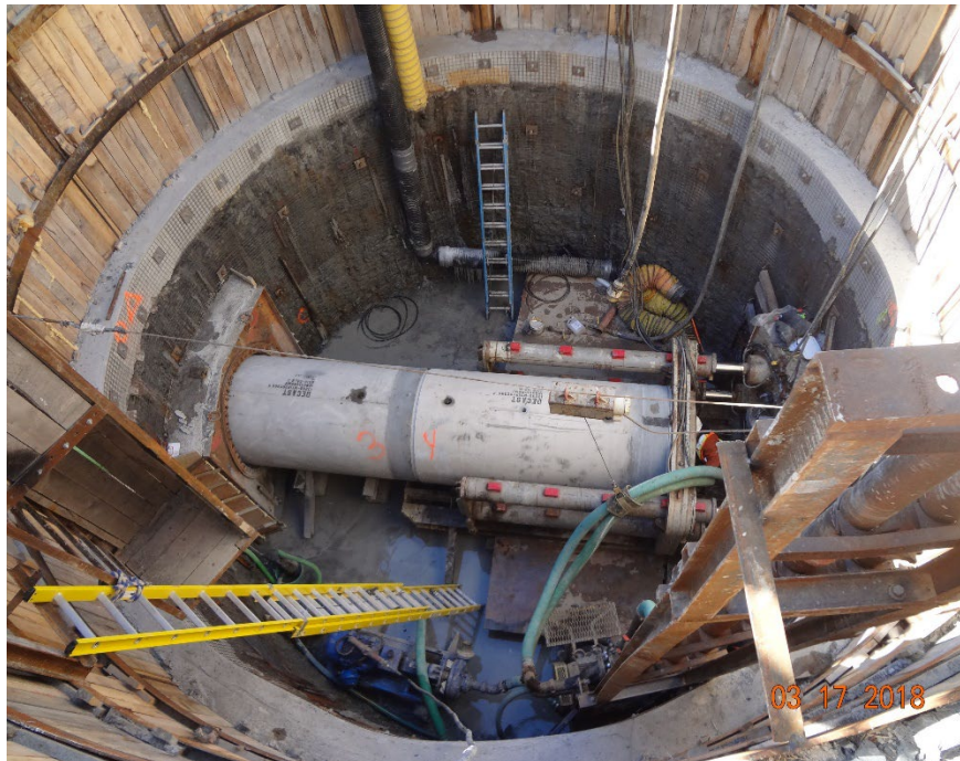
Figure 7-3. Launching Shaft Example
