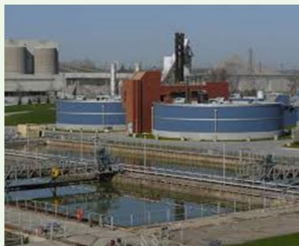
Anaerobic Digestion and Dewatering (Clarkson Wastewater Treatment Plant)
