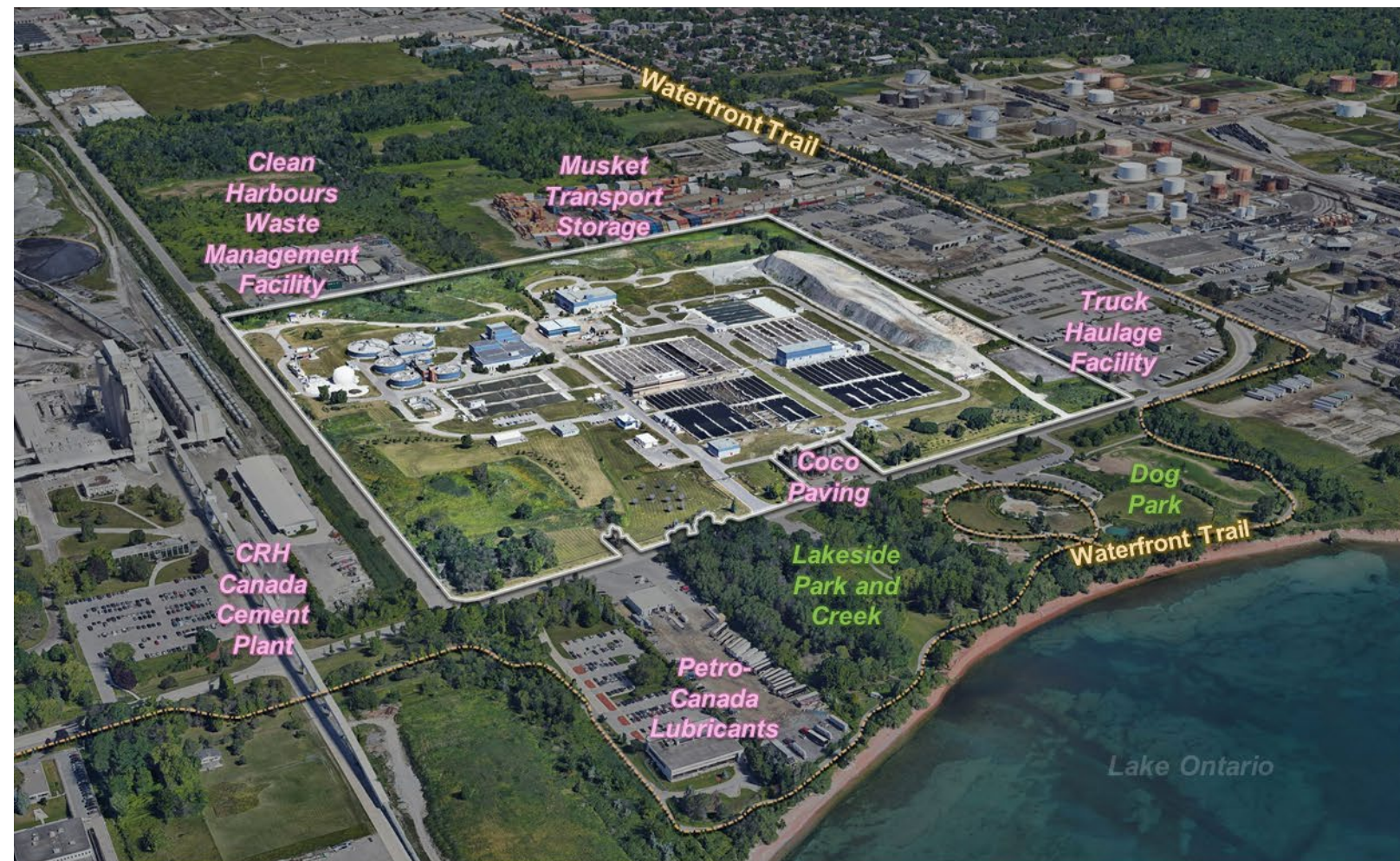
Clarkson Wastewater Treatment Plant
