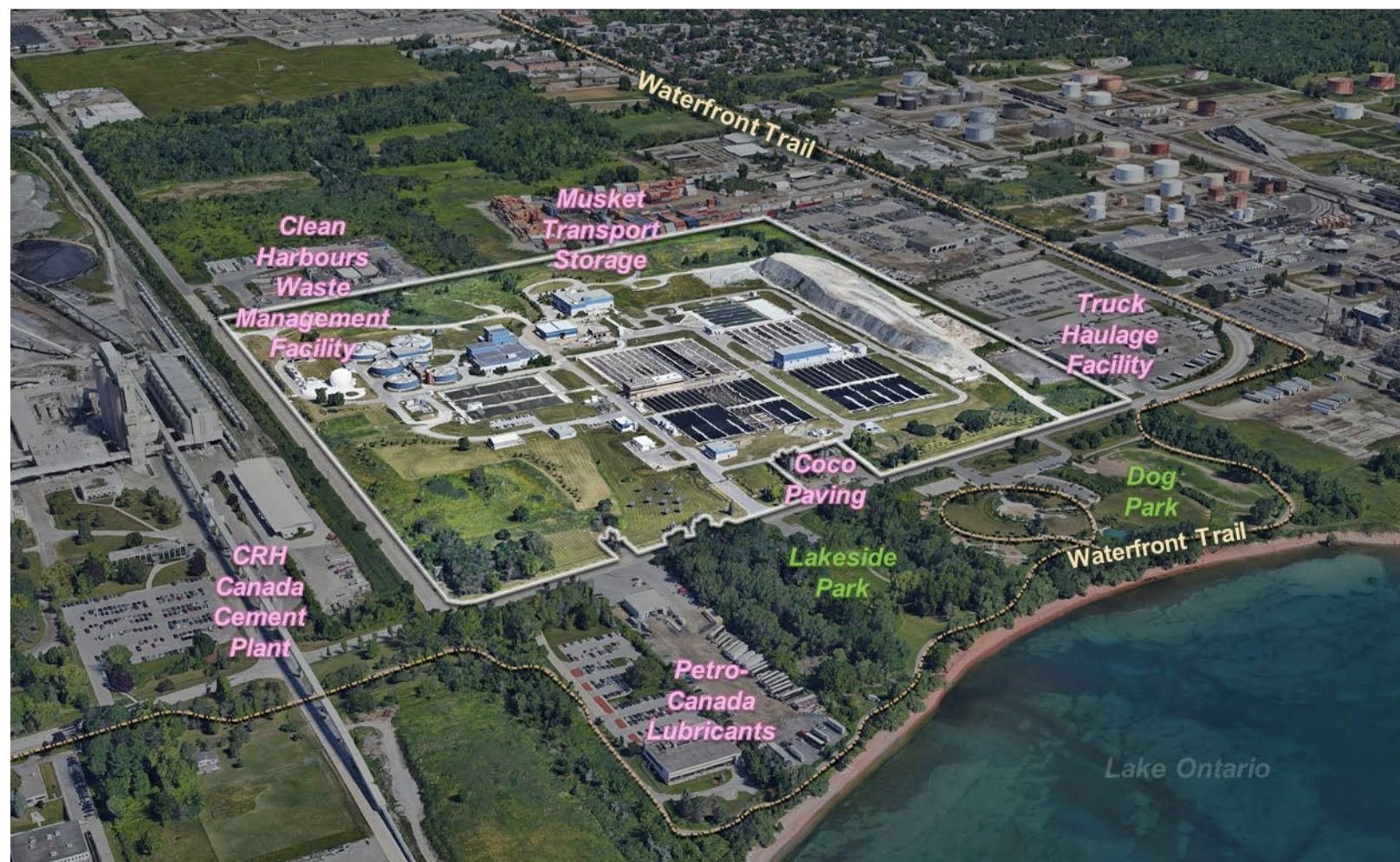
Clarkson Wastewater Treatment Plant
