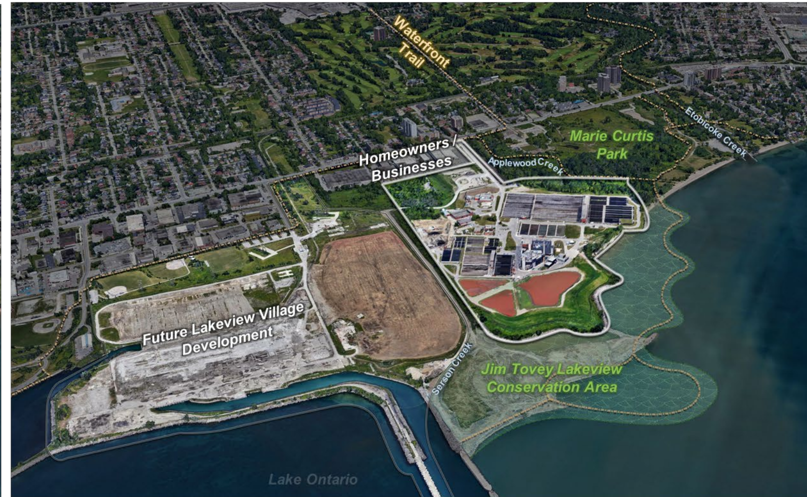
G.E. Booth Wastewater Treatment Plant
