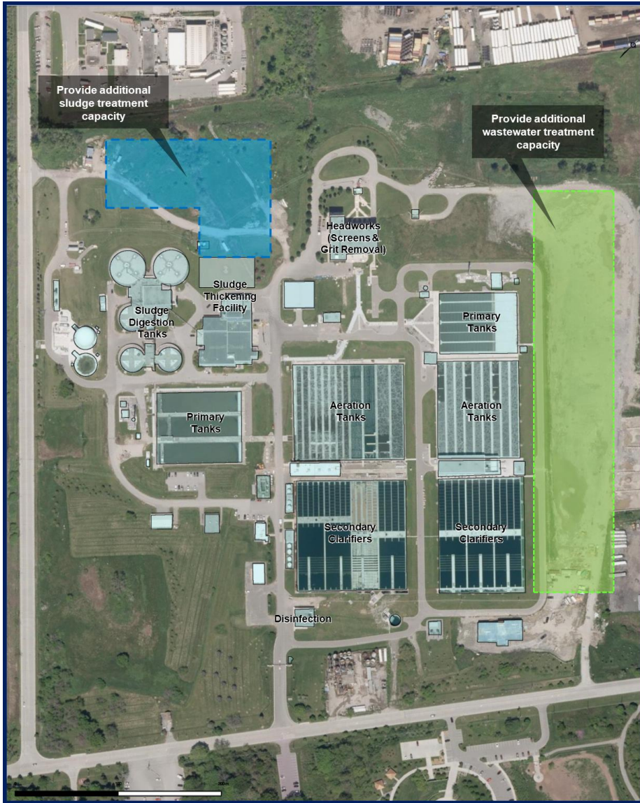
Clarkson Wastewater Treatment
