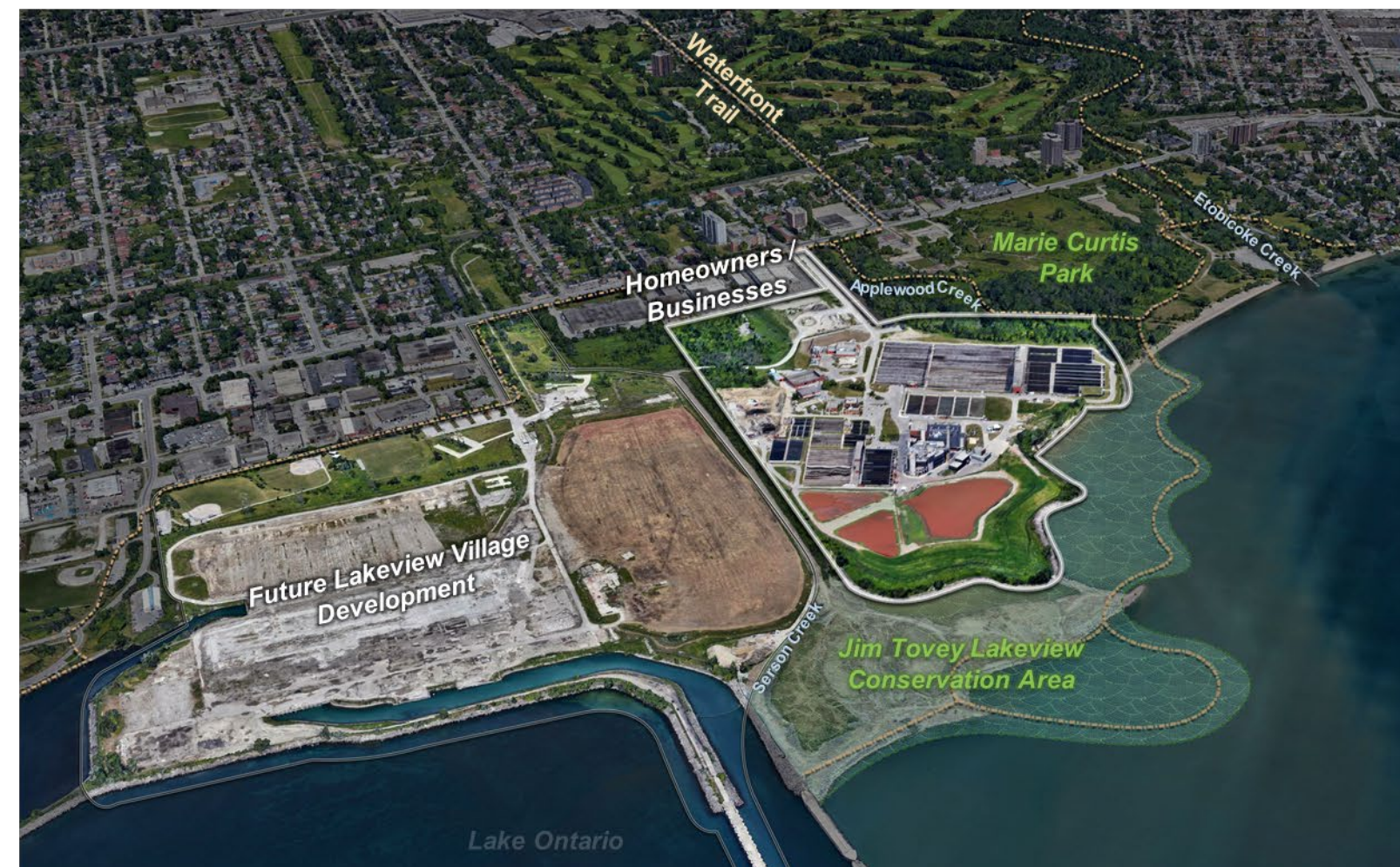
G.E. Booth Wastewater Treatment Plant
