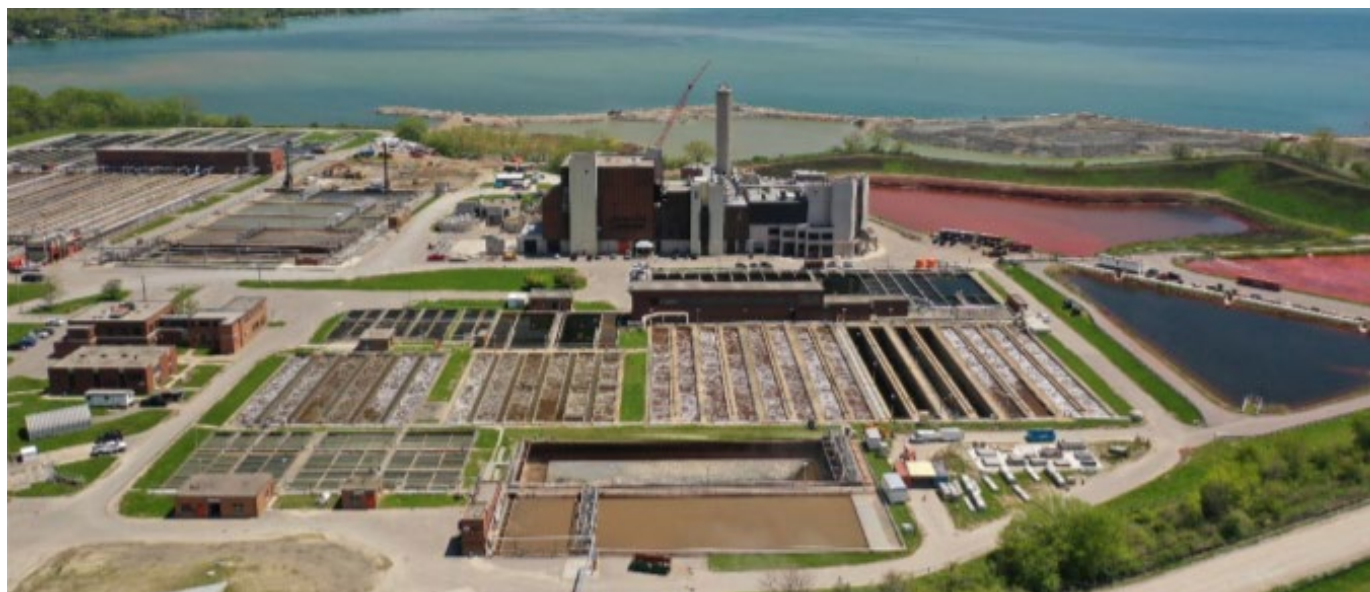
G.E. Booth Wastewater Treatment Plant
