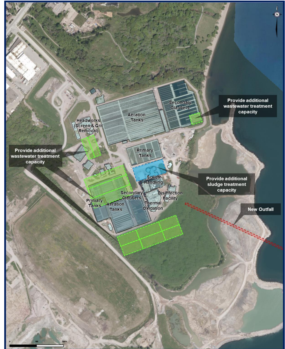
G.E. Booth Wastewater Treatment
