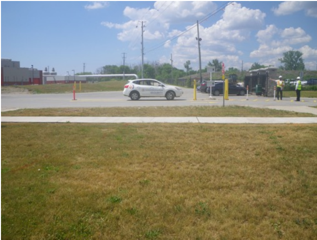
Image 29: View of heaving graded landscape, paved areas and extant buildings and installations around the entrance to G.E. Booth WWTP.
