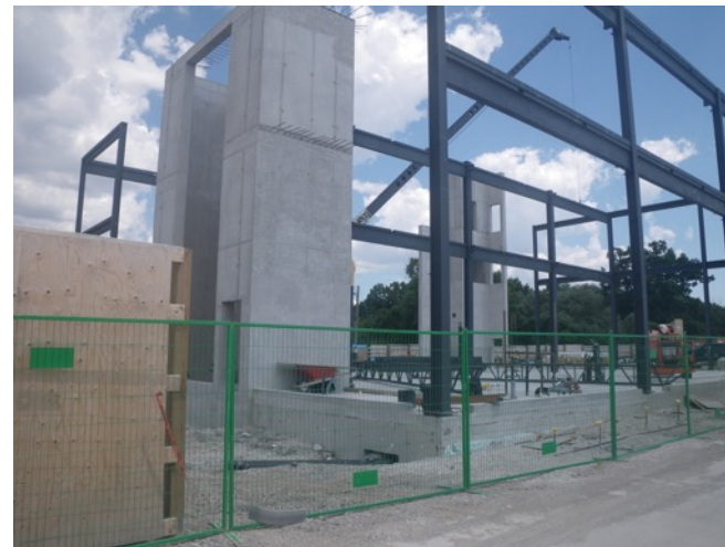
Image 28: View of storage complex under construction at G.E. Booth WWTP.
