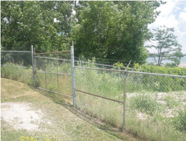
Image 25: View of exposed graded soils forming artificial tableland just above mouth of Applewood Creek, within G.E. Booth WWTP.
