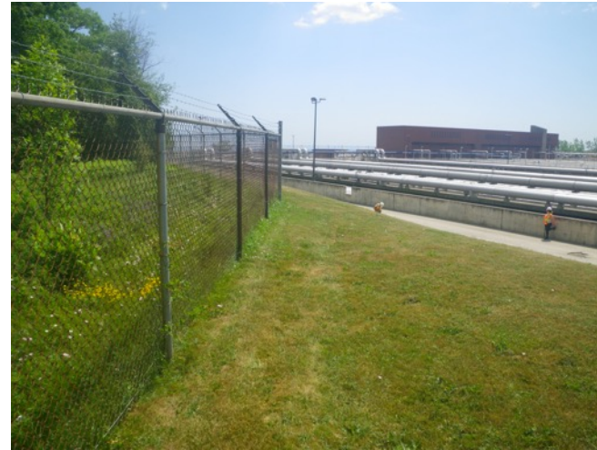
Image 26: View of graded margins and extant structures at G.E. Booth WWTP.
