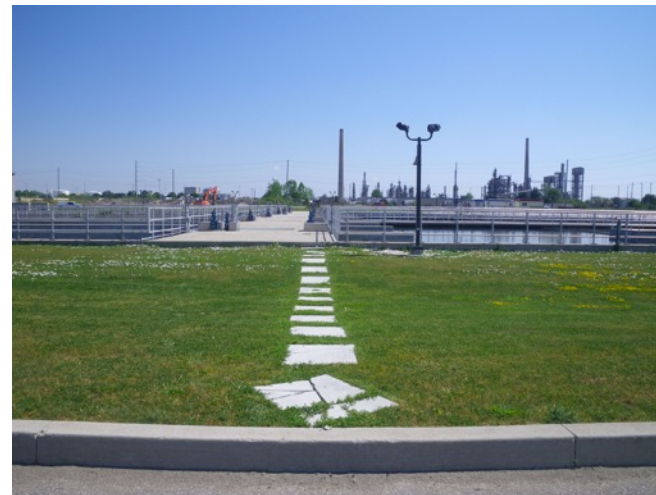
Image 8: View of extant structures and disturbed landscape at Clarkson WWTP.
