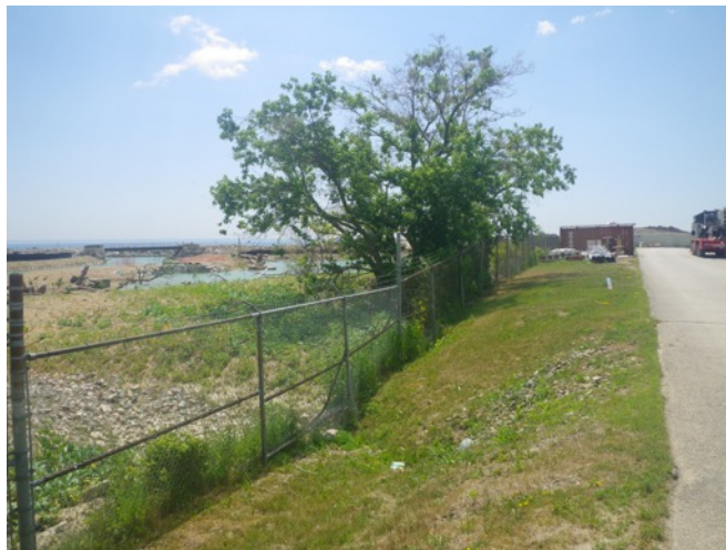
Image 24: View of extant paved road and artificial landscape at G.E. Booth WWTP, with ongoing Lake Ontario reclamation works visible.
