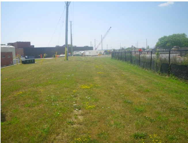
Image 31: View of graded landscape and extant buildings and installations in northwest of G.E. Booth WWTP.
